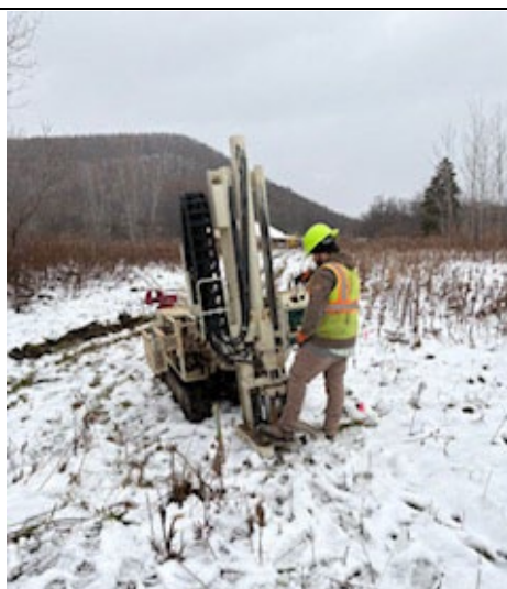
PZ-1 Geoprobe Installation (located between TP-1 and TP-3)
