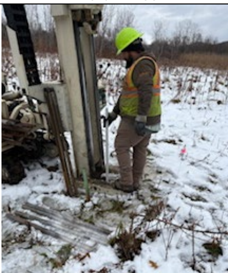
PZ-1 Geoprobe Installation
