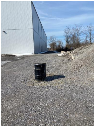
Looking along the North Side of Facility
