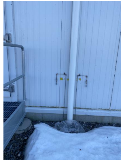
North Side Exterior Air Vents
