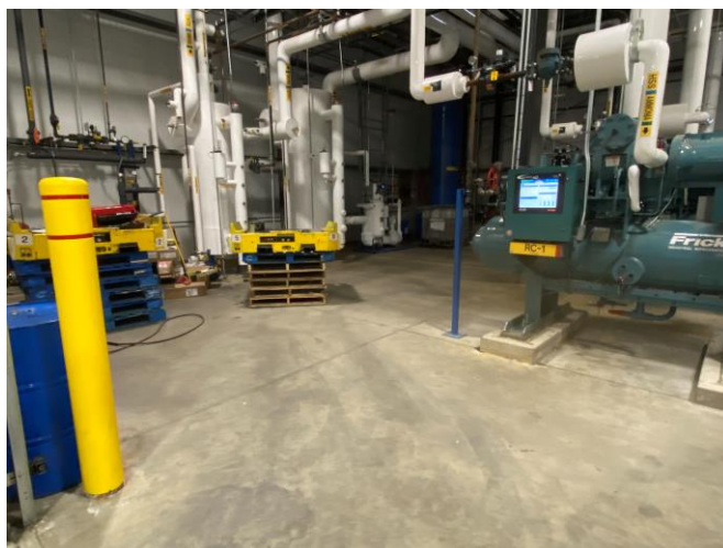
Maintenance area of New Warehouse
