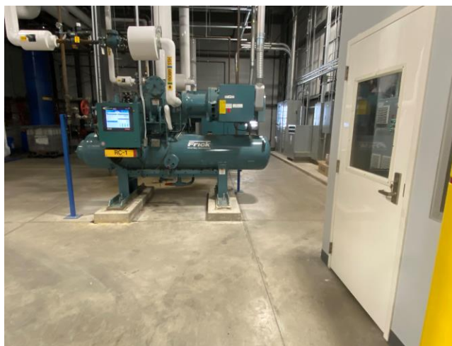
Maintenance area of New Warehouse
