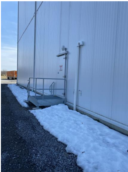
North side Exterior Air Vents
