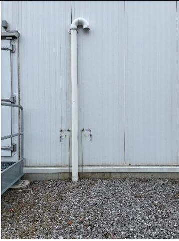
View of typical passive SSDS exhaust pipe
