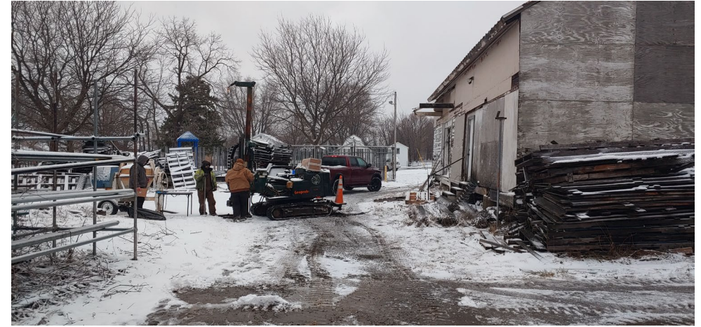
BH4 Location (Facing East)
