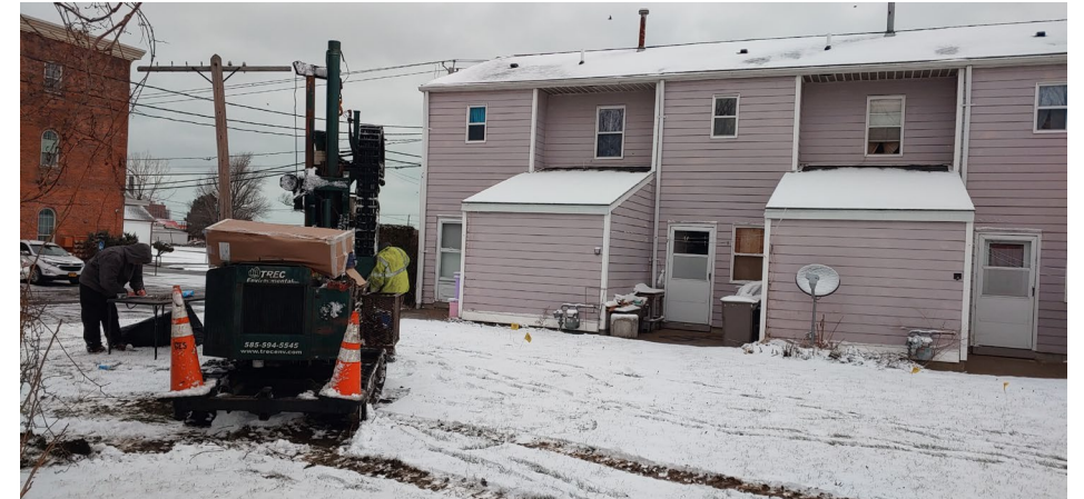
BH16 Location. (Facing North)
