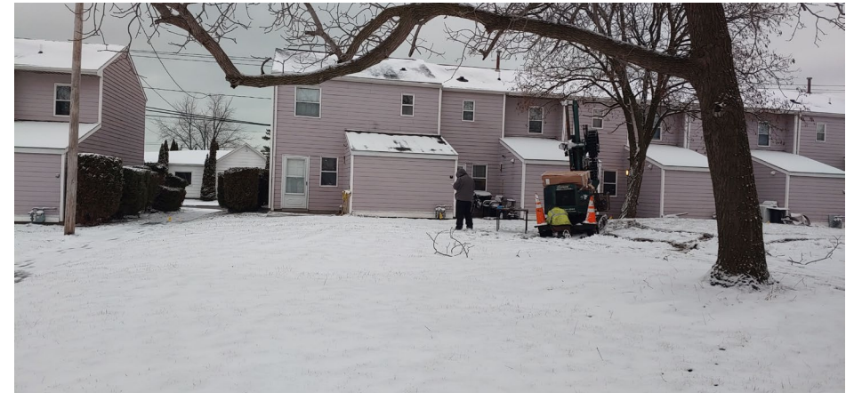
BH13 Location. (Facing North)
