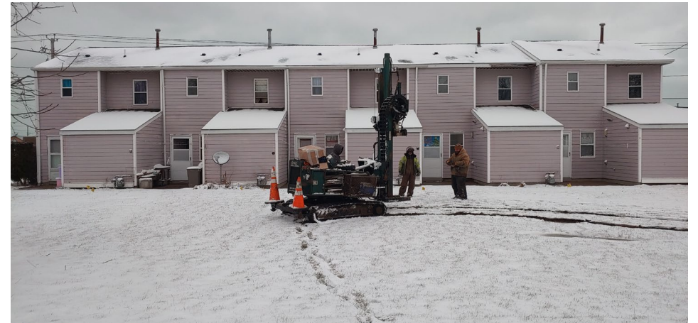
BH15 Location. (Facing North)
