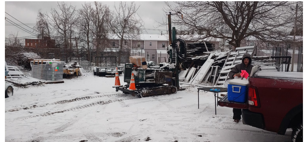
BH5 Location (Facing North)
