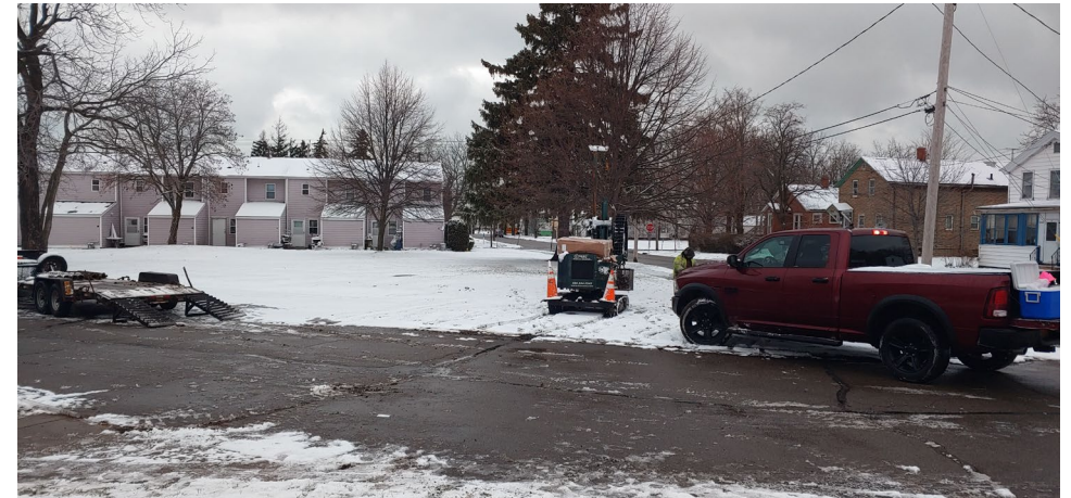
BH9 Location. (Facing North)
