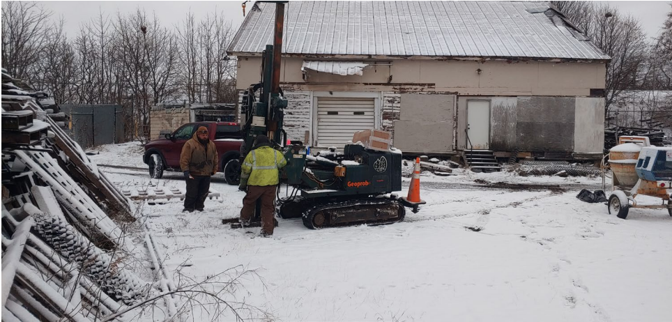
BH5 Location. (Facing South)
