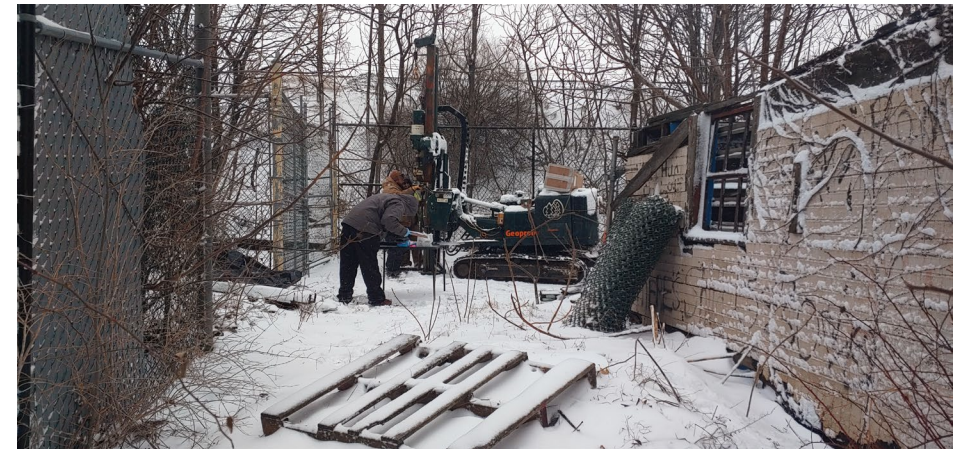
BH2 Location (Facing South)
