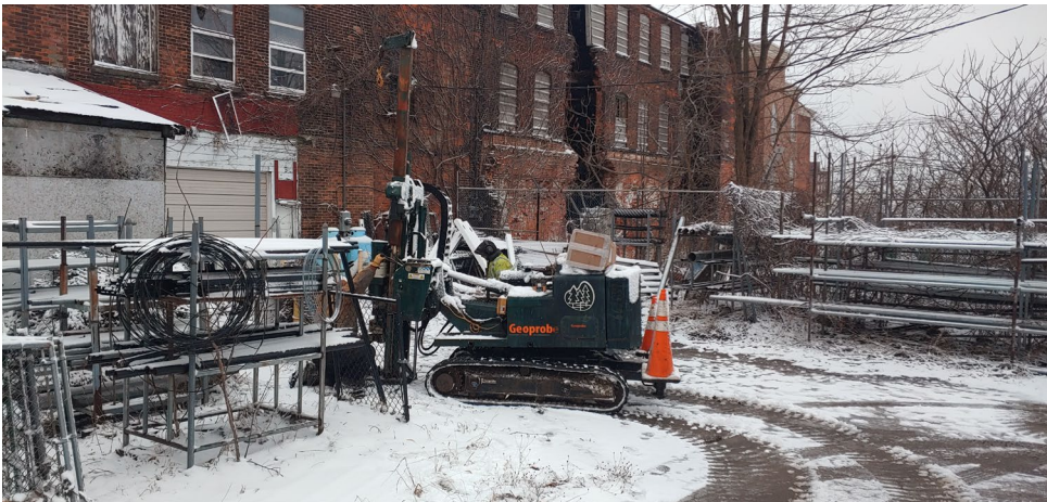
BH3 Location. (Facing Northwest)
