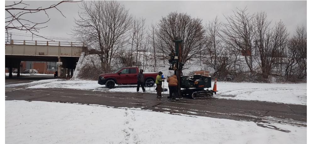
BH8 Location. (Facing South)
