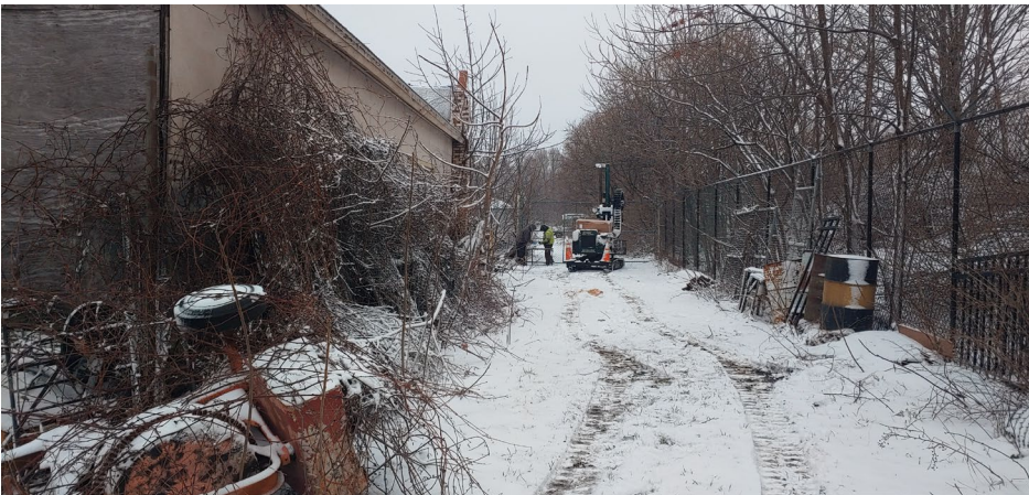
BH2 Location (Facing East)
