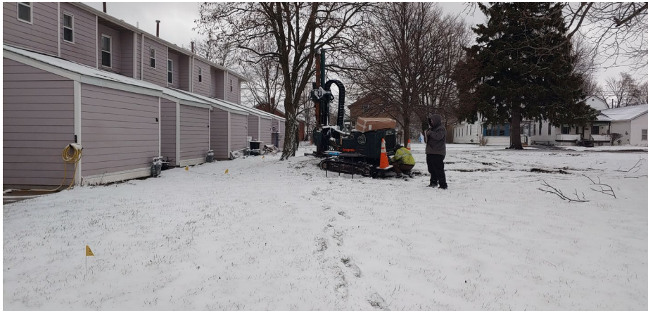
BH13 Location. (Facing East)
