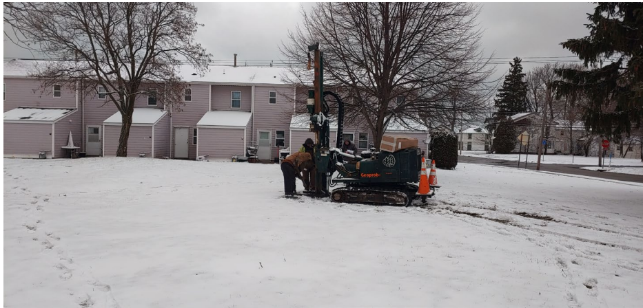
BH11 Location (Facing North)
