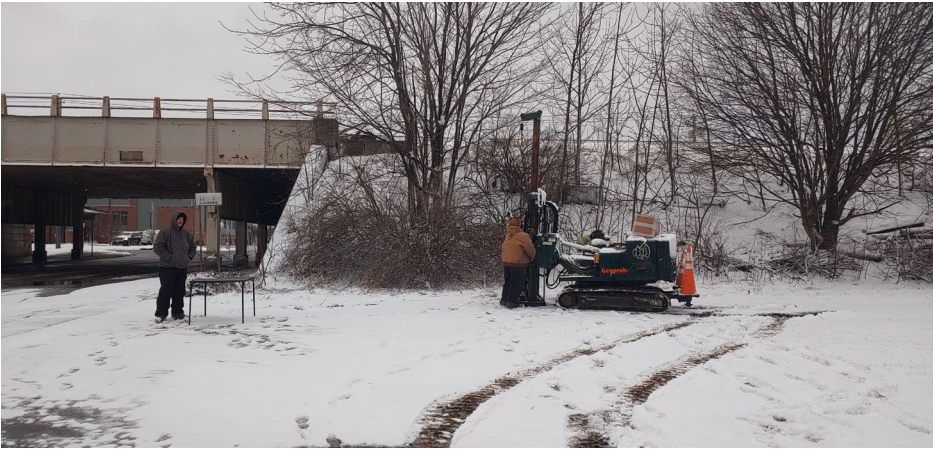
BH1 Location. (Facing South)
