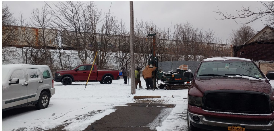
BH7 Location. (Facing Southwest)
