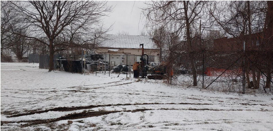
BH17 Location. (Facing South)
