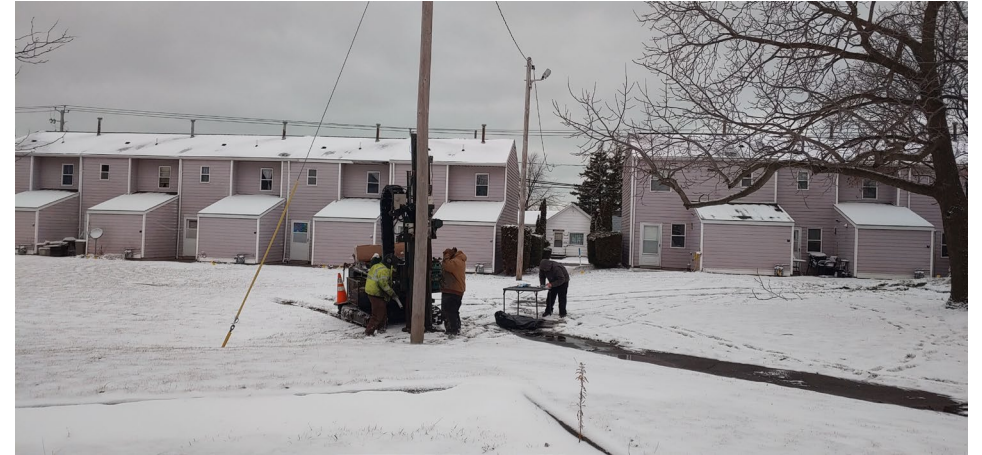
BH14 Location. (Facing North)
