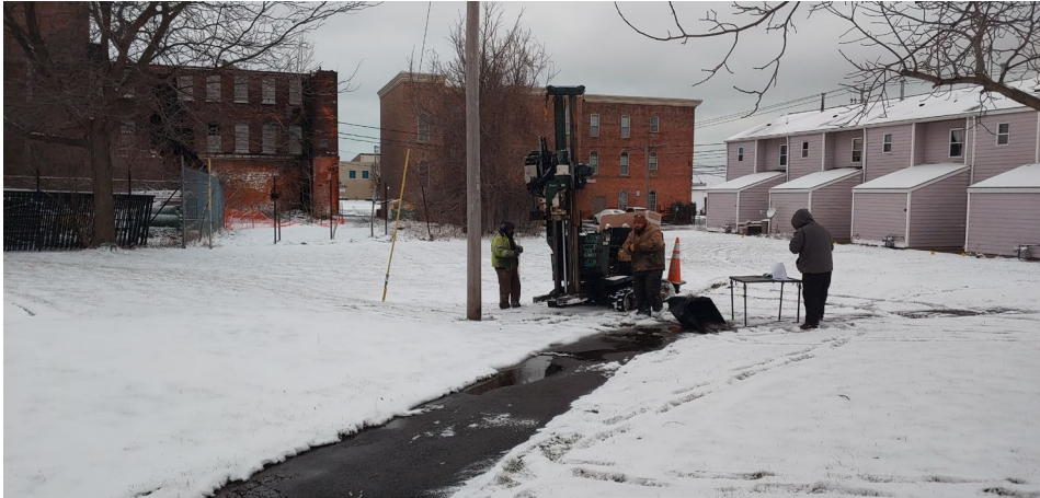
BH14 Location. (Facing Northwest)
