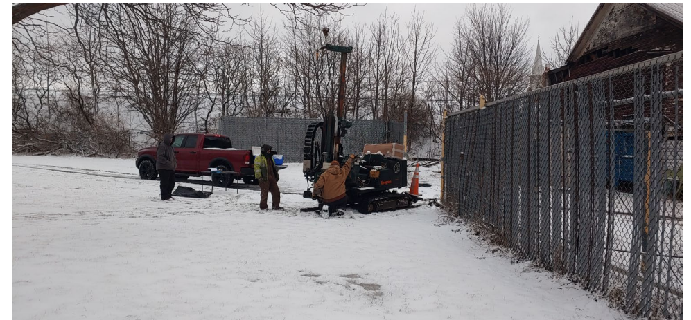
BH6 Location. (Facing South)
