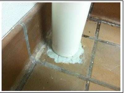
View of the wall penetration at suction point #2 in the produce and floral prep room after the sealant was applied.
