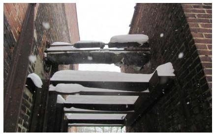
63. Piping between former pump house and boiler room; potential asbestos
