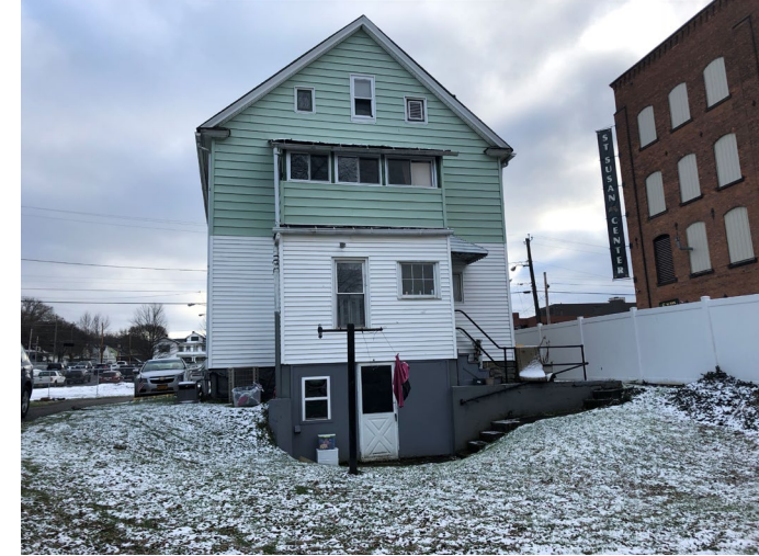
Rear of 53 Water St looking south.
