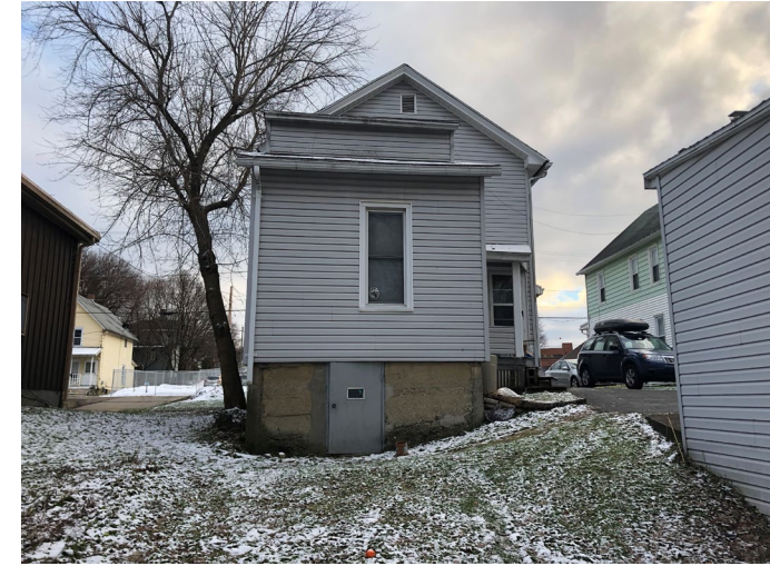
Rear of 55 Water St. looking south.
