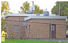
**reating iny(C%(ori e in rinking ater wit% e) o a(E iciency** The Cedarburg, Wisconsin Light and Water Utility installed an E-Z Tray Air Stripper in a discreet addition to their existing production pump building to treat groundwater containing vinyl chloride that has been traced back to a nearby landfill.
