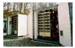
sing a Co) pact esign to reat a aso(ine Spi(( in a esi entia( rea A petroleum company installed compact E-Z Tray Air Strippers on a small lot in a high-end residential neighborhood on Long Island, New York. Compact shipping containers were used to house three E-Z Tray units and other equipment in the same space that would have been totally filled by just one traditional stripper.
