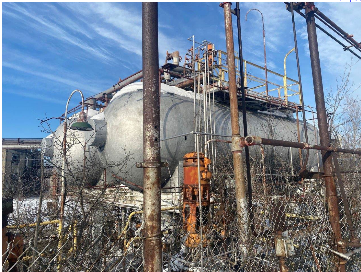
Photograph No. 3 – Abandoned Tanks (Northeast corner of AOI 2) – Note Fire Suppression Systems Surrounding Tank
