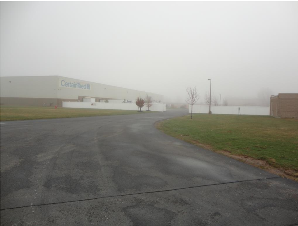
Photograph 12 – Distressed vegetation along edge of main entrance road heading to loading docks
