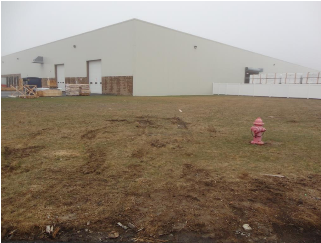
Photograph 7 – Ruts in grass at south end of building
