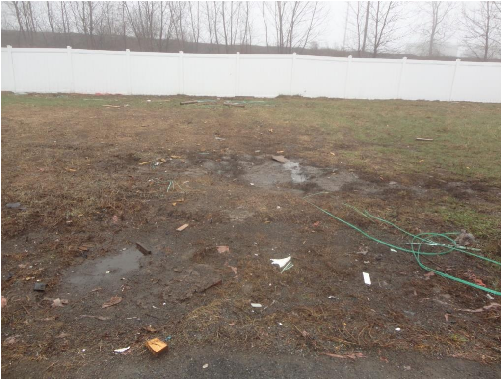
Photograph 9 –Distressed vegetation in Storage Yard
