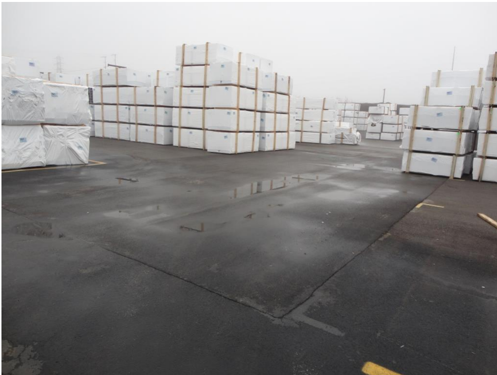
Photograph 4 – Area in central Storage Yard milled and repaved in 2014
