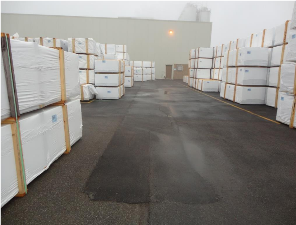
Photograph 1 – Area on east side of Storage Yard milled and repaved 2014
