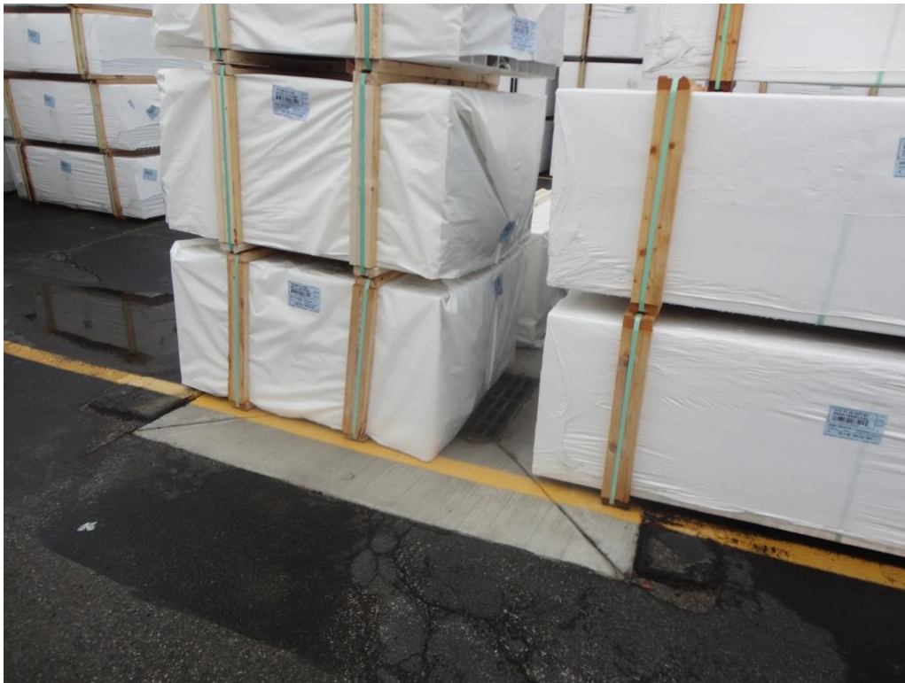
Photograph 2 – New catch basin apron installed 2014
