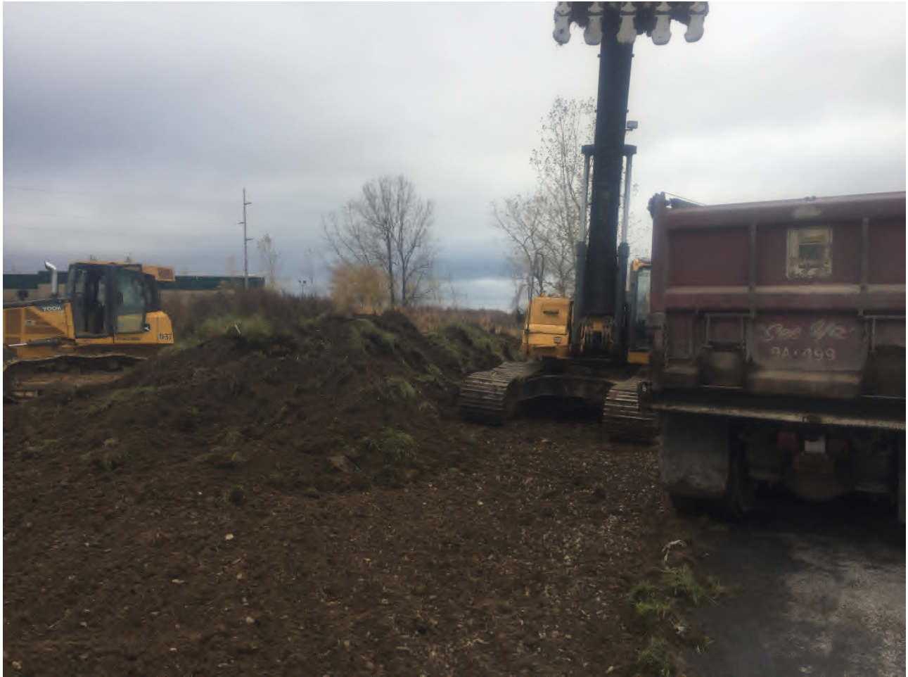
Segregation of Clean cover soil for reuse.
