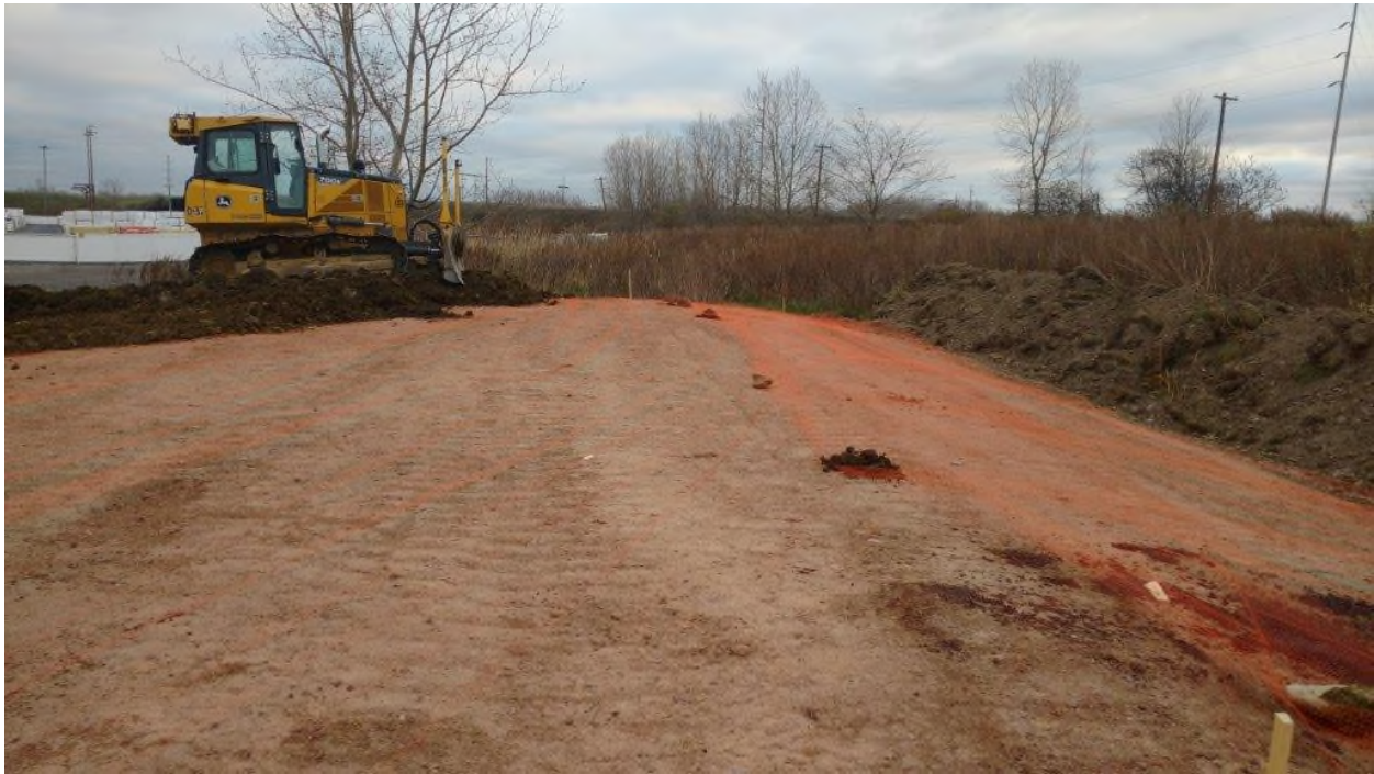
Placement of clean soil cover onto new demarcation mesh.
