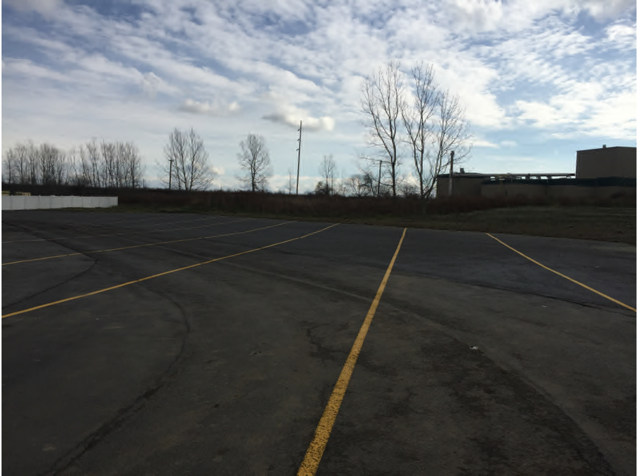
Finished pavement, SW area.
