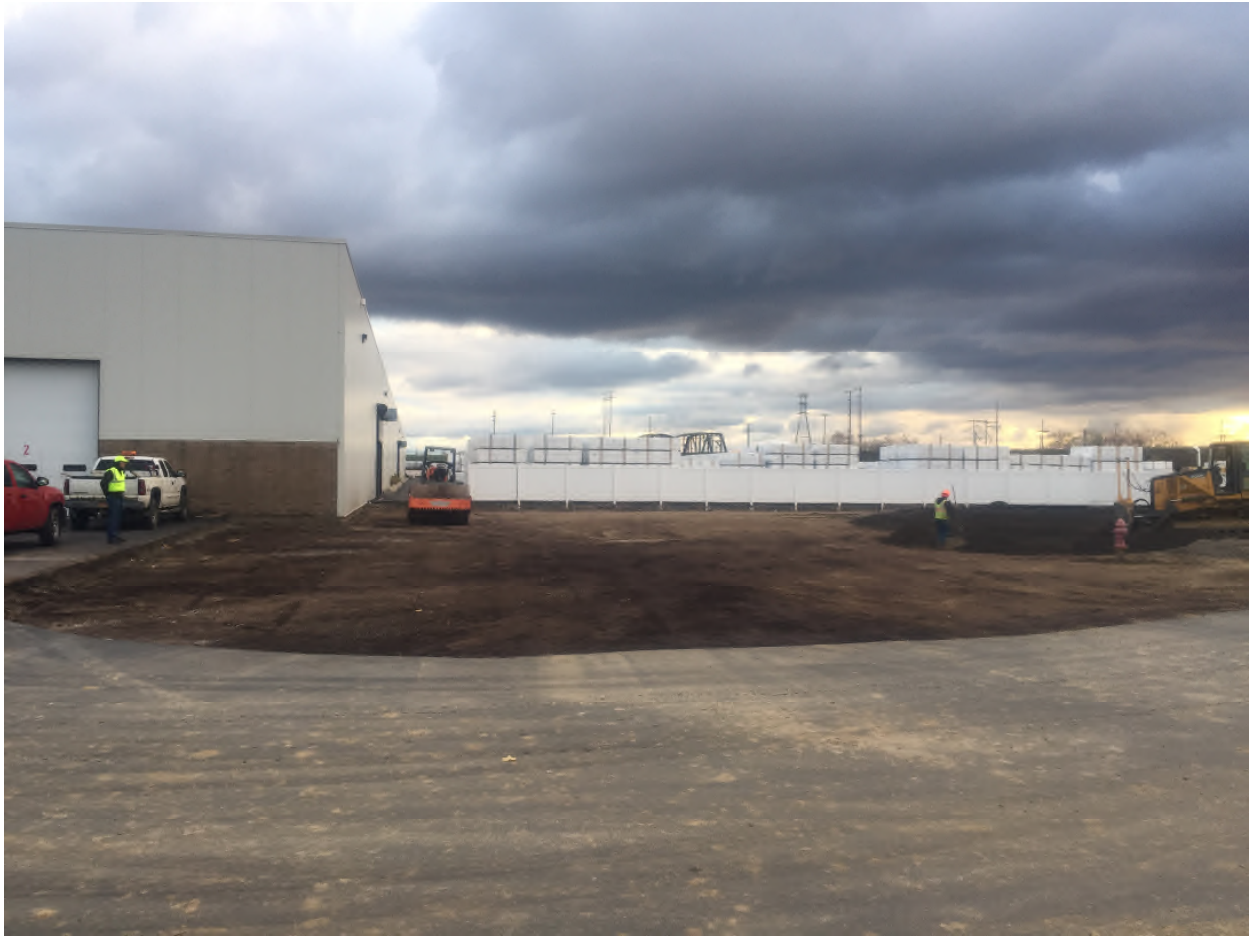
Rolling subsurface soil/fill and placement of pre-pave stone layer
