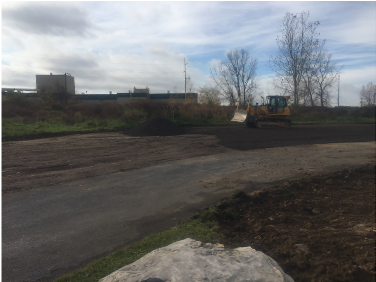
Placement of pre-pave stone layer.
