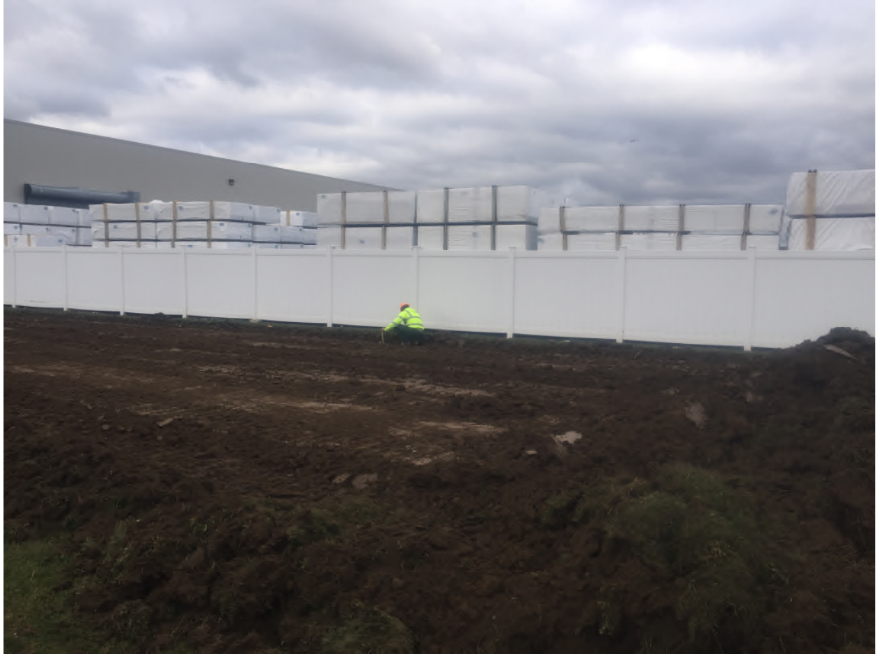
Removal of clean cover soil.
