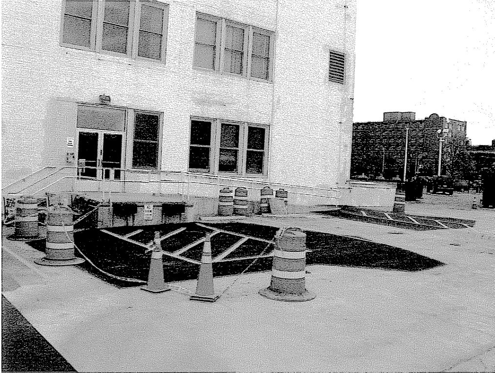
Photo 3: Completion of paving activities. EBEX-1 is the paved area on the right side of the photo. View is northwest.
