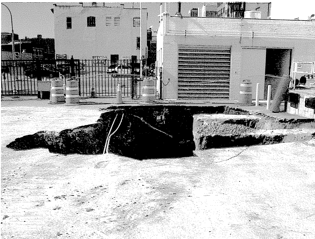
Photo 2: Final excavation limits of EBEX-2. View is south.
