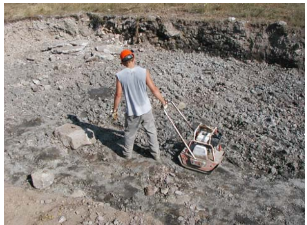
Finally the bottom is tamped
