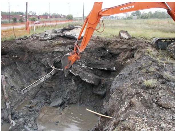
Massive concrete and metal pieces are encountered on the north side of Area A
