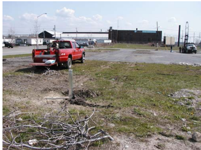
Casing for MW-1 is installed. The drilling rig in the background is starting MW-2
