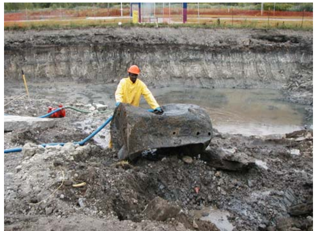
Water pumped from Area A is used to clean UST-2. The water runs back down into the hole.
