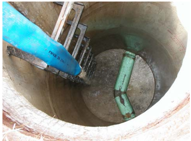
The treated water is discharged into the Sanitary Sewer at the southeast corner of the job site
