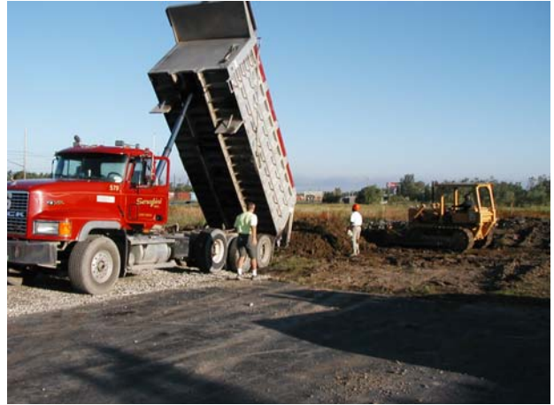
The bulldozer pushes fill into Area D
