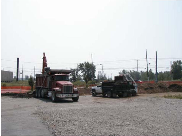
Bank Run Gravel is delivered ...
