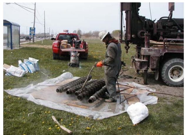
At the end of the day, drilling equipment is decontaminated
