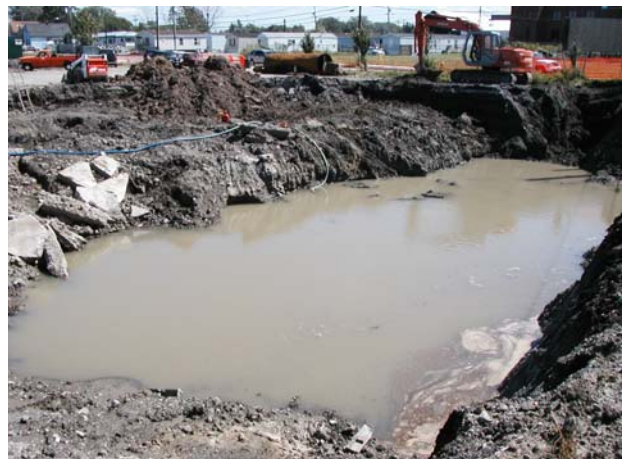
Then pumped the diluted water (mostly rainwater) directly into the Sanitary Sewer
