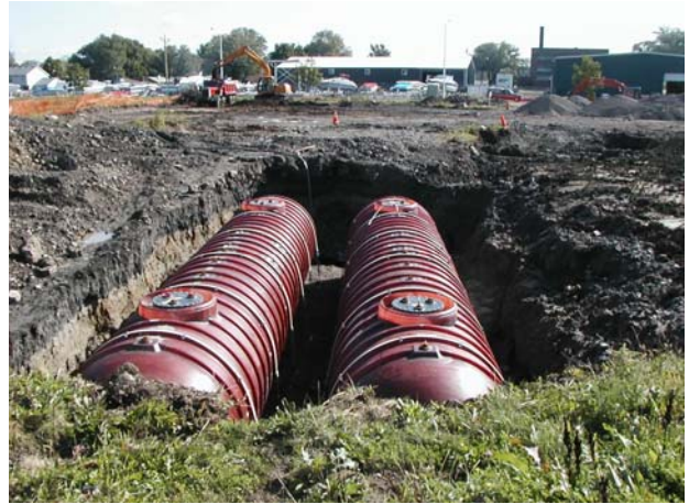
The New USTs are in the hole
