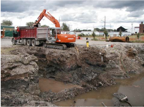
PITD excavator puts dam in hole to separate the water muddied from digging and the water being pumped out
