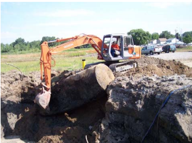
Excavating the UST
