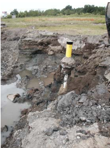
PW-1 about to be pulled out
