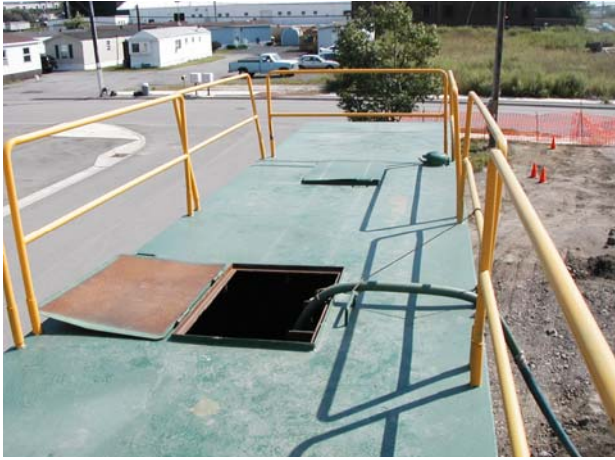
Top of Baker Tank showing hose that conveys the water from Area A
