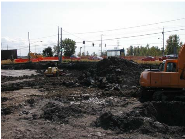
New Tank Area excavated material is piled next to the hole...
