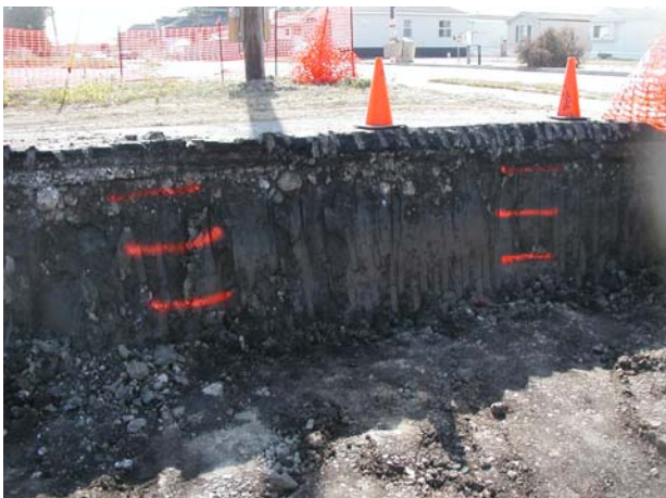
Lines are painted on the walls 1' apart. The gravel will be added and tamped intermittently.
