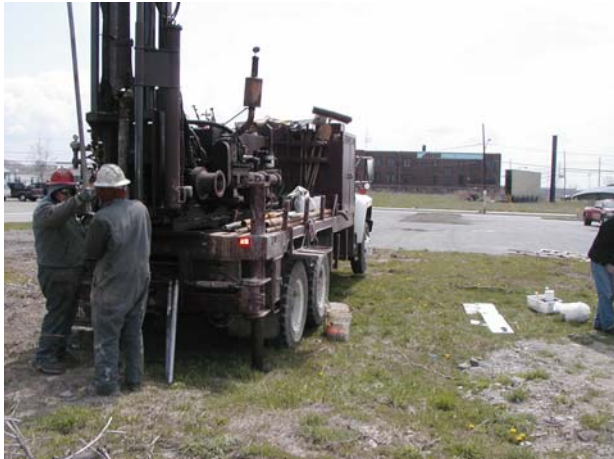
Starting to drill MW-1
