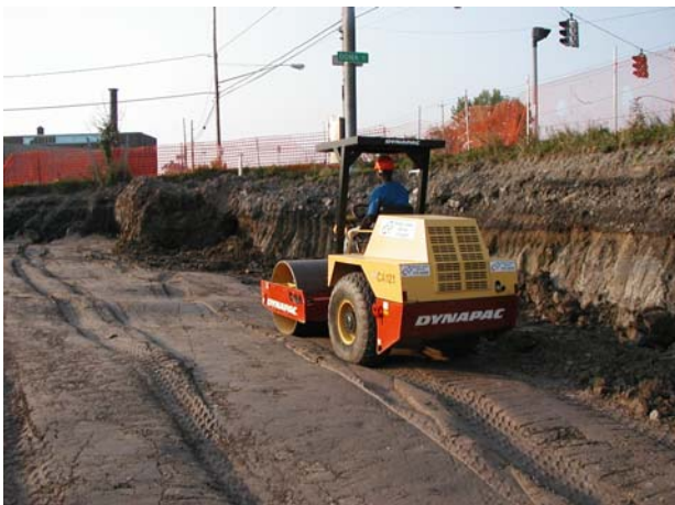
The material is rolled intermittently...
