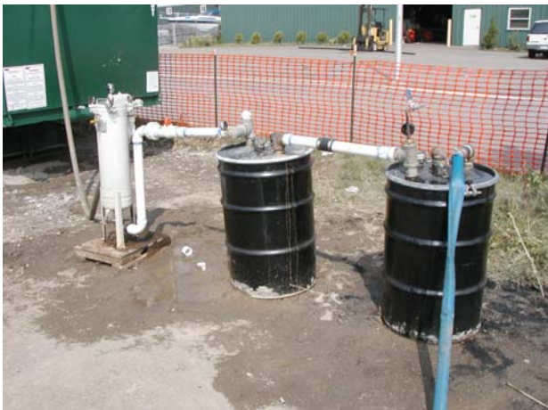
The Water Treatment System: (1) bag filter and (2) carbon drums
