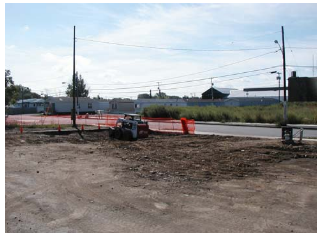
The west half of Area E is brought up to Area C grade so that one of the driveway entrances can be used
