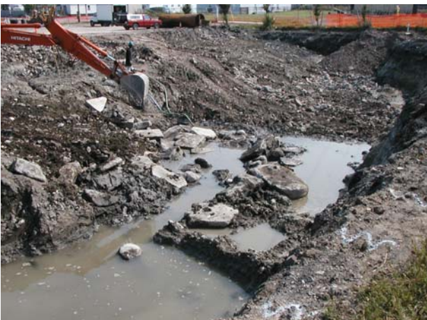
Large pieces of concrete are pushed into the bottom
