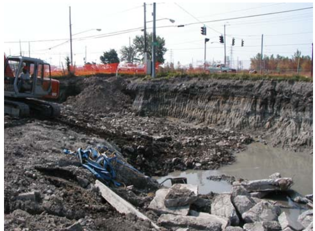
Backfilling starts at the south end of Area A/B and progresses to the north
