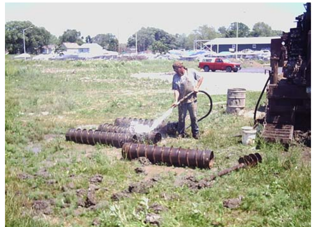
Decontaminating augers on site
