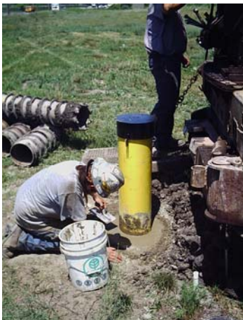
Finishing the concrete at grade
