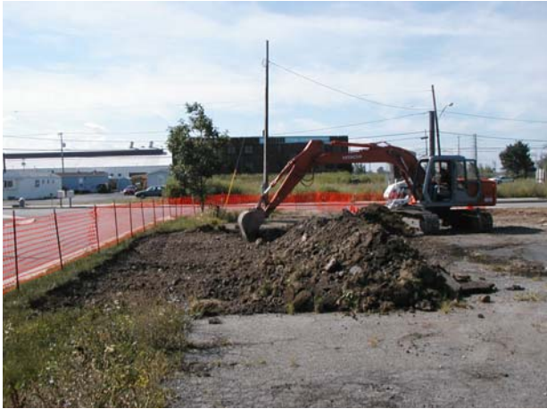
The top 1' of Area C along the eastern border is scraped away in preparation for the Baker Tank
