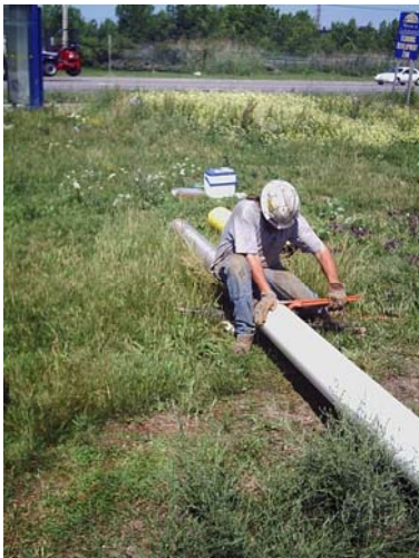
Attaching the PVC riser to the stainless steel bottom
