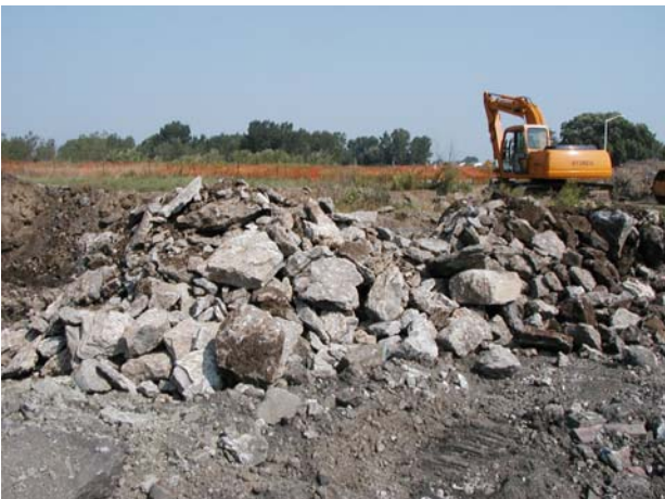
Pile of shot rock will be pushed over the large pieces of concrete at the bottom of the hole
