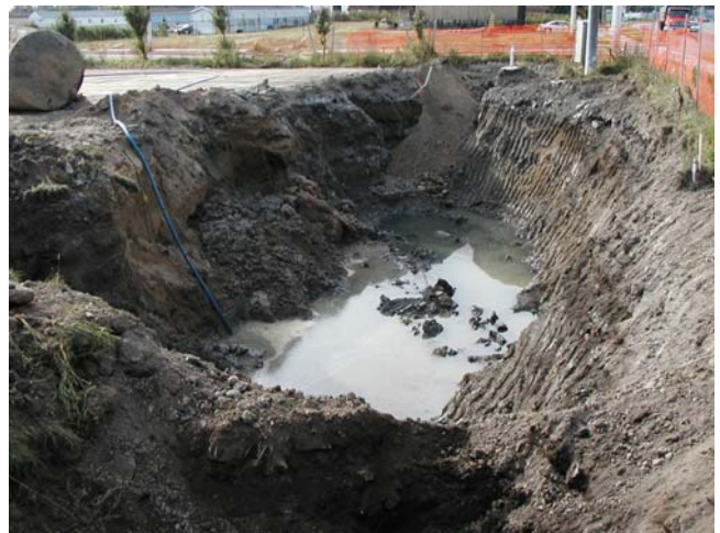
Small pipes are encountered just north of where UST – 1 was pulled
