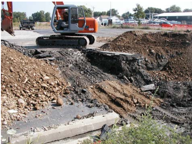
A ramp is made in the northwest corner to access the bottom
