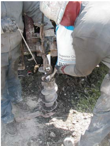
Adding sand to MW-1
