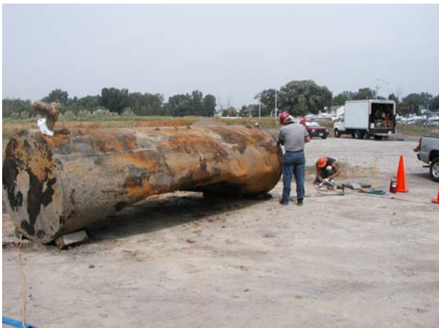
Sawing the ends off of the UST
