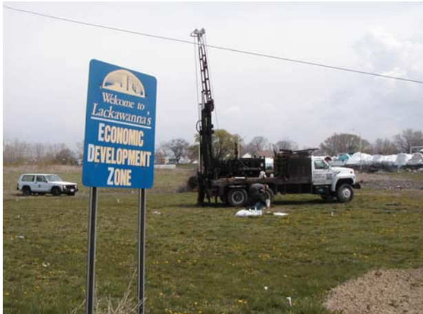
SJB crew drills SB-10 while IEG field technician collects soil samples and tests for VOCs
