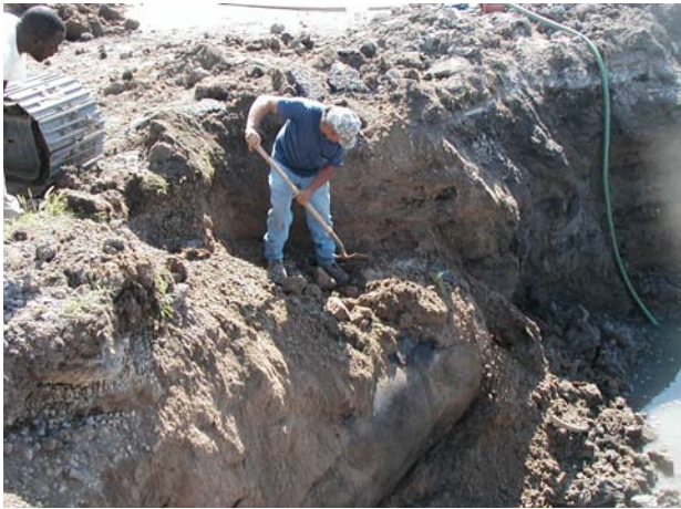
A UST is discovered on the east border of Area A
