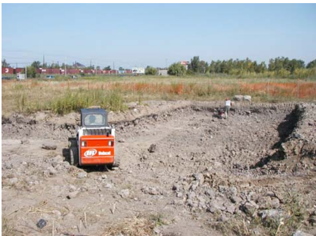
Skid Steer smoothing out the bottom
