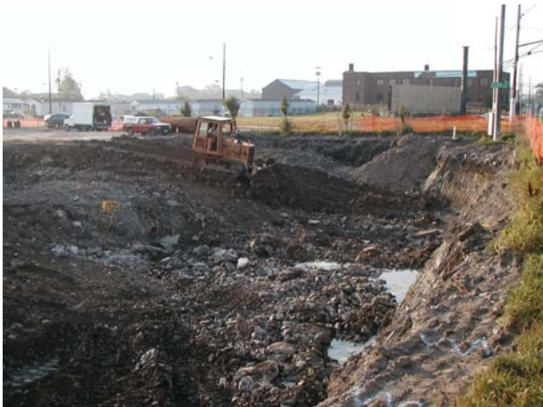
The bulldozer pushes the clay into the south end...
