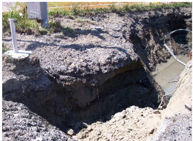
MW-3 at the south end of Area A. Several yards distance was kept around the light pole to maintain stability.
