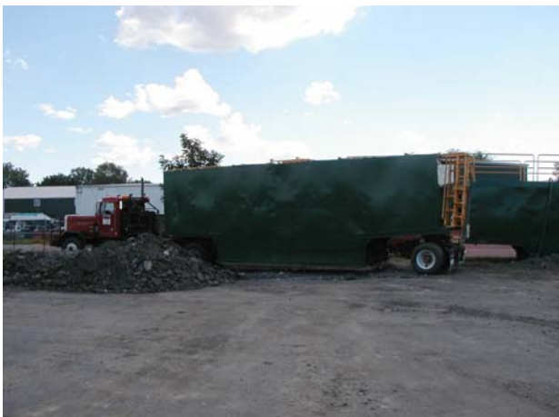
As the excavated area gets larger, a second Baker Tank is mobilized
