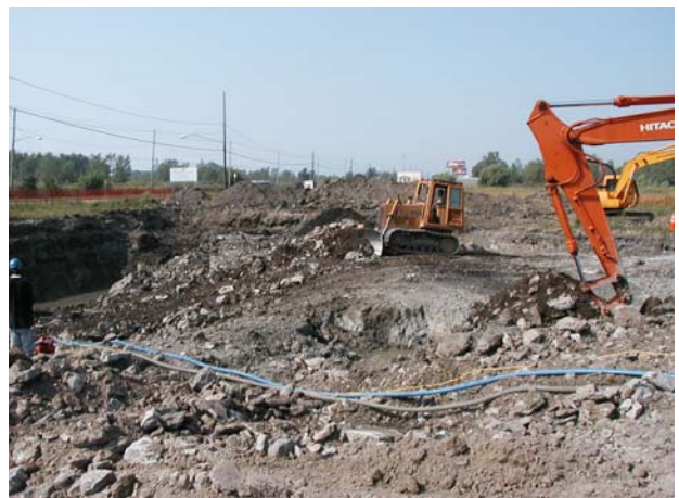
Bulldozer pushing shot rock into hole
