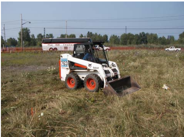
The Skid Steer pushes debris out of the way and knocks down the vegetation
