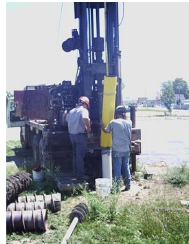
Lowering the metal casing over the plastic riser
