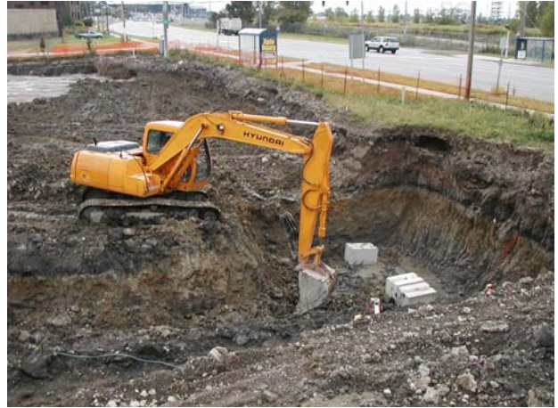
Acome Construction excavates for the new USTs
