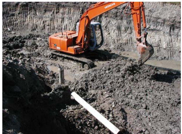
Excavator scraping down to the bedrock at the bottom of the hole
