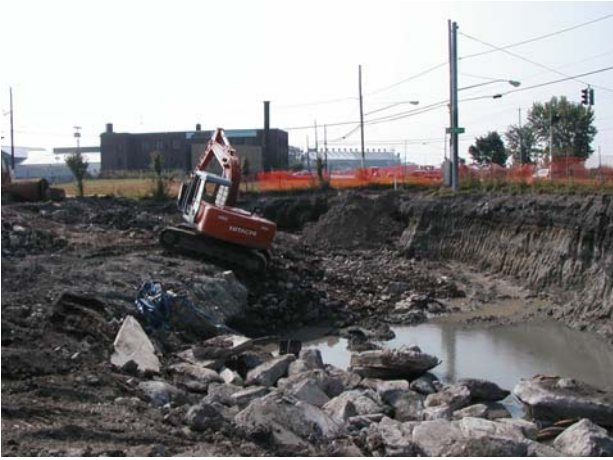
Large pieces of rock and concrete are placed at the bottom of the hole.
