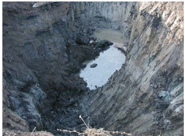
The hole begins to fill with water once 12' is reached
