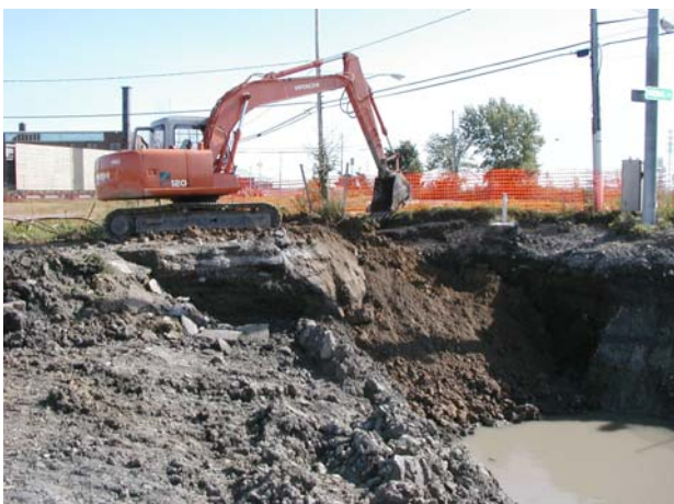
This area is quickly backfilled to prevent losing the stability of either MW-3 or the Traffic Light Pole
