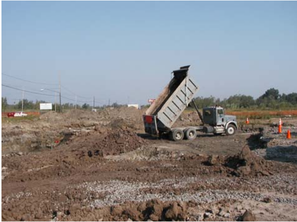
After all the rock is spread, loads of clean clay fill arrives in Tandem Dump Trucks...
