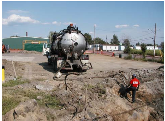
Pumping out contents of UST - 1
