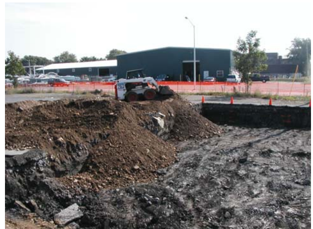
After the bottom is tamped, the gravel is pushed in
