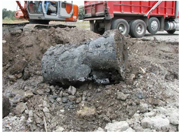
The UST is badly corroded and its contents (mostly water) spill down into the bottom of Area A
