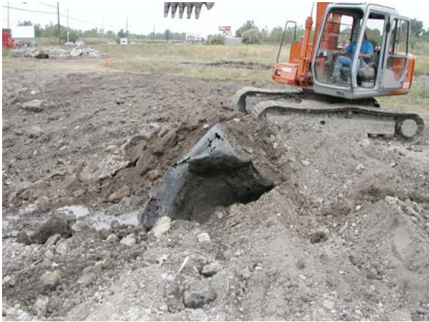
A UST of approximately 550 gallons is uncovered
