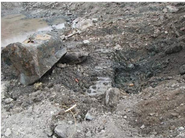
There is a concrete footing where the UST was buried
