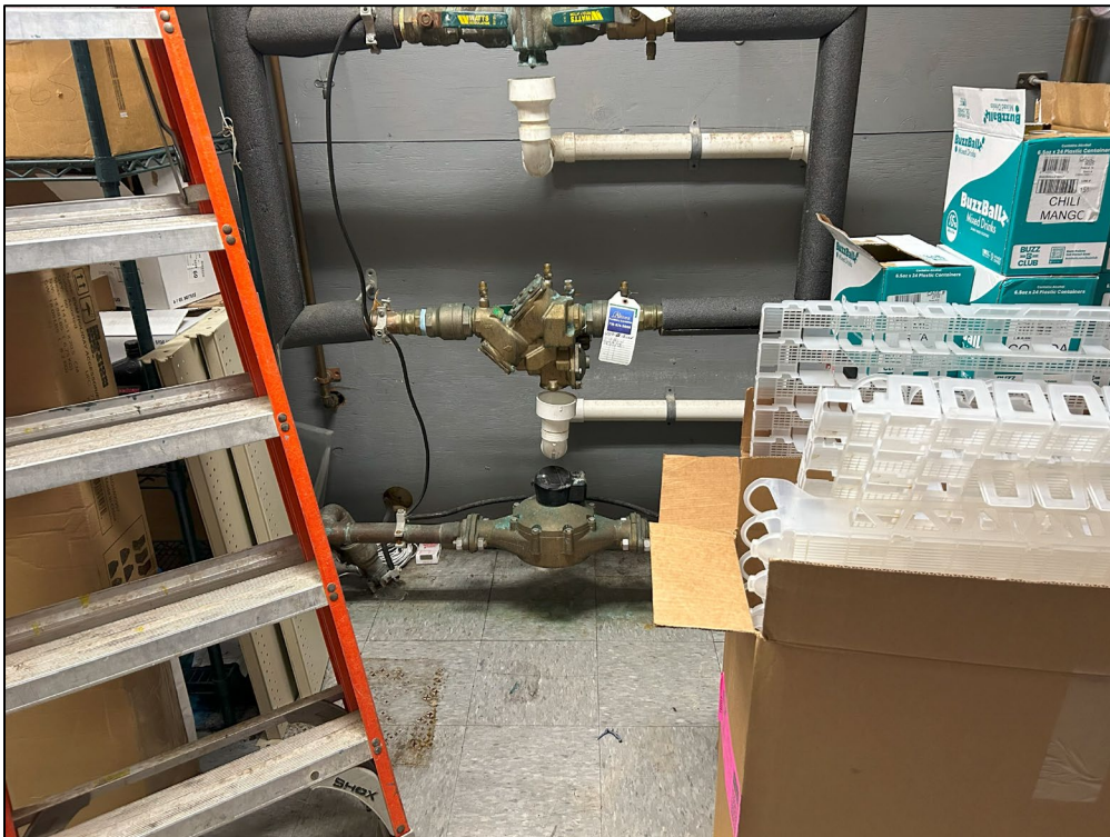
Photograph 10: Municipal water connection inside station building.
