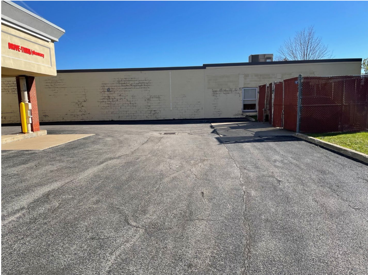
Site conditions facing east.
