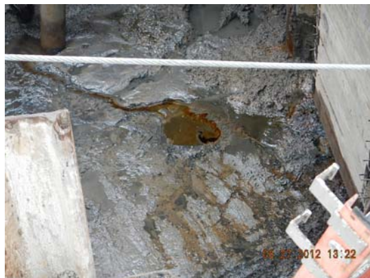
Looking southeast. Coal tar entering excavation from beneath Fourth Street (on the right).
