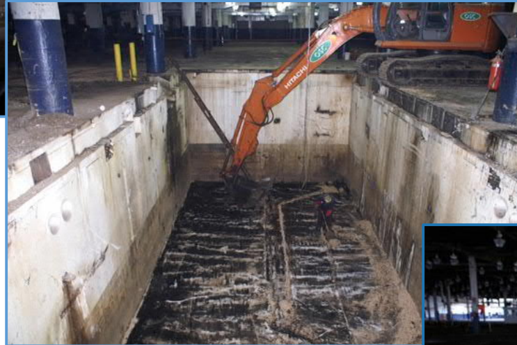
Typical Cleaning of Pit/Sump in Former Machining Area
