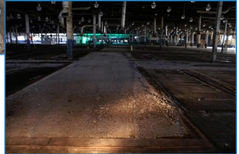
Typical Backfilled Pits/Trenches in Former Machining Area
