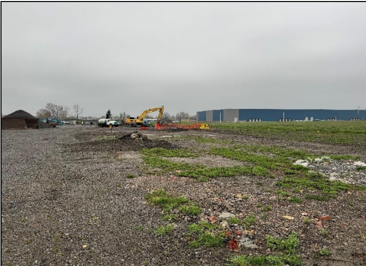
I-1 facing east
