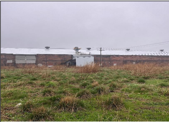
I-9 facing west
