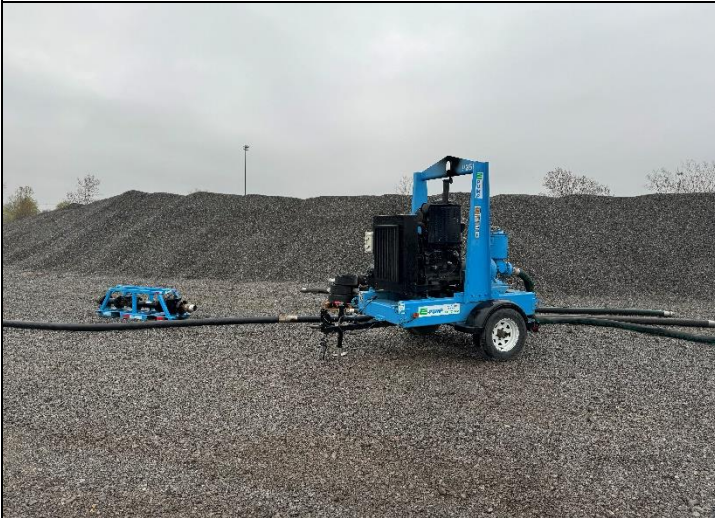
I-3 facing east
