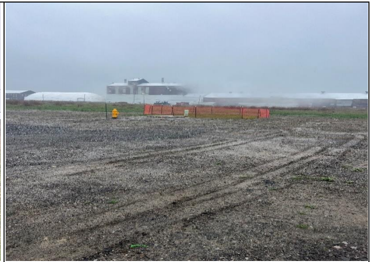
I-9 facing west Disturbed area due to water/sewer line installation
