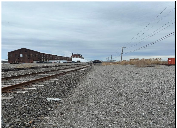
Typical View of railroad tracks (near I-3)
