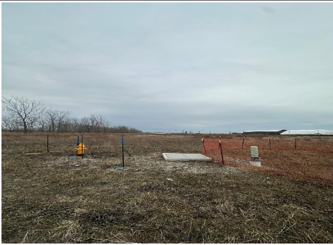
I-9 facing south Utilities constructed on site
