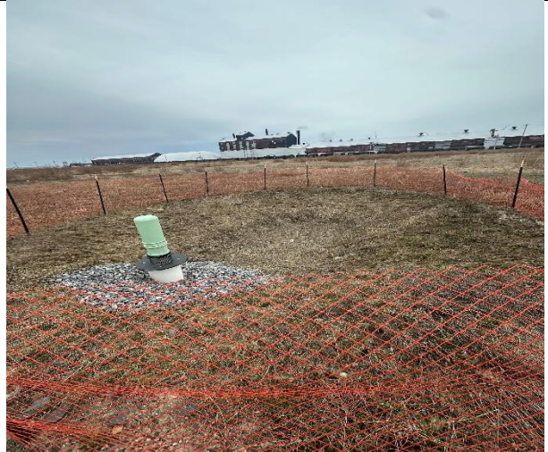
I-9 facing west Utility constructed on site
