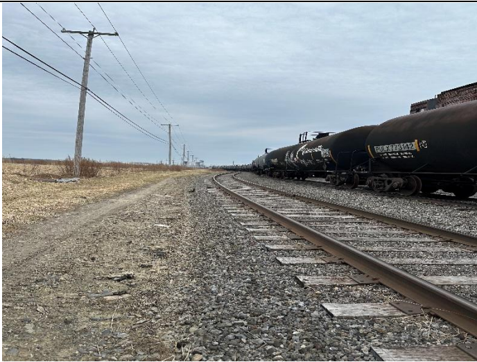
Typical View of railroad tracks (near I-5)
