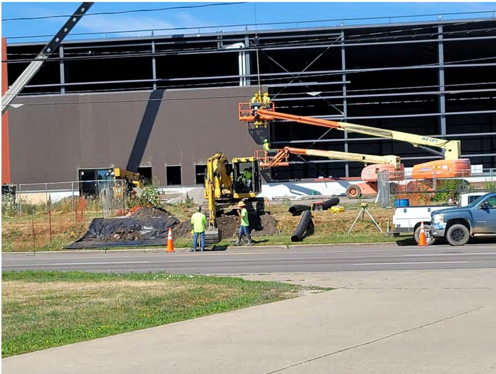
*Photo 4-Excavation across Greenway trail for stormwater connector*
