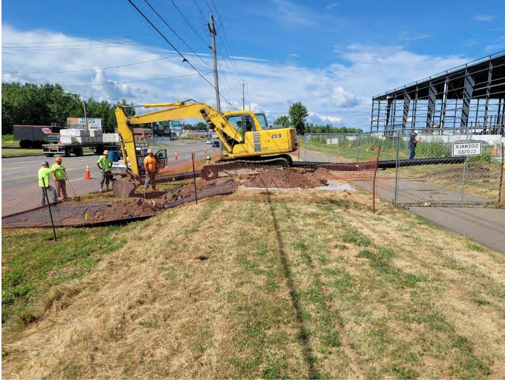
*Photo 3-Excavation across Greenway trail for stormwater connector*
