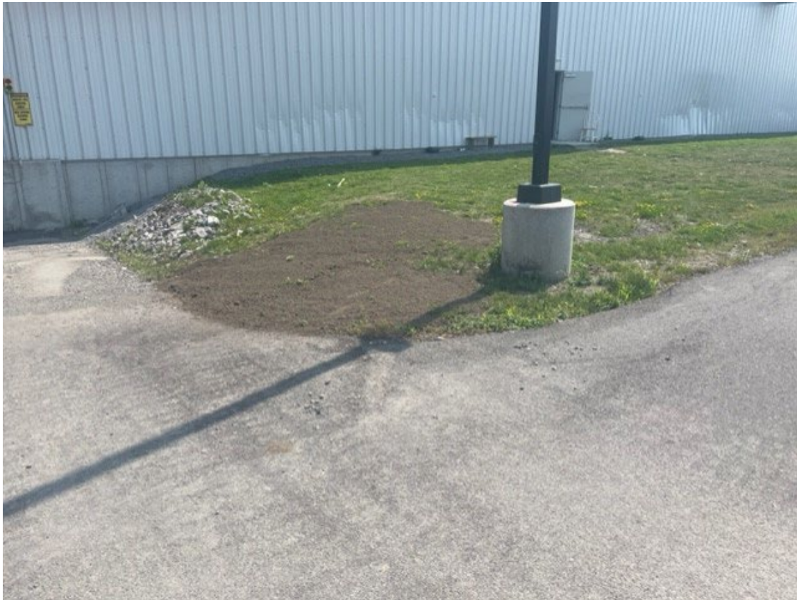
Photograph 7: 5/30/2023 – Topsoil repair from snowplow damage at the northeast corner of the building near the loading dock located at the north end of the building (looking southwest).
