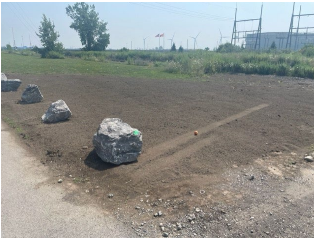
Photograph 12: 8/4/2023 – Topsoil cover repair from truck traffic along the west side of the truck driveway south of the access road (looking southwest).
