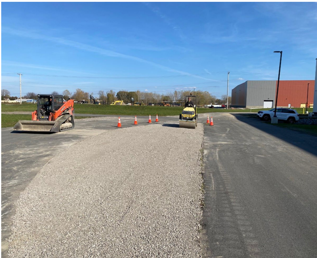
Photograph 5: 11/5/2022 – Placement of 2” ROC to expand the shoulder of the road north of the building (looking east).
