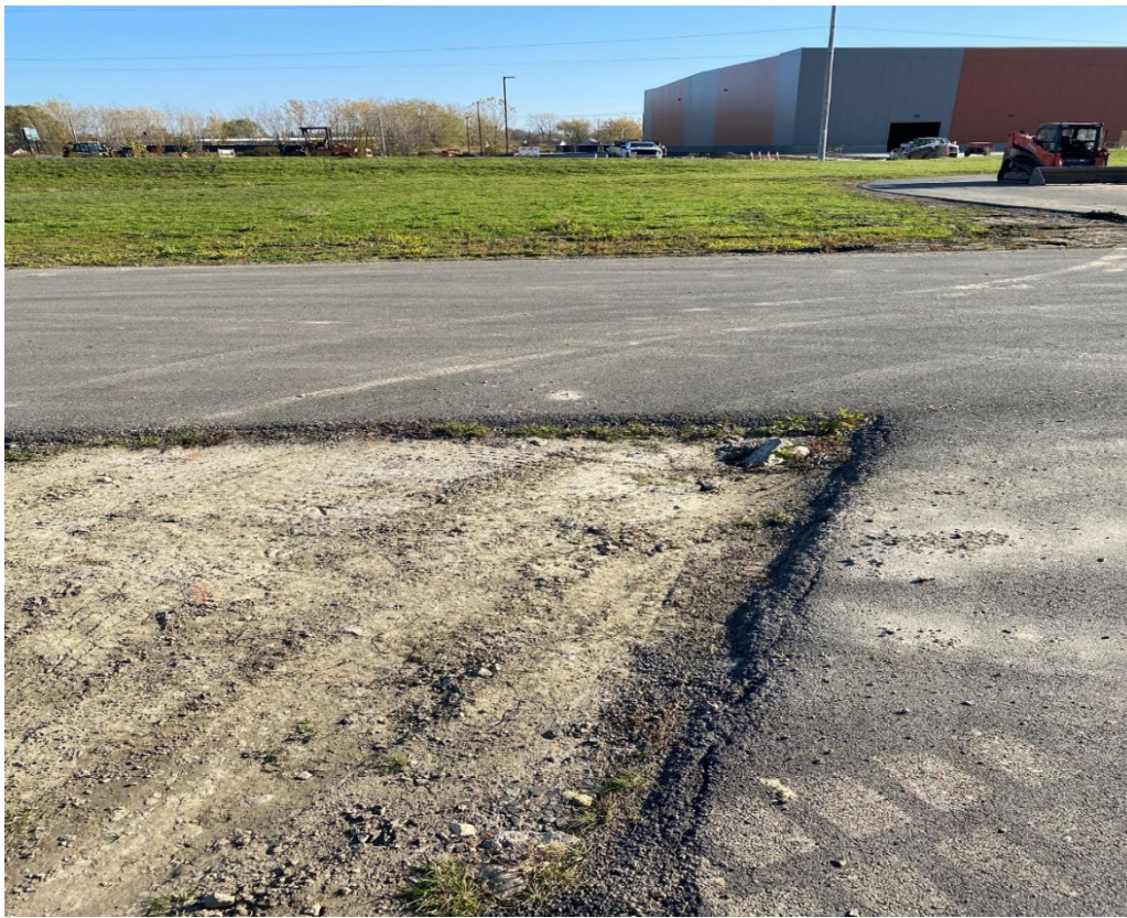
Photograph 1: 11/5/2022 – Removal of excess topsoil from the shoulder of the road in preparation of 2” ROC placement at the north end of the building (looking east).
