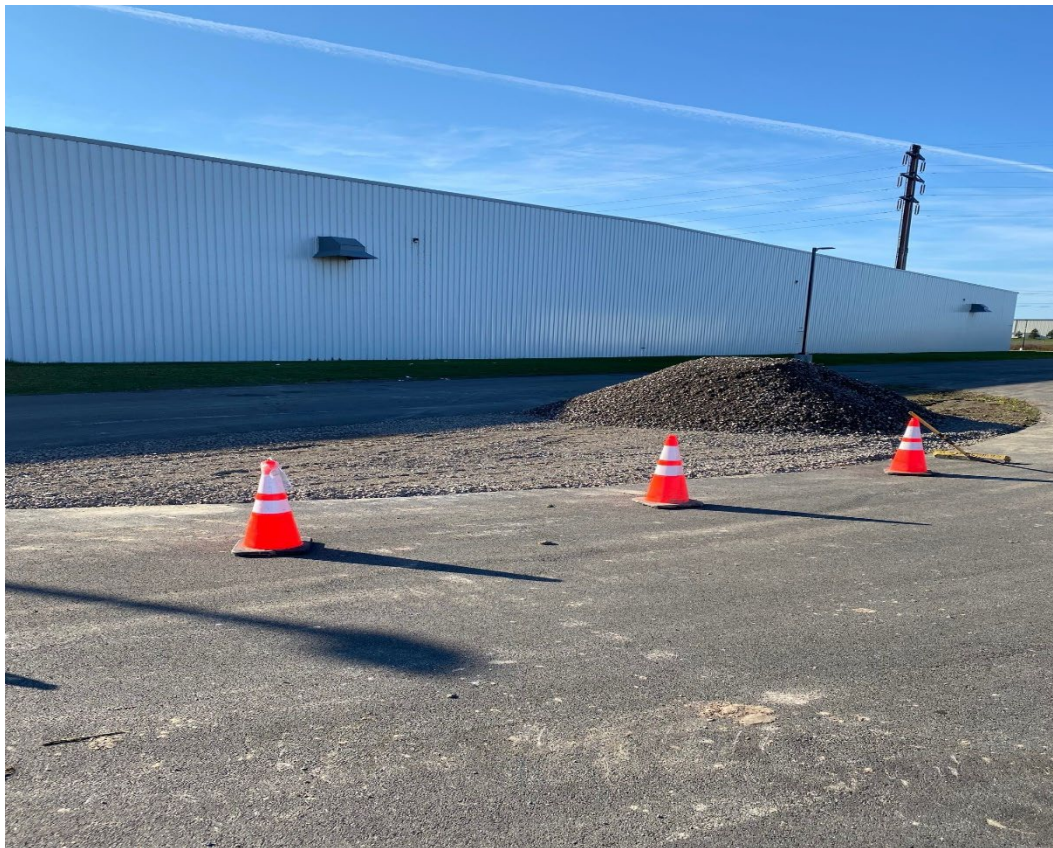
Photograph 4: 11/5/2022 – Placement of 2" ROC to expand the shoulder of the road northwest of the building (looking southwest).
