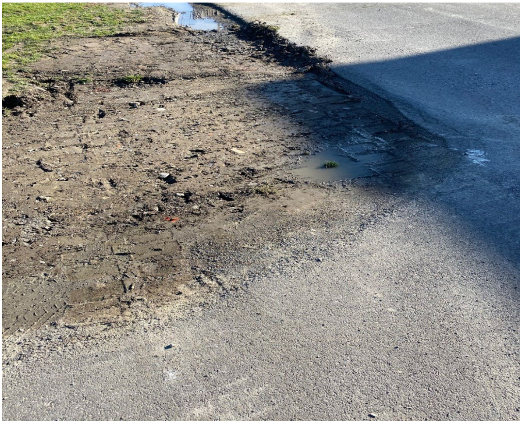
Photograph 2: 11/5/2022 – Removal of excess topsoil from shoulder of the road in preparation of 2” ROC placement at the north end of the building (looking east).
