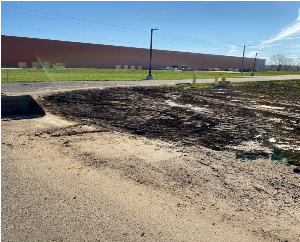
Photograph 3: 11/5/2022 – Removal of excess topsoil from shoulder of the road in preparation of 2" ROC placement at the north end of the building (looking southeast).
