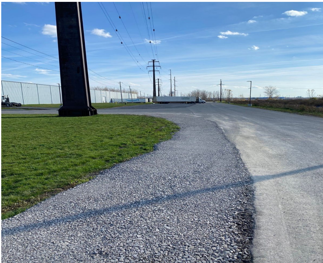
Photograph 6: 11/5/2022 – Placement of 2” ROC to expand the shoulder of the road west of the building (looking south).
