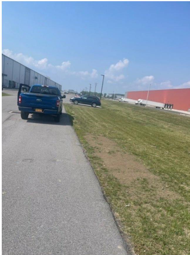
Photograph 9: 8/4/2023 – Topsoil cover repair from snowplow damage along the east side of the main driveway (looking north).
