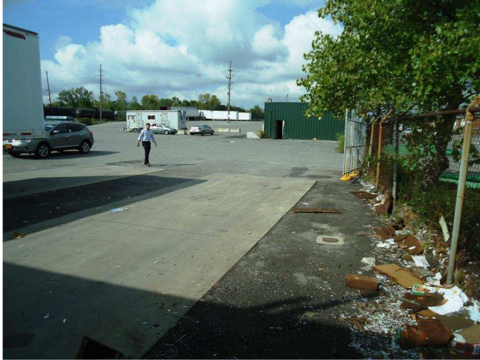
Photo 3 – Building Apron Concrete System looking west across MW-103.
