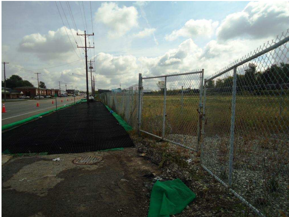
Photo 18 – Fence at northwest property boundary looking east-southeast. Soil cover work along Walden Avenue is in progress.
