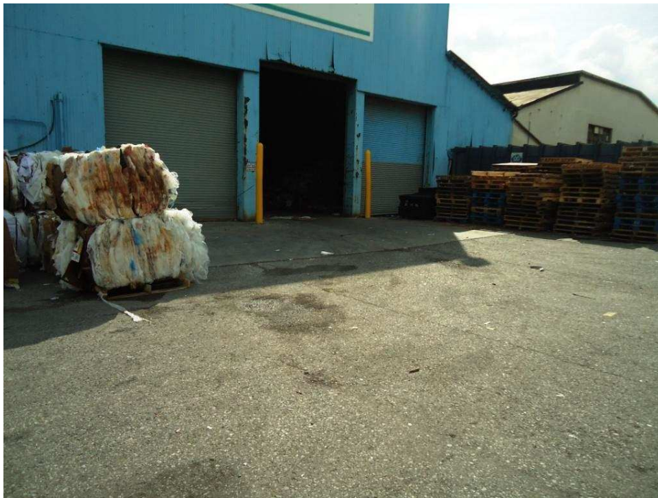
Photo 4 – Building Apron Concrete System looking southeast.
