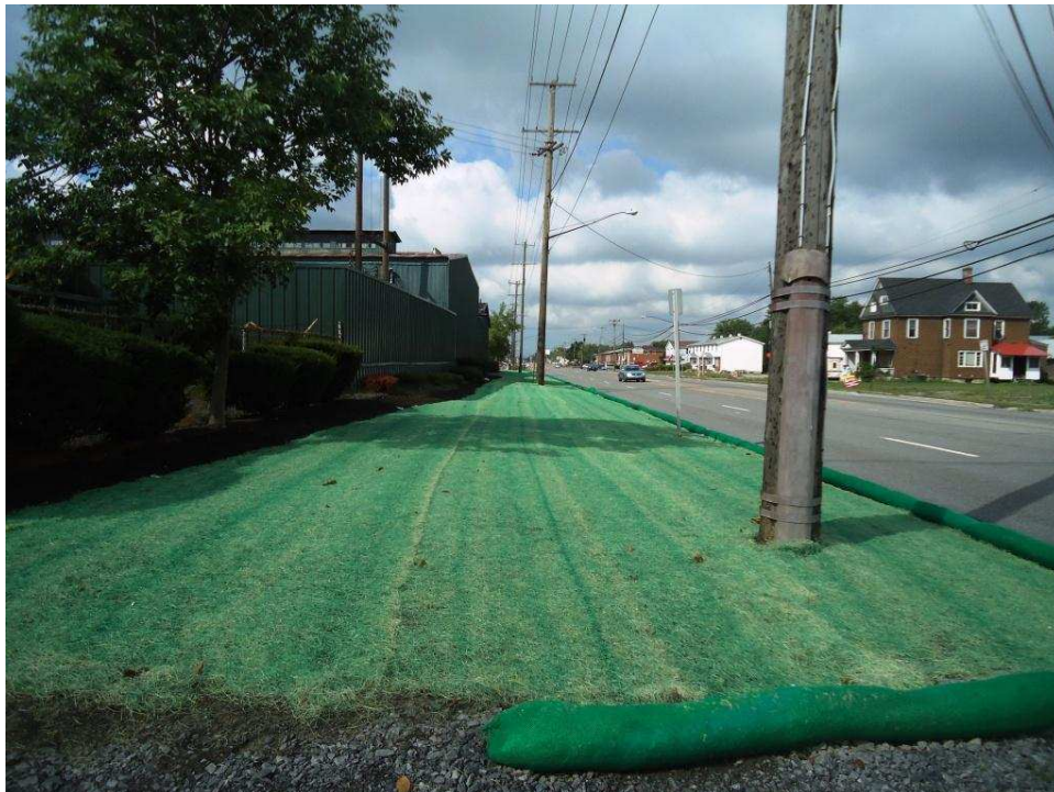
Photo 20 – Completed soil cover, looking west along Walden Avenue.
