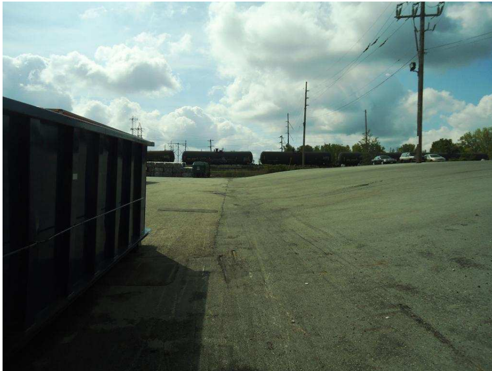
Photo 8 – GCL and Asphalt Cover System looking south across east slope.
