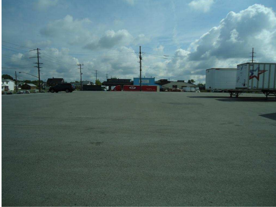
Photo 15 – GCL and Asphalt Cover System looking east across cap.
