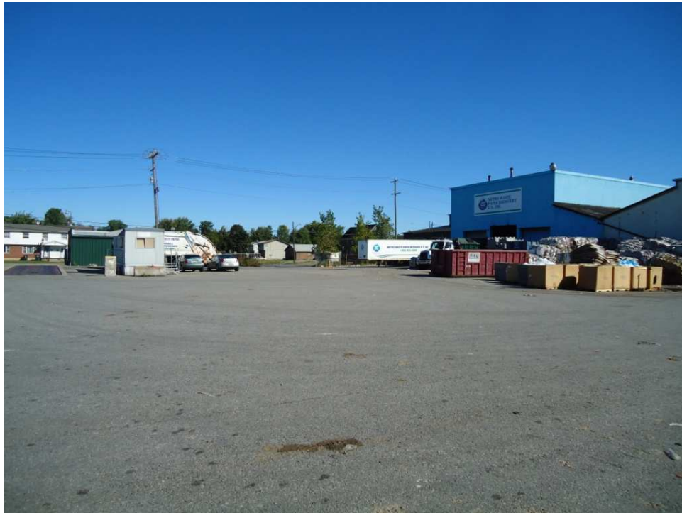
Photo 6 - Trucking Yard looking northeast.
