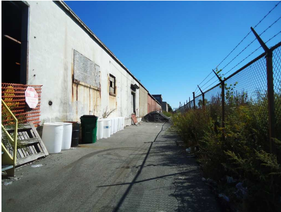
Photo 5 - Former Rail Siding looking east.
