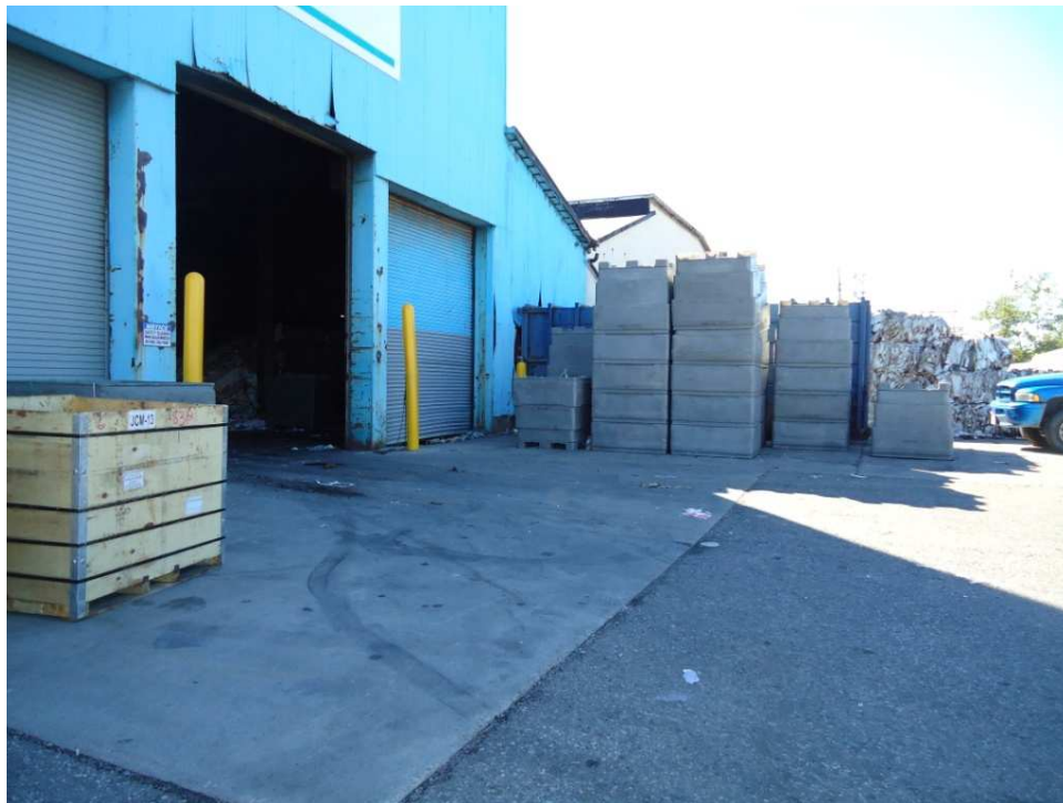
Photo 4 - Building Apron Concrete System looking southeast.
