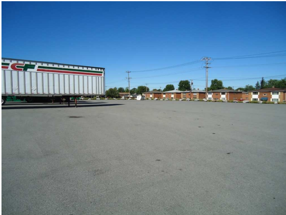
Photo 16 - GCL and Asphalt Cover System looking northeast across cap.
