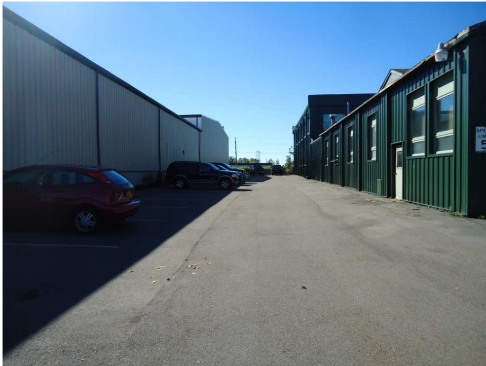
Photo 2 - Parking lot looking south.
