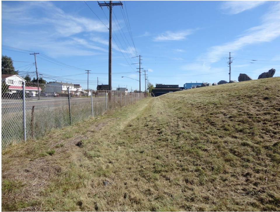
Photo 9 - GCL and Soil Cover System looking east along north slope.
