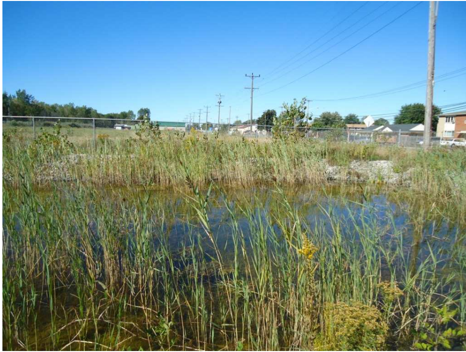
Photo 13 – Retention pond looking northwest.
