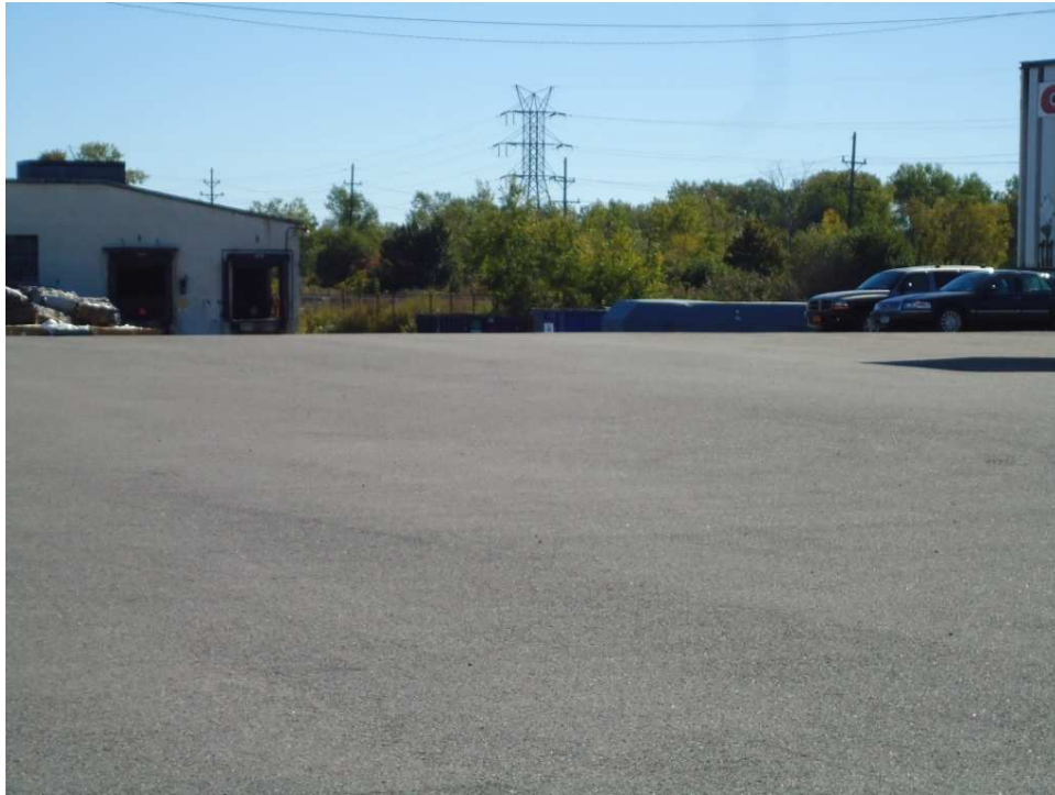
Photo 15 - GCL and Asphalt Cover System looking southeast across cap.
