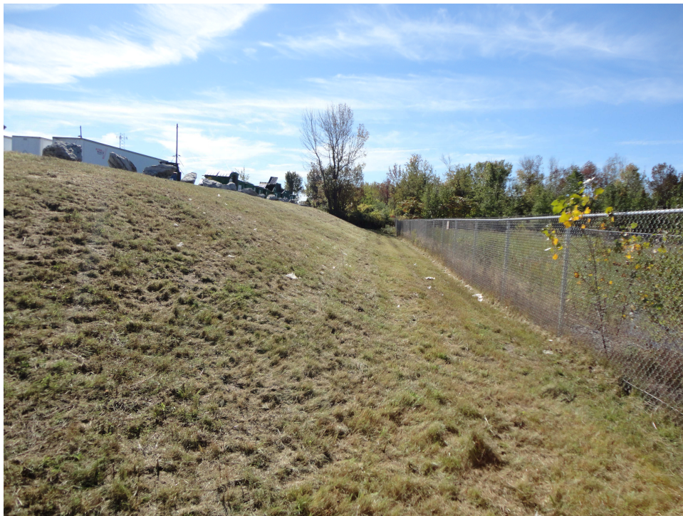
Photo 10 - GCL and Soil Cover System looking south along west slope.
