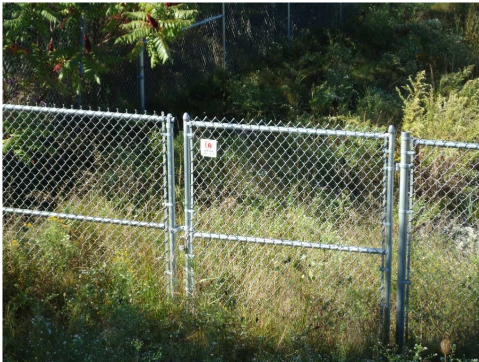
Photo 12 – Access gate at southeast corner of retention pond enclosure.
