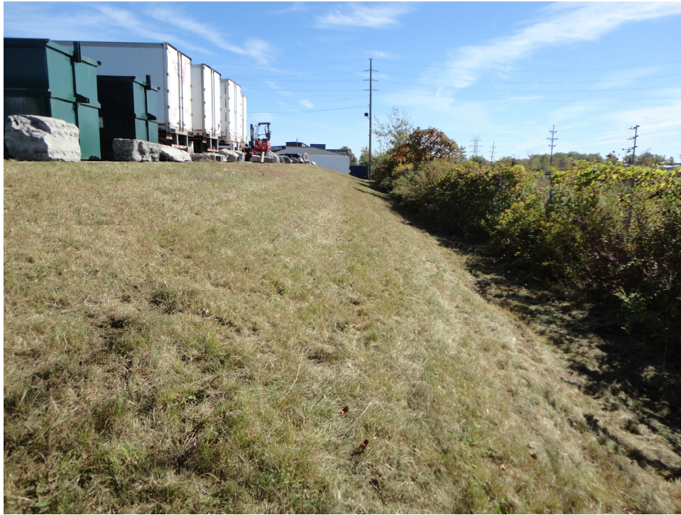
Photo 11 – GCL and Soil Cover System looking east along south slope.
