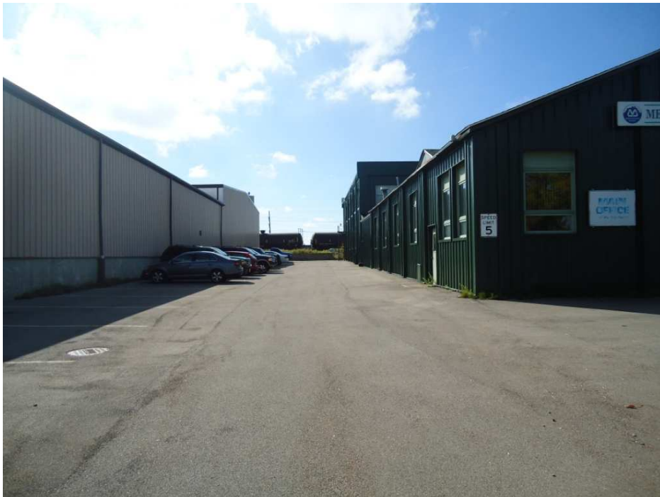
Photo 2 – Parking lot looking south.
