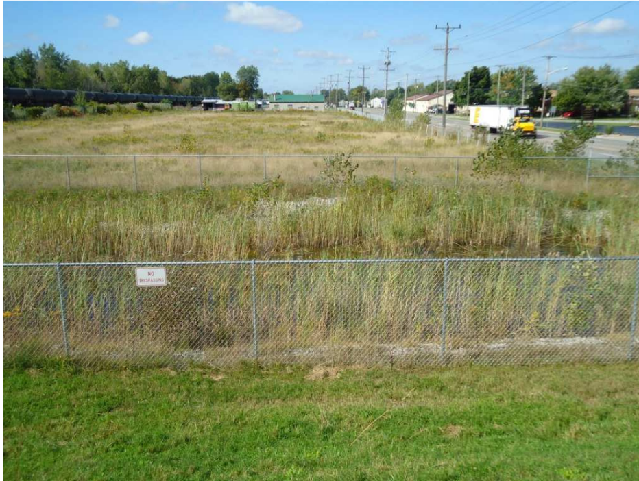
Photo 13 – North end of retention pond looking west.
