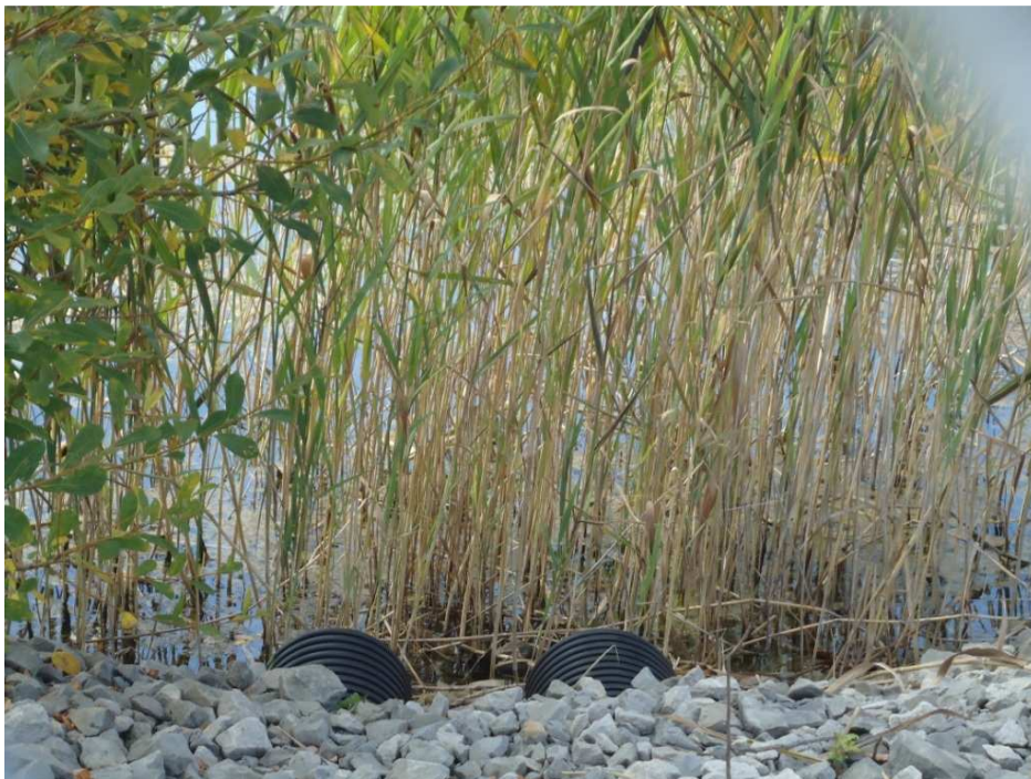
Photo 14 – Retention pond looking southwest across outlet pipes in northeast corner.
