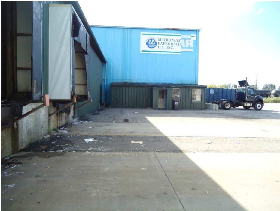
Photo 4 – Building Apron Concrete System looking south.
