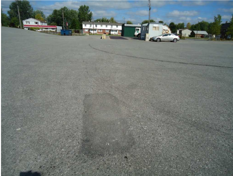
Photo 7 – Trucking Yard looking north.
