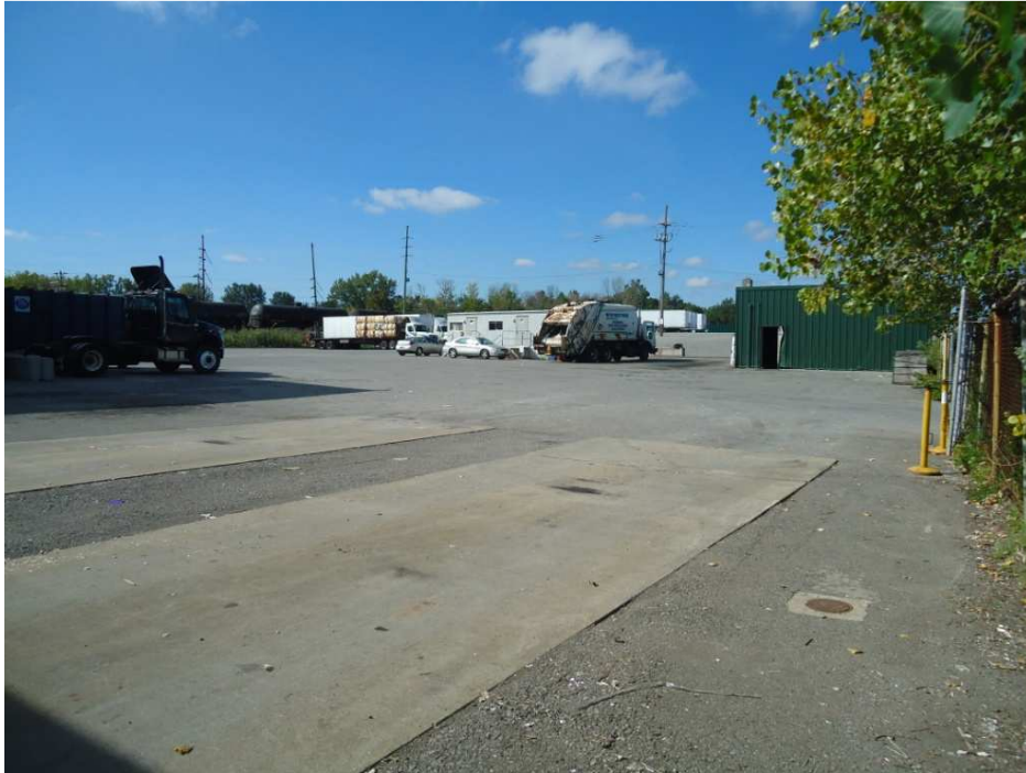
Photo 3 – Building Apron Concrete System looking west-southwest across MW-103.
