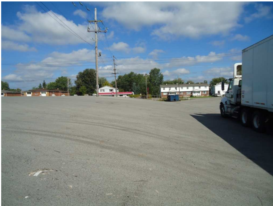
Photo 8 – GCL and Asphalt Cover System looking north across east slope.
