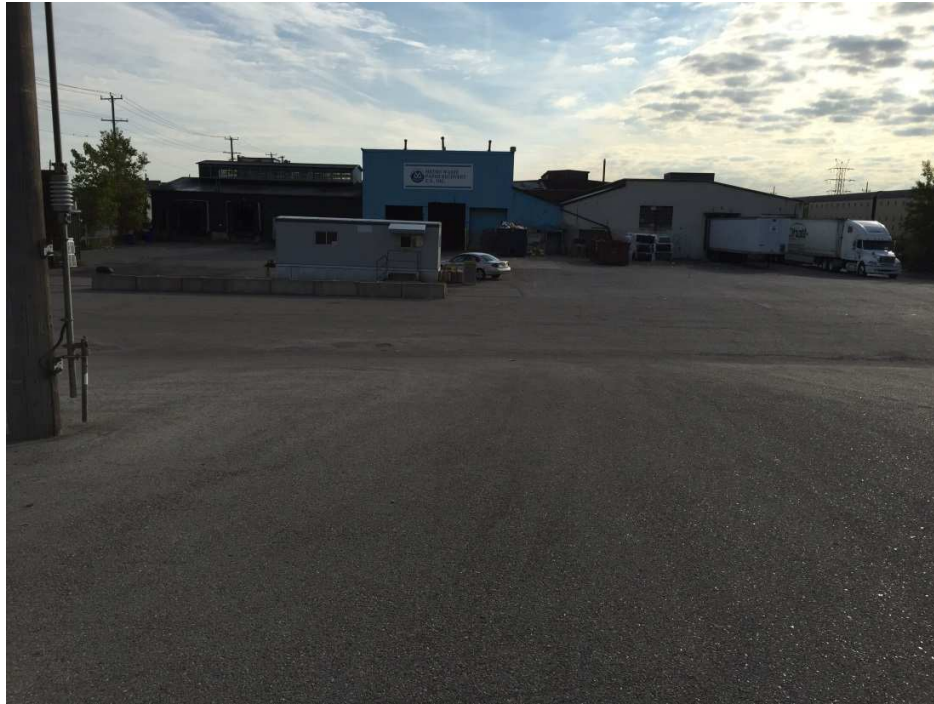
Photo 17 – GCL and Asphalt Cover System looking east down slope.
