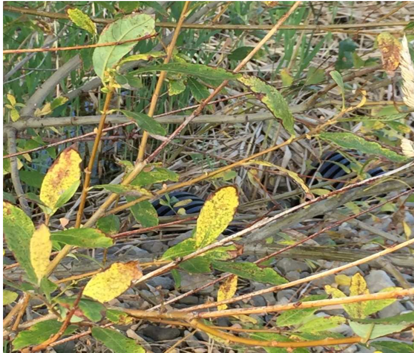
Photo 15 – Retention pond looking southwest across outlet pipes in northeast corner.
