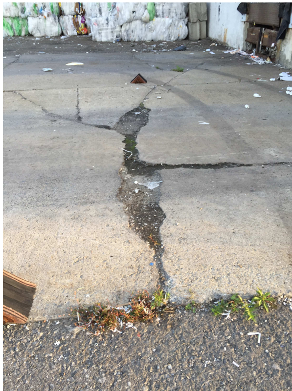
Photo 6 – Building Apron Concrete System (south end of building) looking north.
