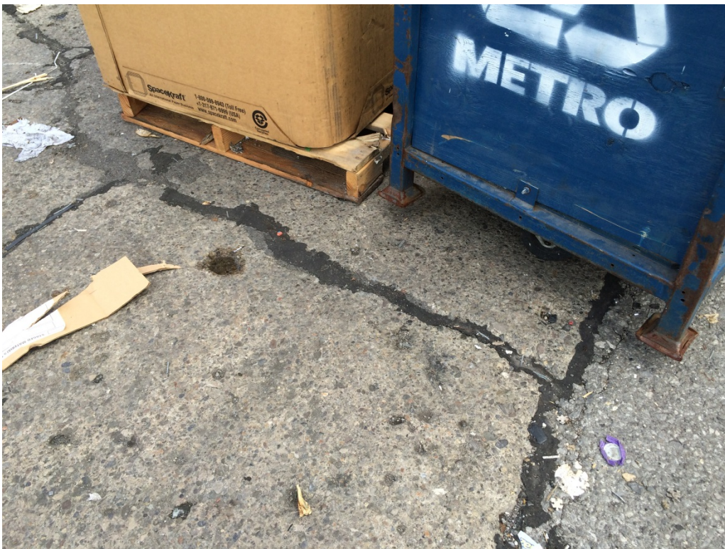
Photo 6 – Building Apron Concrete System (close-up of repaired cracks).
