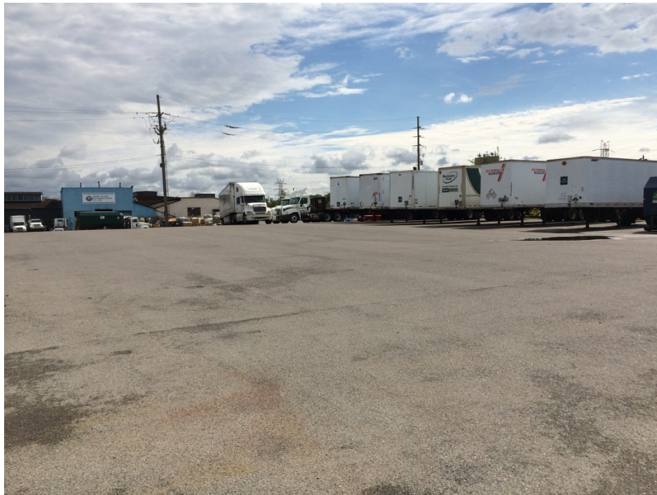
Photo 17 – GCL and Asphalt Cover System looking southeast across cap.
