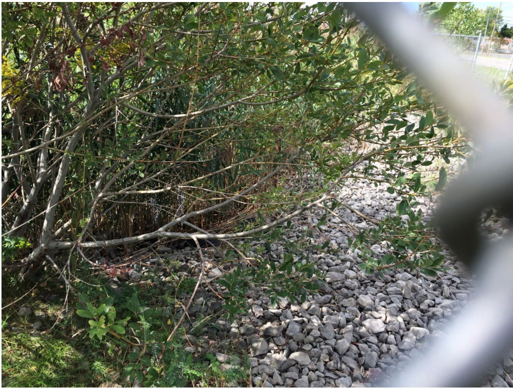
Photo 15 – Retention pond outlet pipes in northeast corner.
