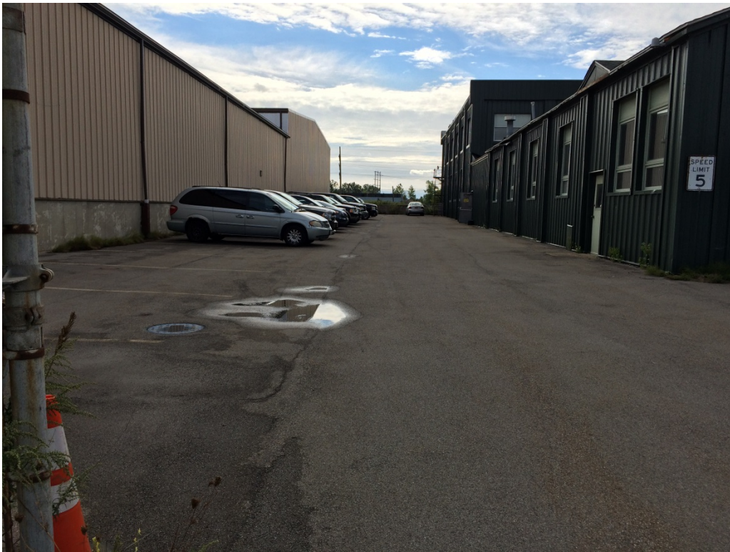
Photo 2 – Parking lot looking south.
