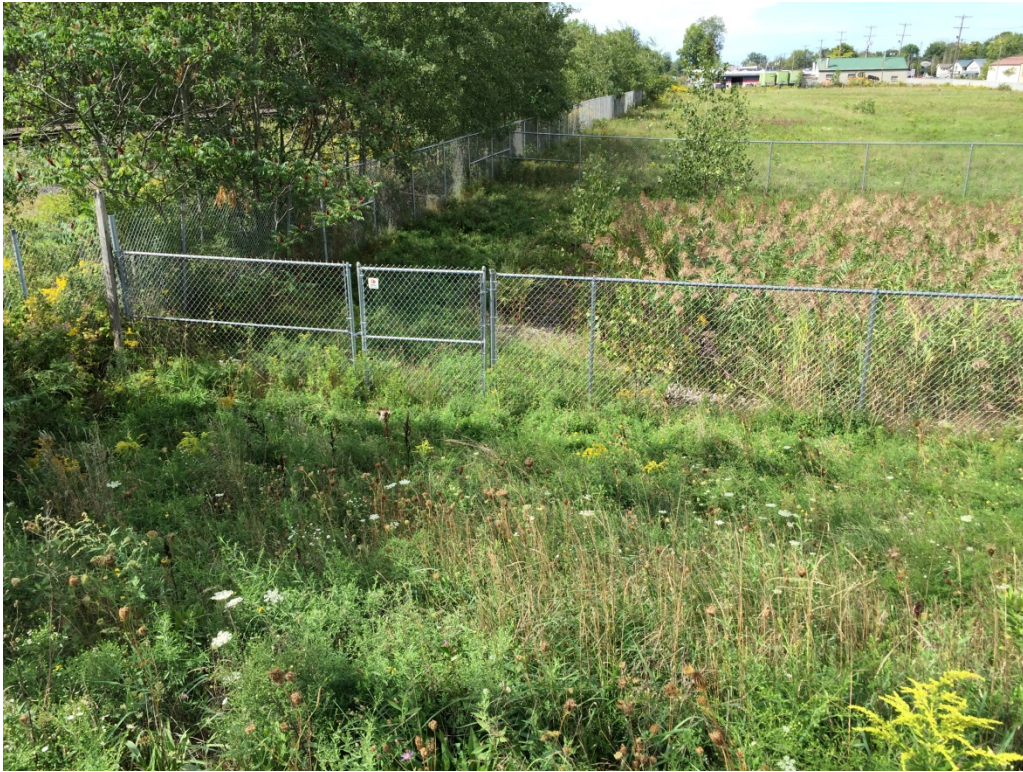
Photo 13 – South end of retention pond enclosure showing vegetation re-growth.
