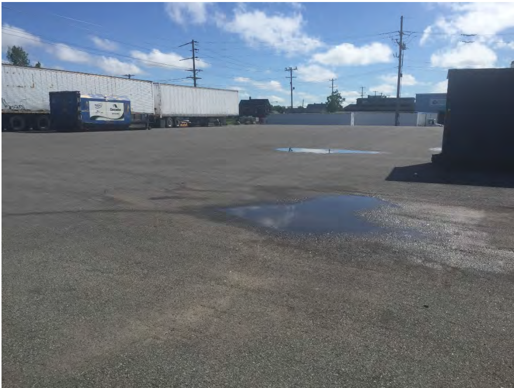
Photo 15 – GCL and Asphalt Cover System looking northeast across cap.
