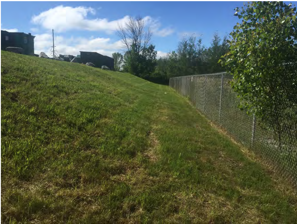
Photo 9 – GCL and Soil Cover System looking south along west slope.
