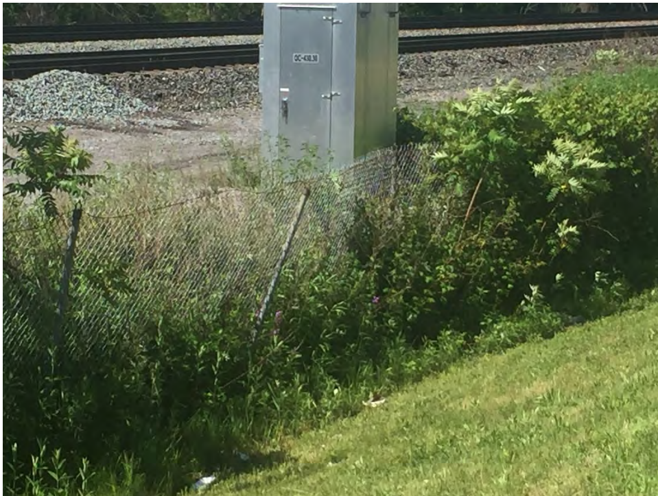
Photo 18 – Damaged fence along southern slope of GCL Area.
