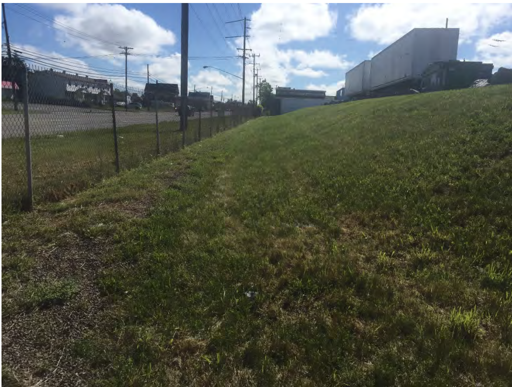
Photo 8 – GCL and Soil Cover System looking east along north slope.
