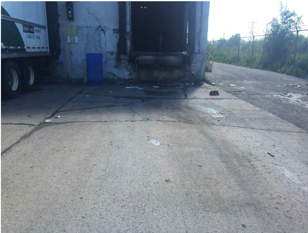
Photo 5 – Building Apron Concrete System (south end of building) looking east.
