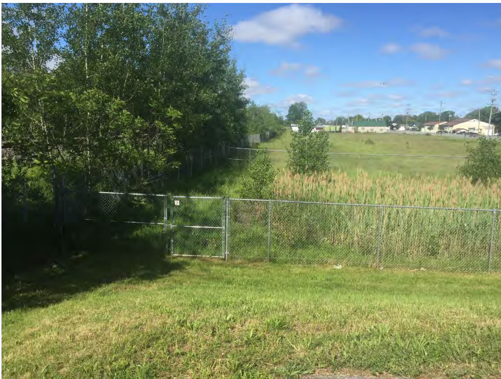
Photo 12 – South end of retention pond enclosure.
