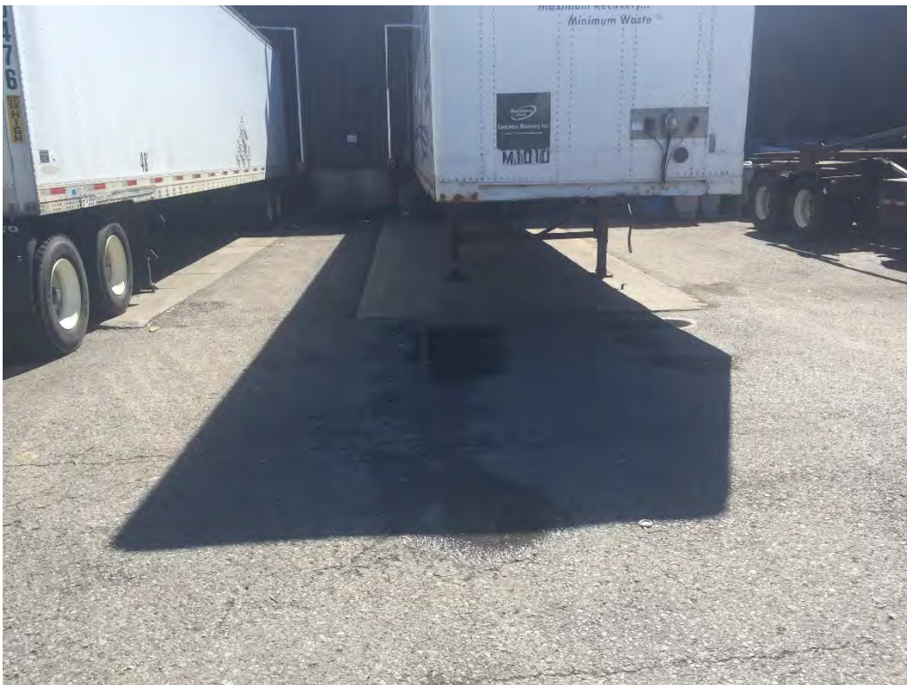
Photo 4 – Building Apron Concrete System (north end of building) looking east.
