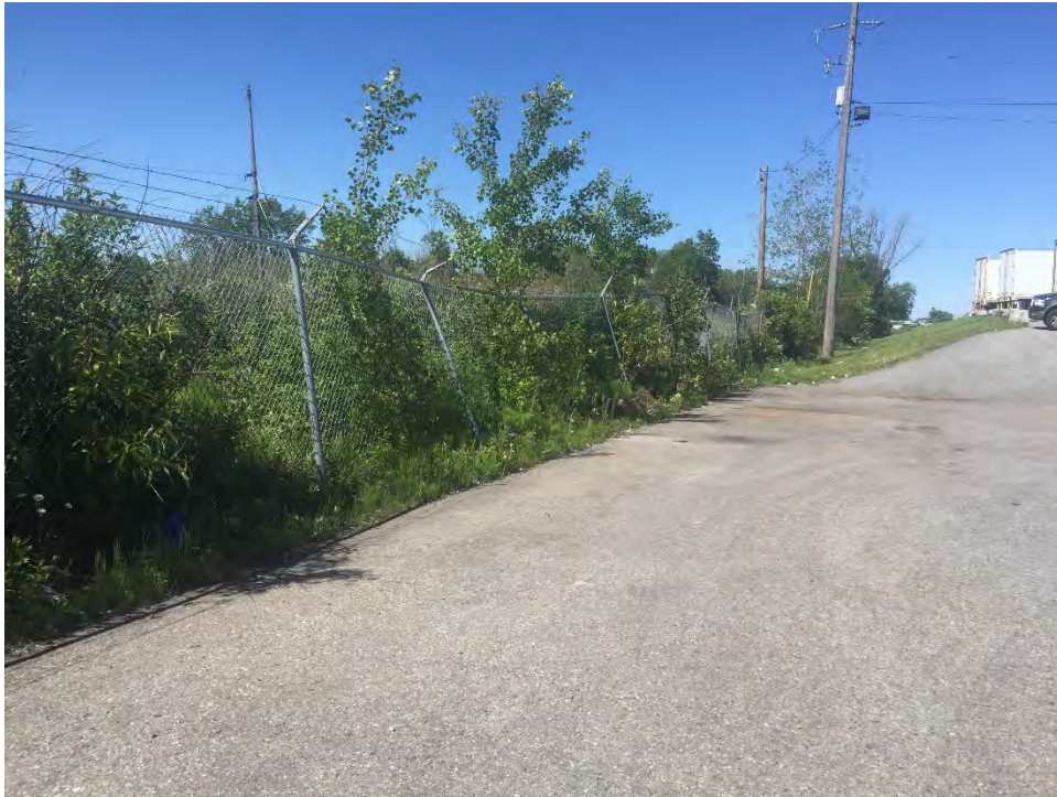
Photo 17 – Damaged fence along southern truck yard.
