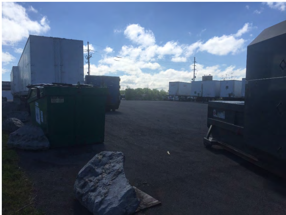
Photo 16 – GCL and Asphalt Cover System looking southeast across cap.
