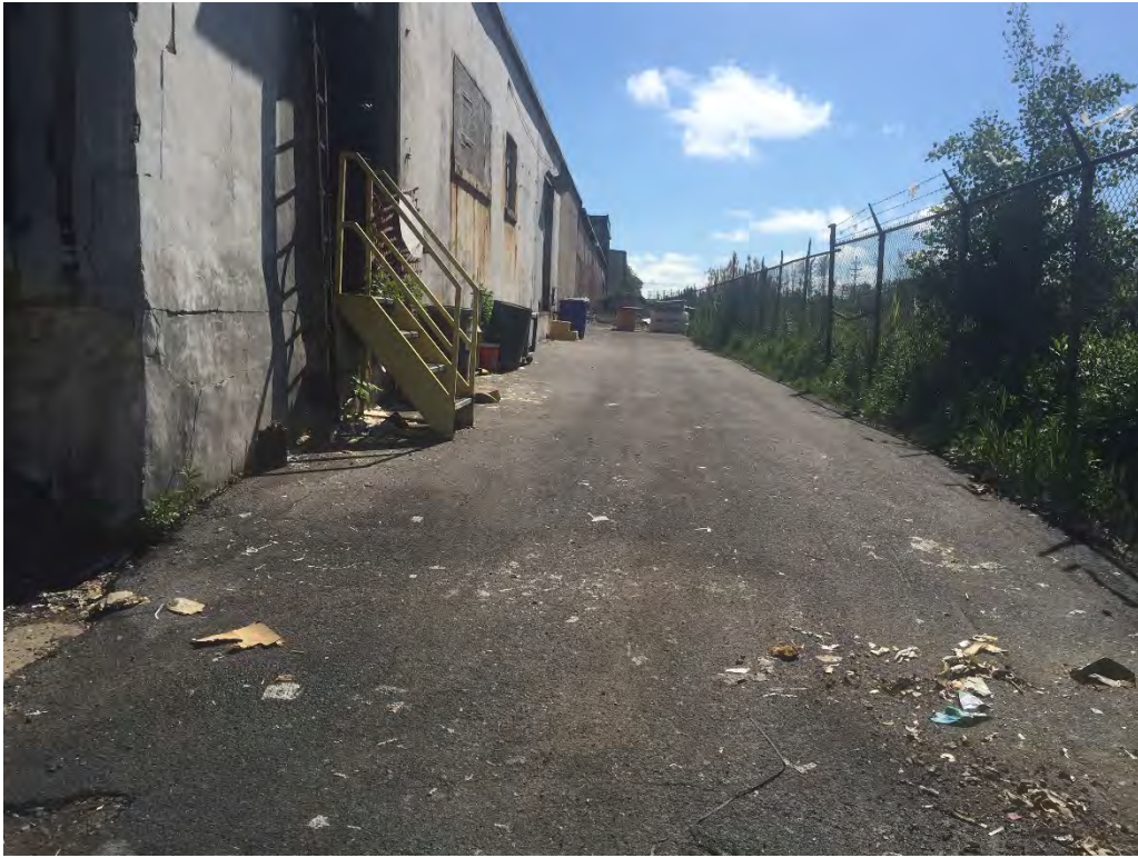
Photo 3 – Former rail siding looking east.
