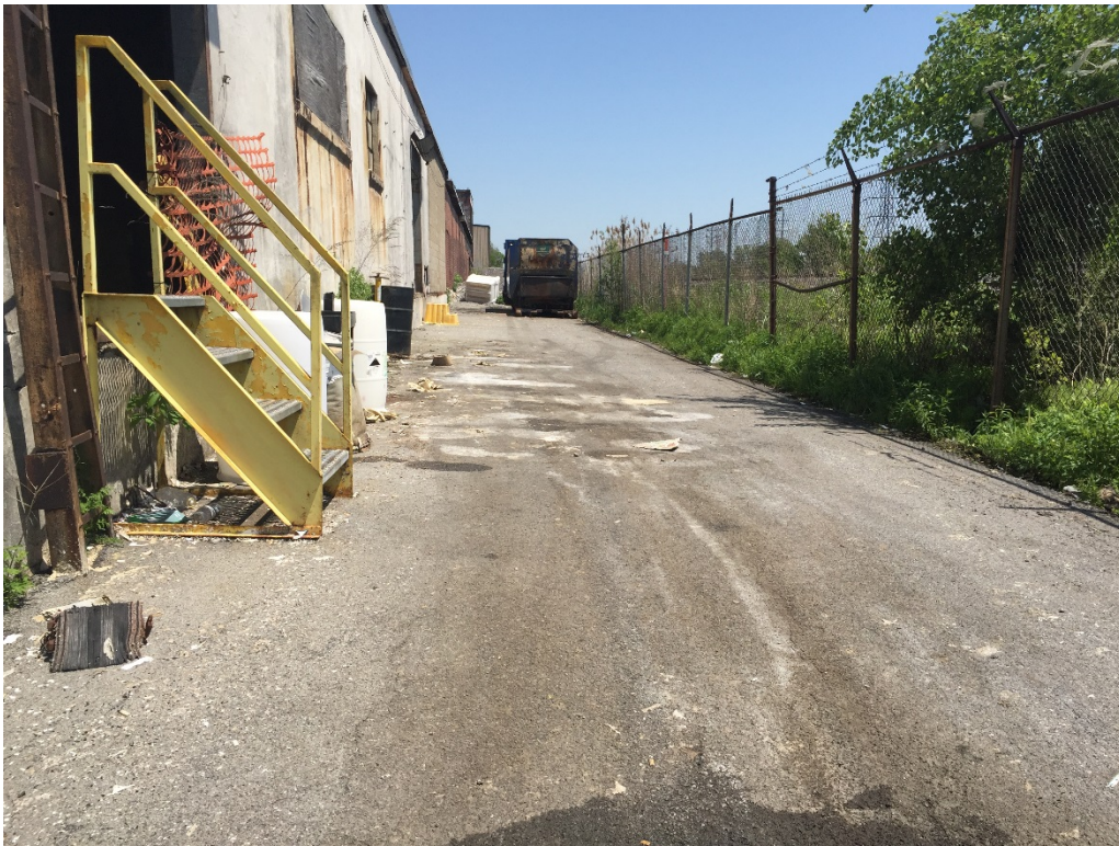
Photo 3 – Former rail siding looking east.
