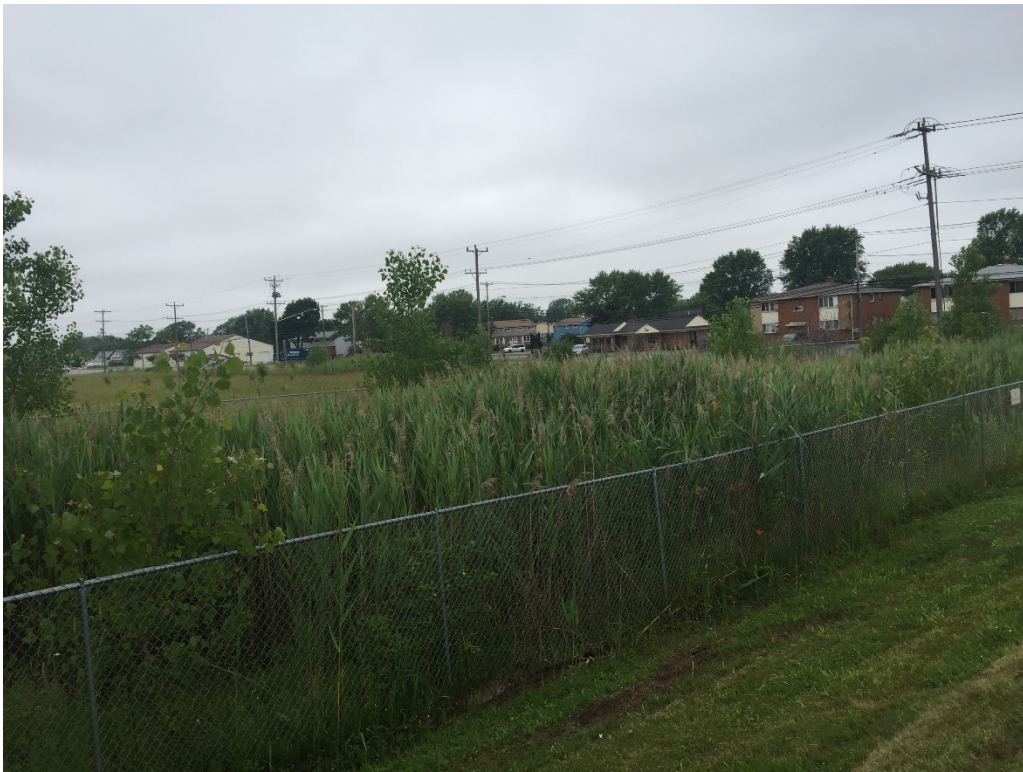
Photo 11 – Looking northwest across retention pond.
