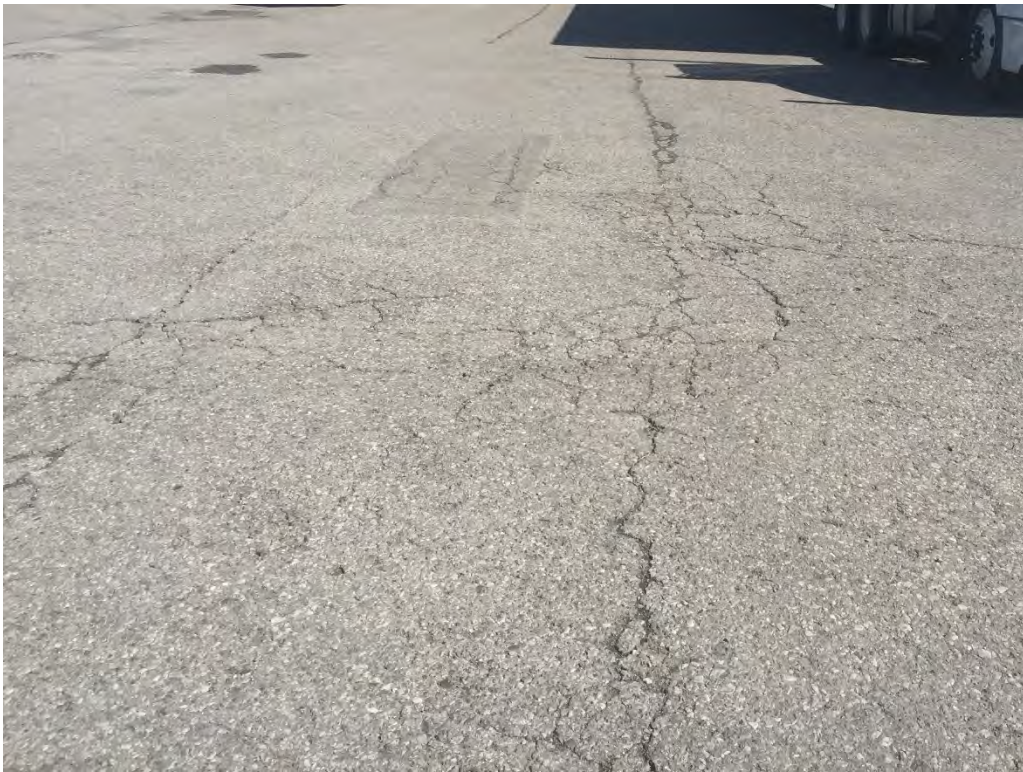
Photo 7 – Example of asphalt cracking in Trucking Yard.
