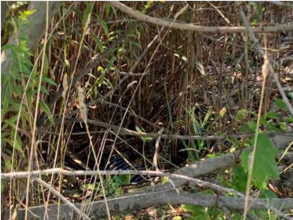
Photo 16 – Looking over outlet pipes of pond.
