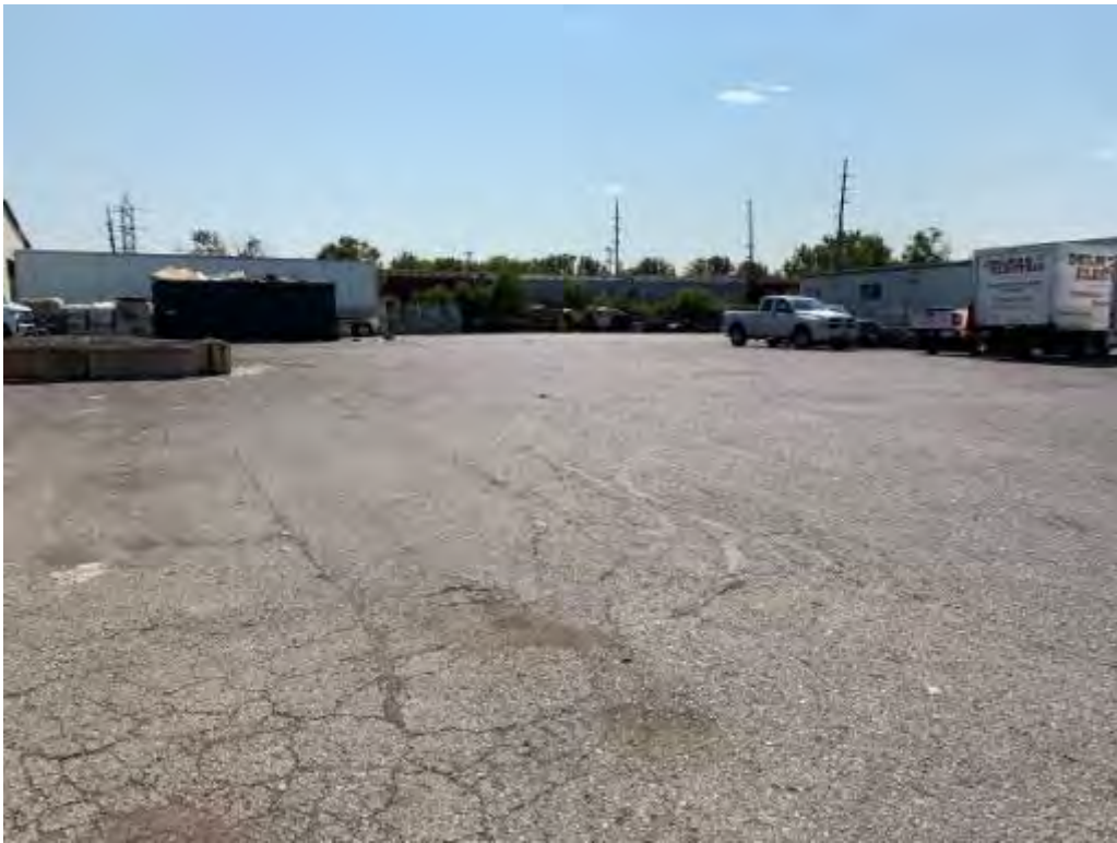
Photo 9 – Trucking yard looking south-southwest.
