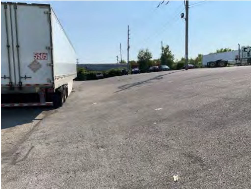
Photo 17 – Looking south over east slope of GCL/asphalt cover.
