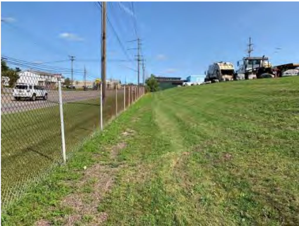
Photo 14 – GCL and Soil Cover System looking east along north slope.
