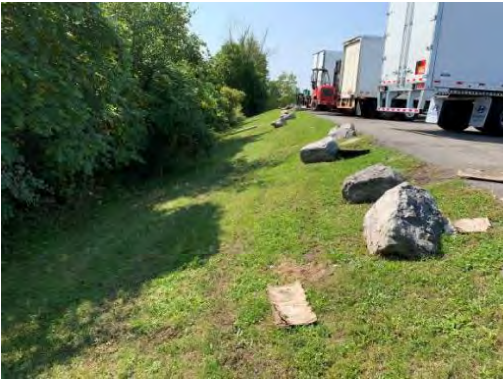
Photo 11 – GCL and Soil Cover System looking west along south slope.
