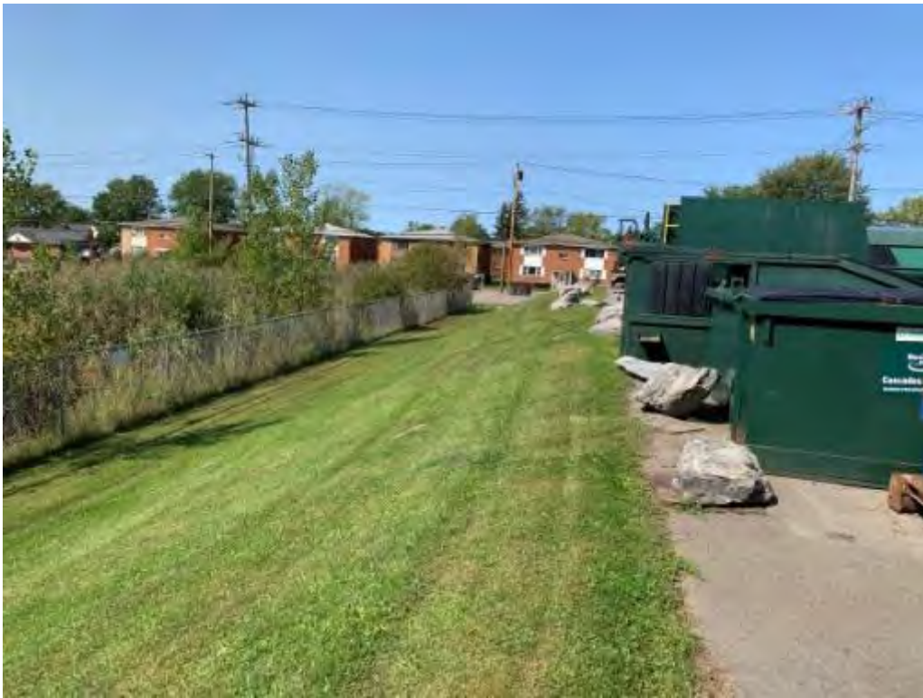
Photo 13 – GCL and Soil Cover System looking north along west slope.
