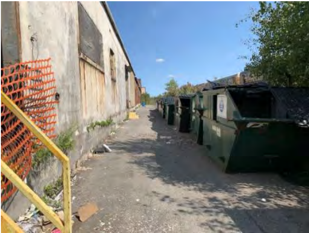
Photo 3 – Former rail siding looking east.
