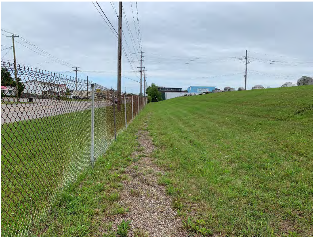
Photo 12 – GCL and Soil Cover System looking east along north slope.
