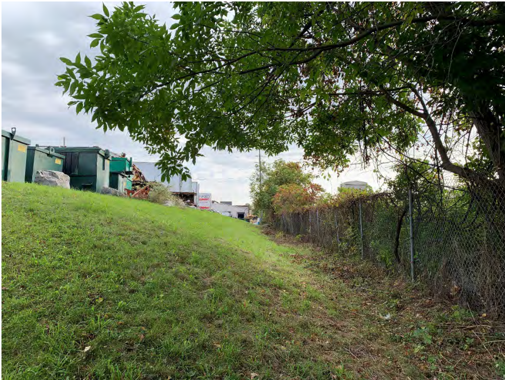
Photo 10 – GCL and Soil Cover System looking east along south slope.
