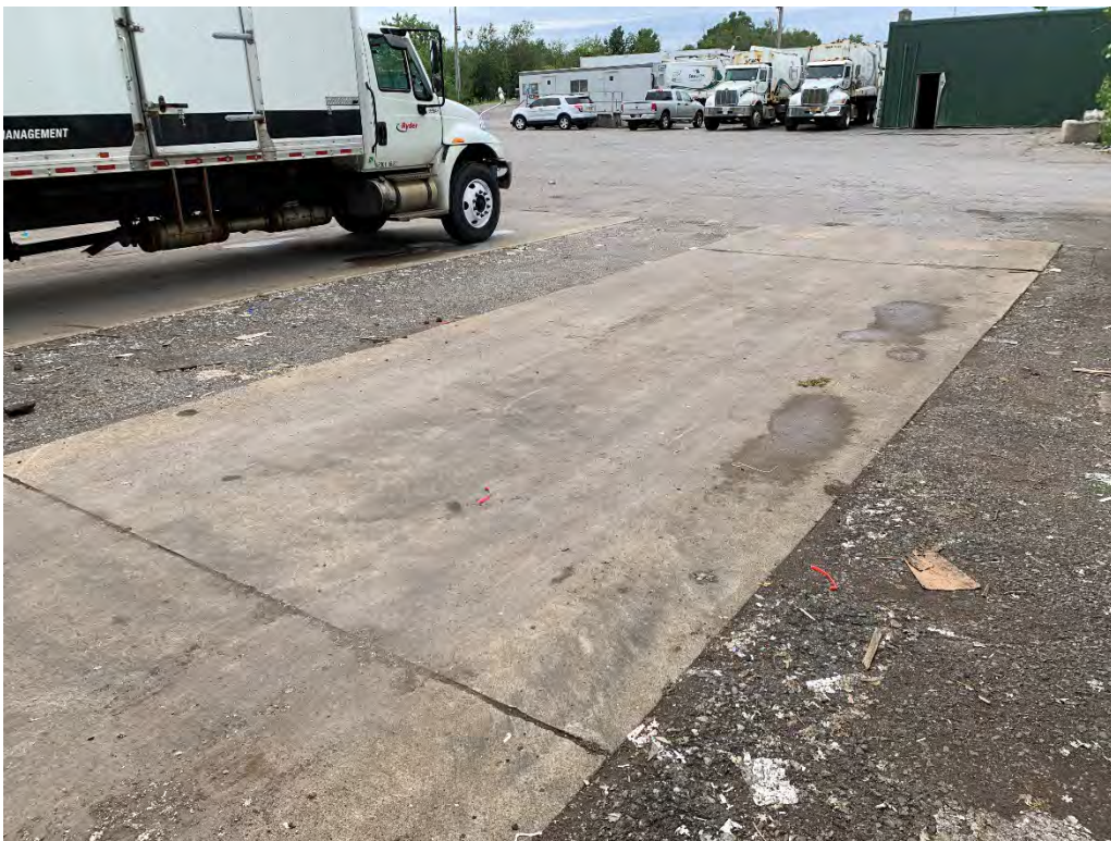
Photo 6 – North concrete aprons looking west-southwest.
