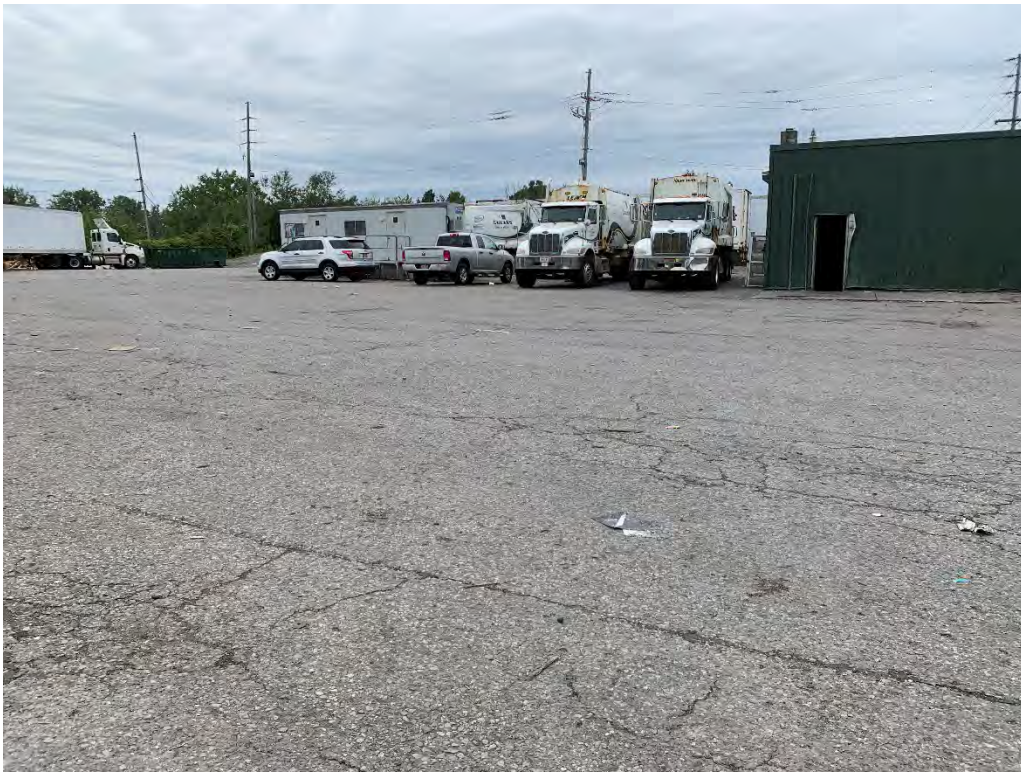
Photo 7 – Trucking yard looking southwest.
