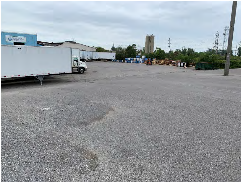
Photo 16 – Looking southeast across slope of GCL/asphalt cover toward trucking yard.
