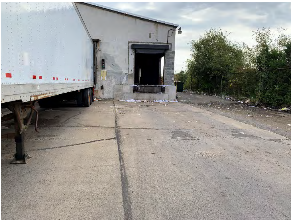
Photo 4 – South concrete apron looking east.
