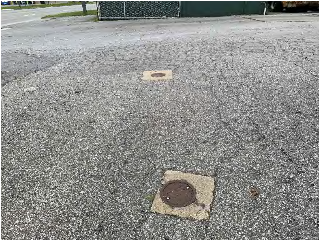
Photo 17 – Looking east across trucking yard entrance.
