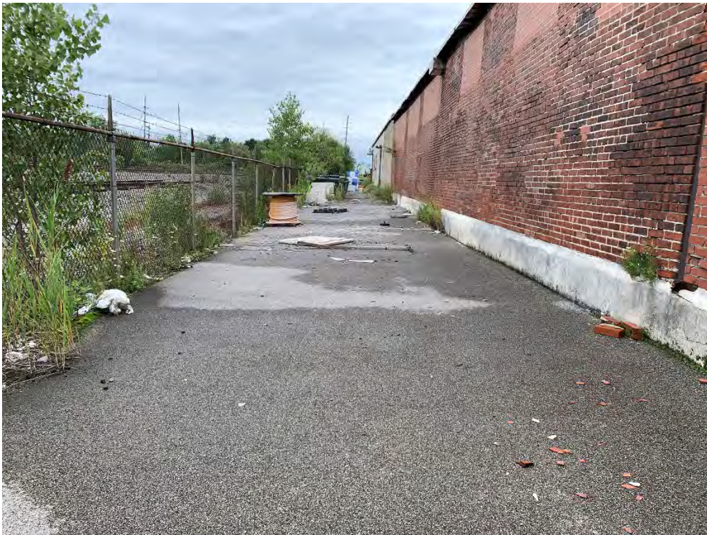
Photo 3 – Former rail siding looking west.
