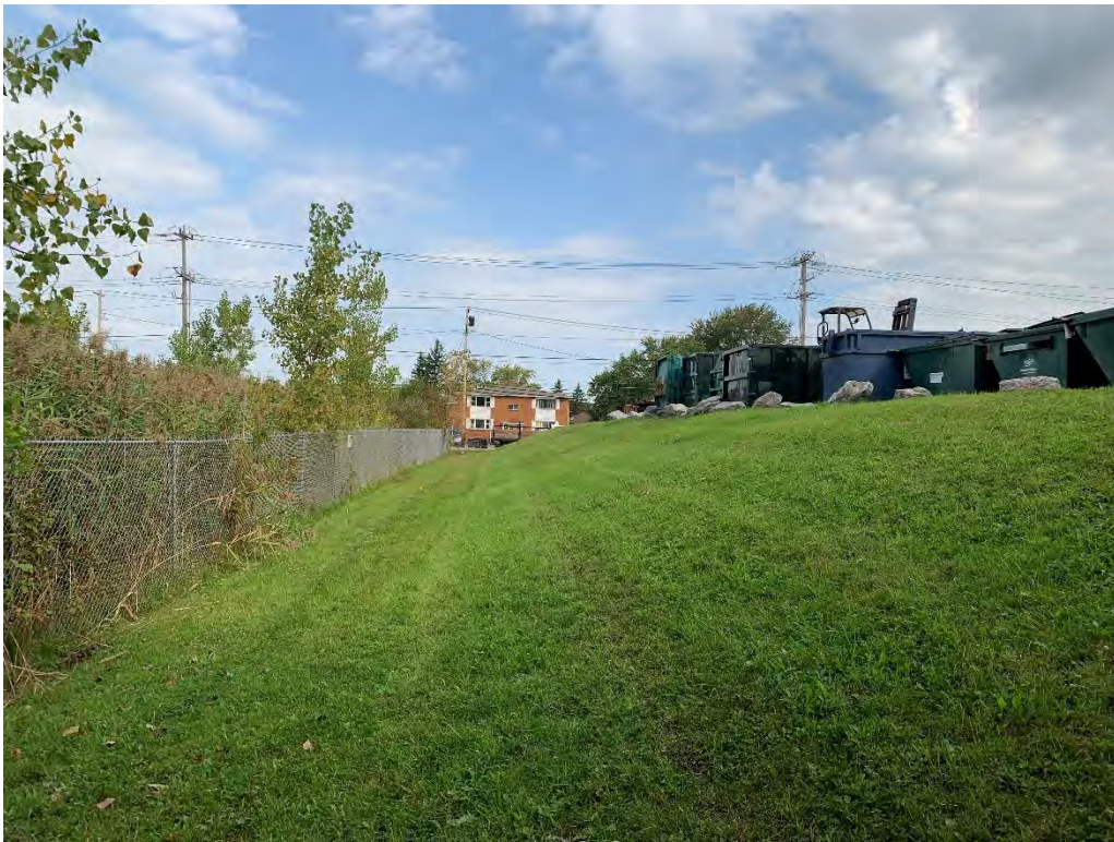
Photo 11 – GCL and Soil Cover System looking north along west slope.
