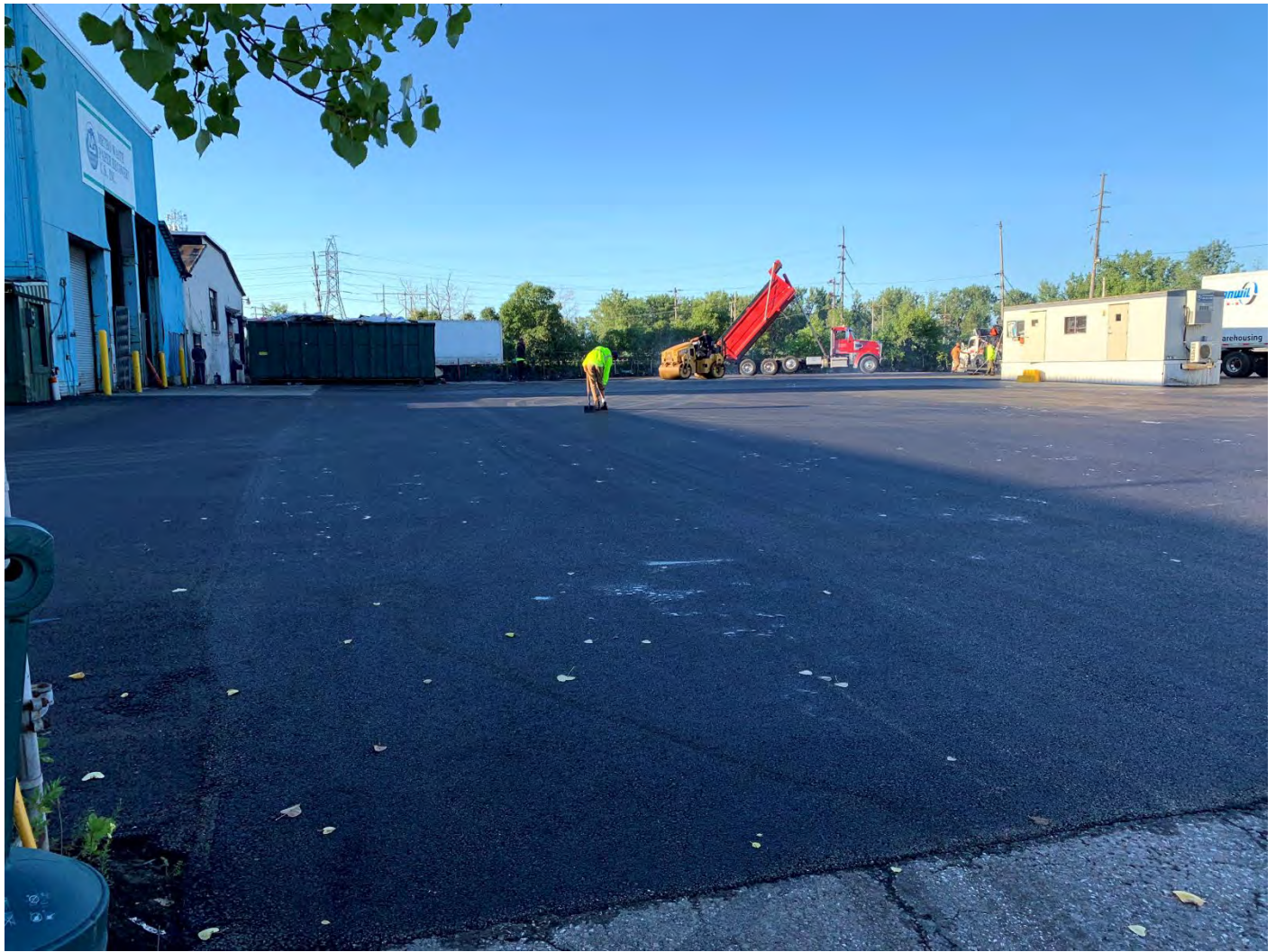
Photo 19 – Looking south across trucking yard at the resurfacing of the trucking yard
