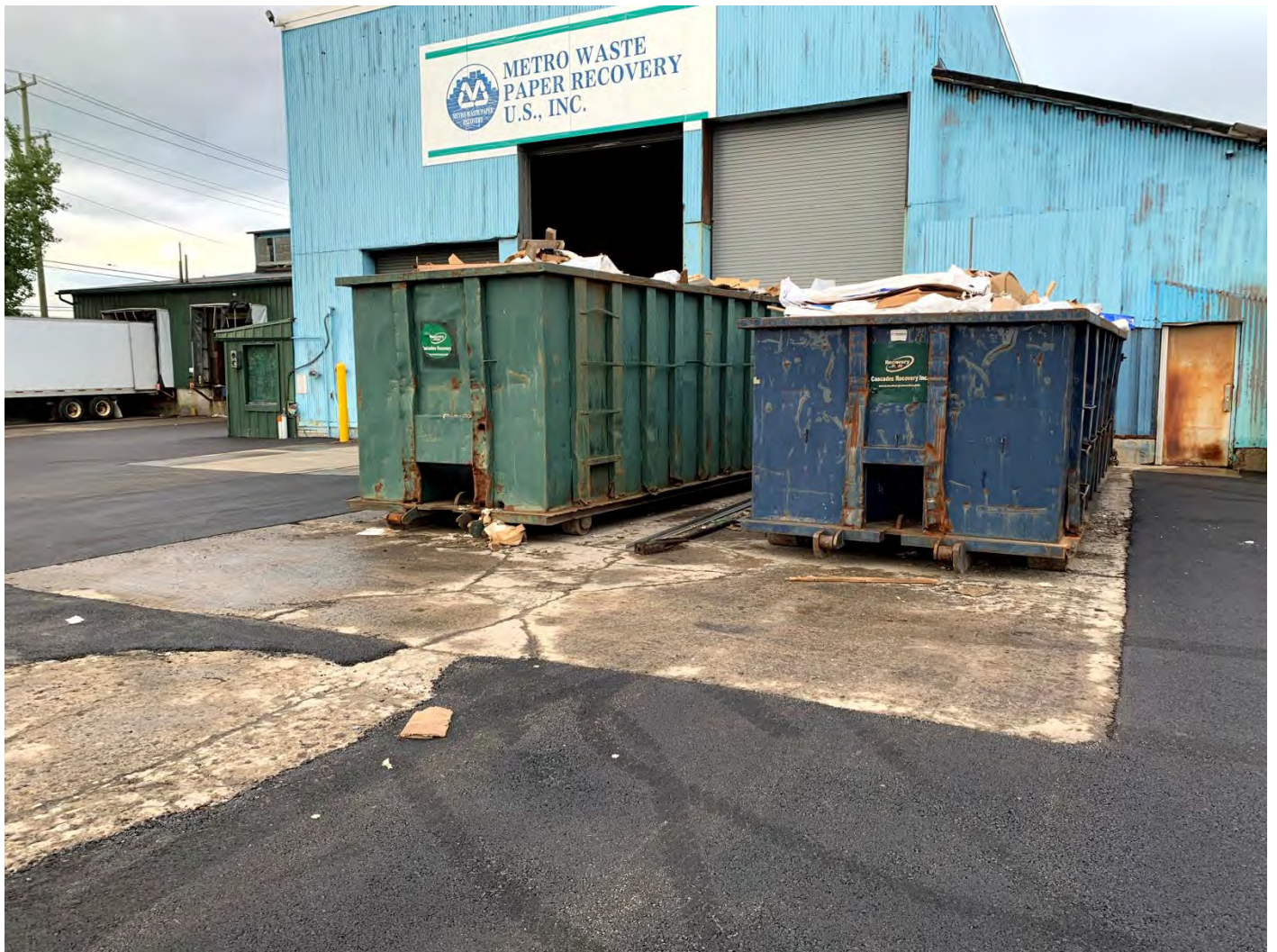
Photo 5 – Building Apron Concrete System (central portion) looking east-northeast. Surface cracks are sealed.
