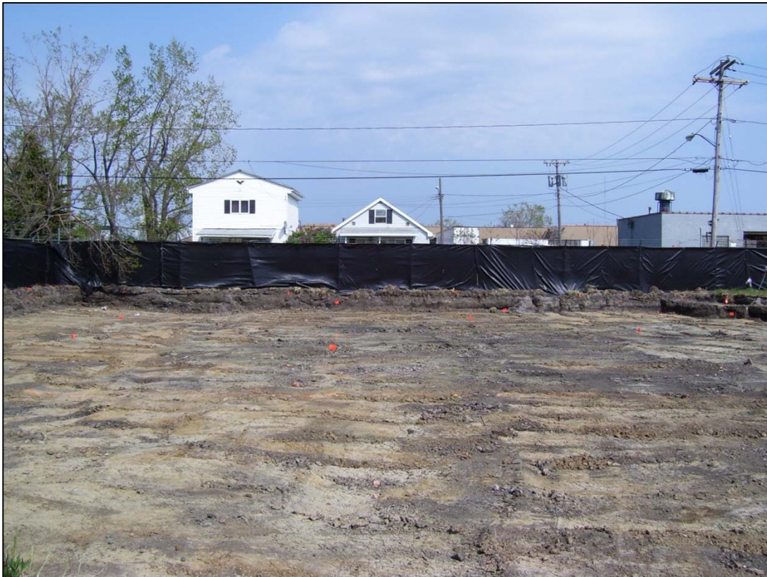
Photograph 5: Parcel #5 – Facing E, NE corner of excavation, 2'-3', 5/15/07
