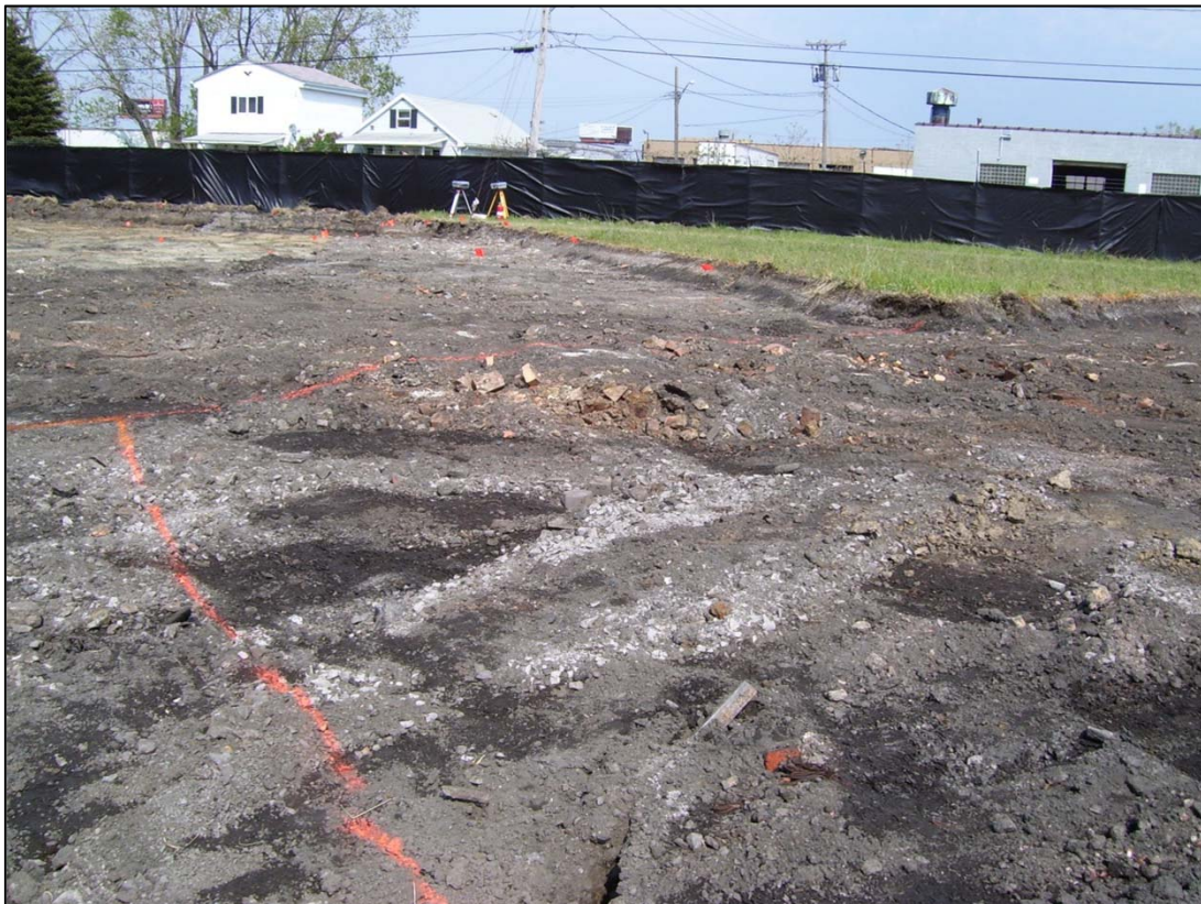
Photograph 8: Parcel #5 – Facing E, central area of excavation, 0-1', 5/15/07
