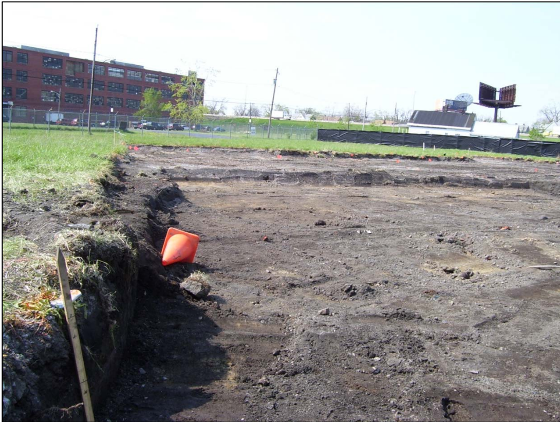
Photograph 15: Parcel #5 – Facing NW, southern area of excavation, 1'-2' and 0-1', 5/15/07
