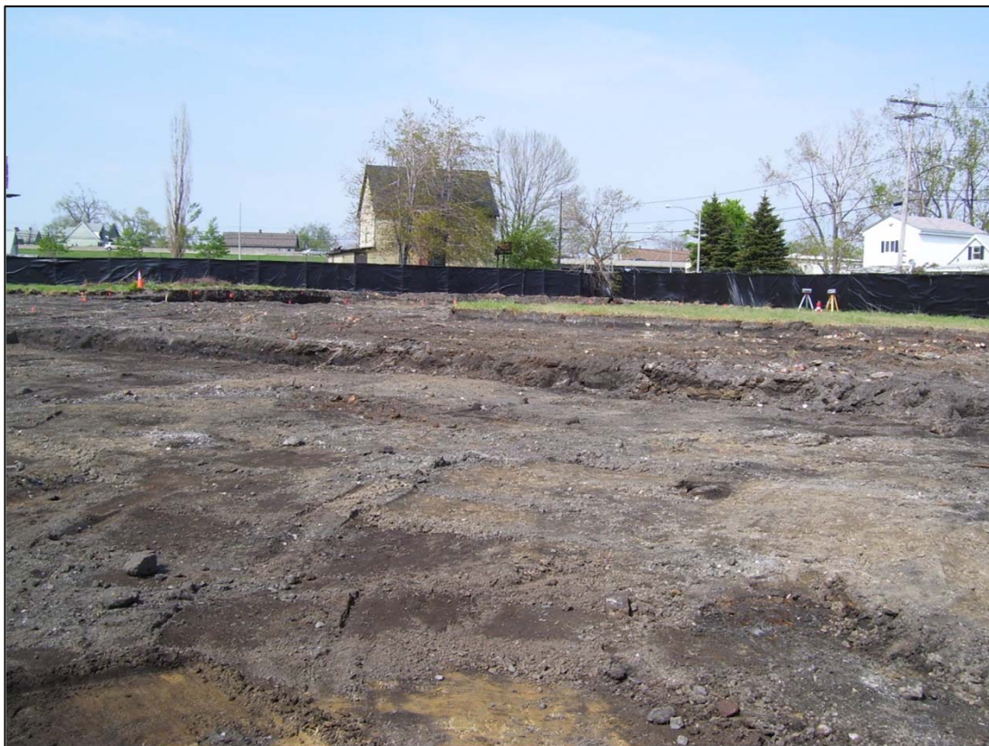
Photograph 14: Parcel #5 – Facing NE, southern area of excavation, 1'-2' and 0-1', 5/15/07
