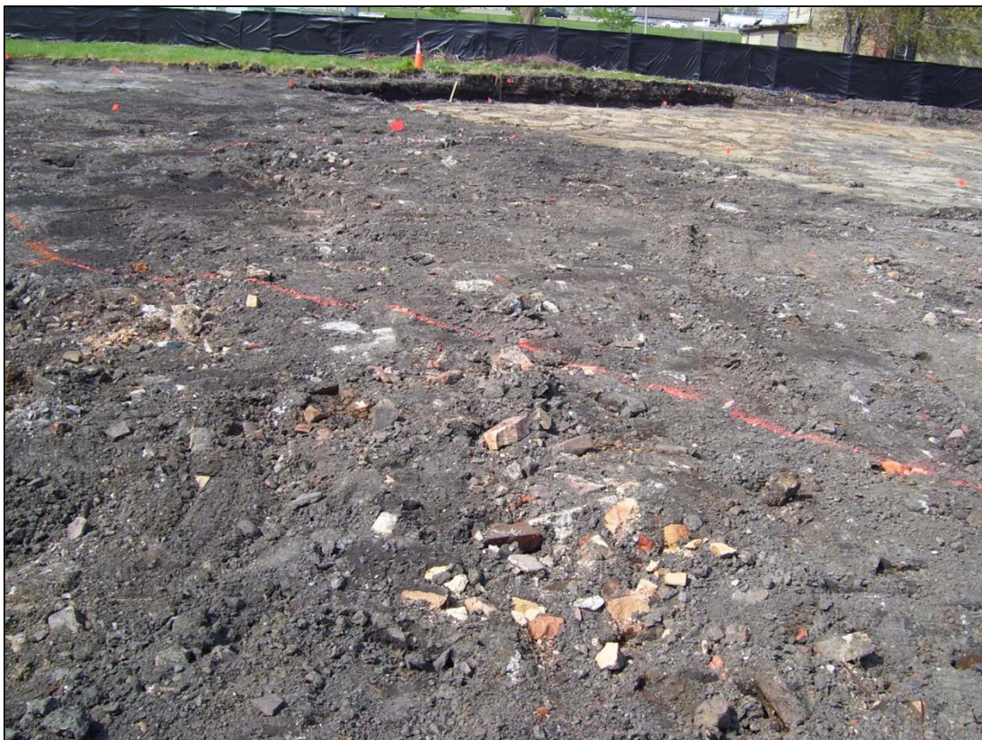
Photograph 12: Parcel #5 – Facing N, central area of excavation, 0-1' and 2'-3', 5/15/07
