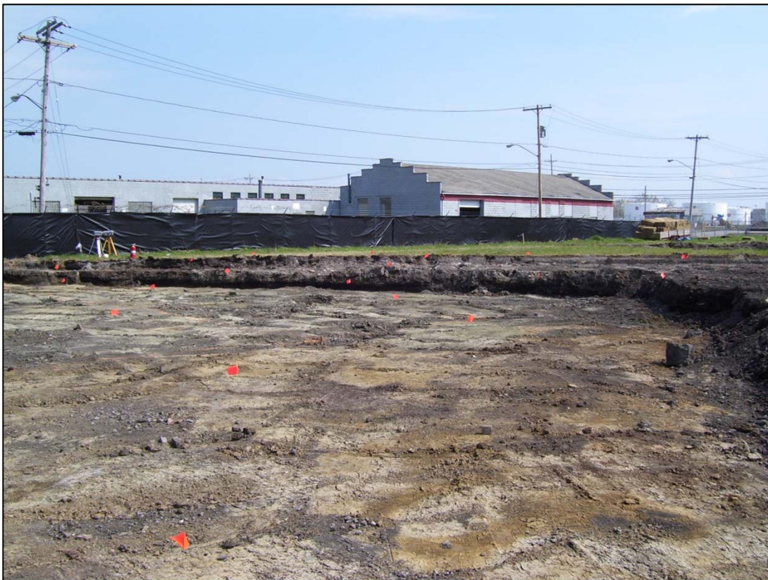
Photograph 6: Parcel #5 – Facing SE, NE corner of excavation, 2'-3', 5/15/07
