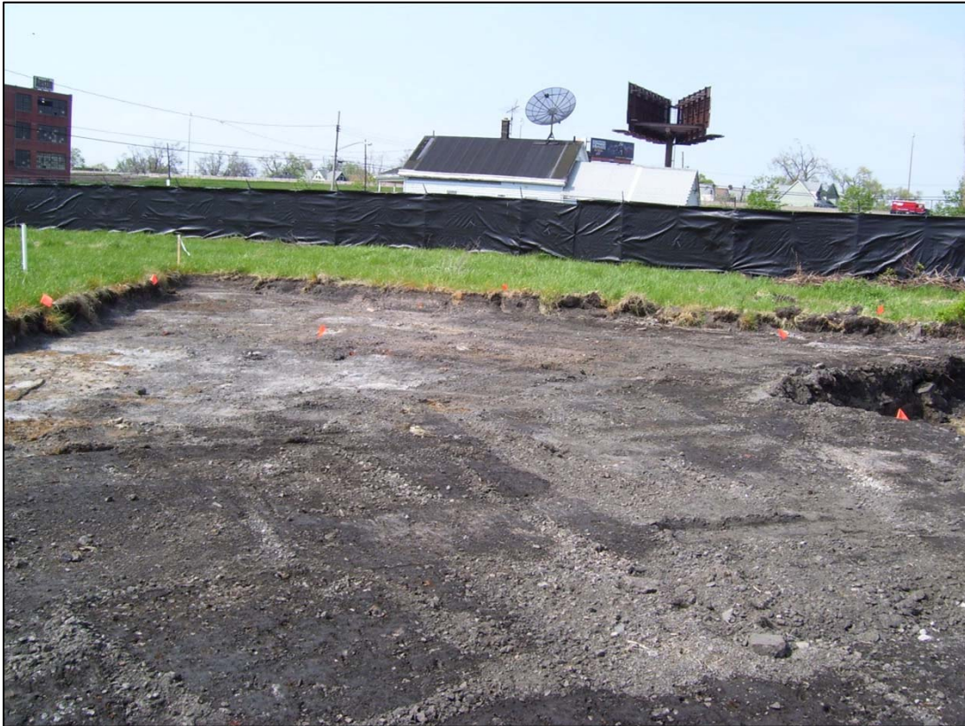
Photograph 7: Parcel #5 – Facing NW, NW corner of excavation, 0-1', 5/15/07
