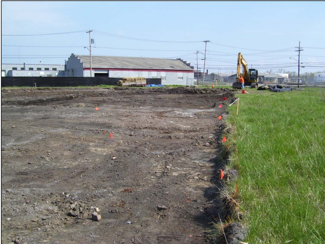
Photograph 11: Parcel #5 – Facing SE, central area of excavation, 0-1', 5/15/07
