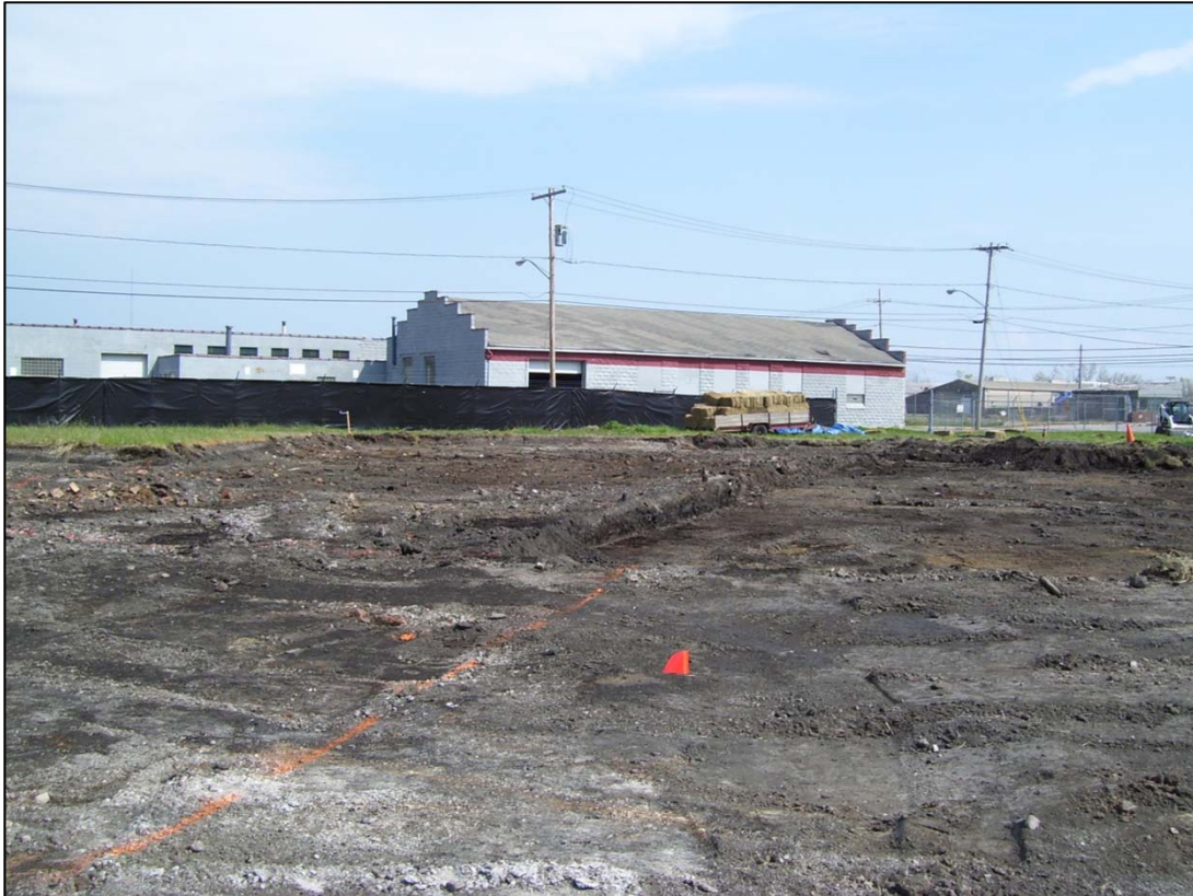
Photograph 9: Parcel #5 – Facing SE, central and southern areas of excavation, 0-1' and 1'-2', 5/15/07
