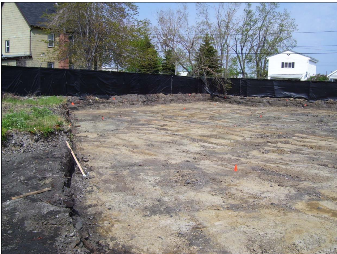
Photograph 4: Parcel #5 – Facing NE, NE corner of excavation, 2'-3', 5/15/07
