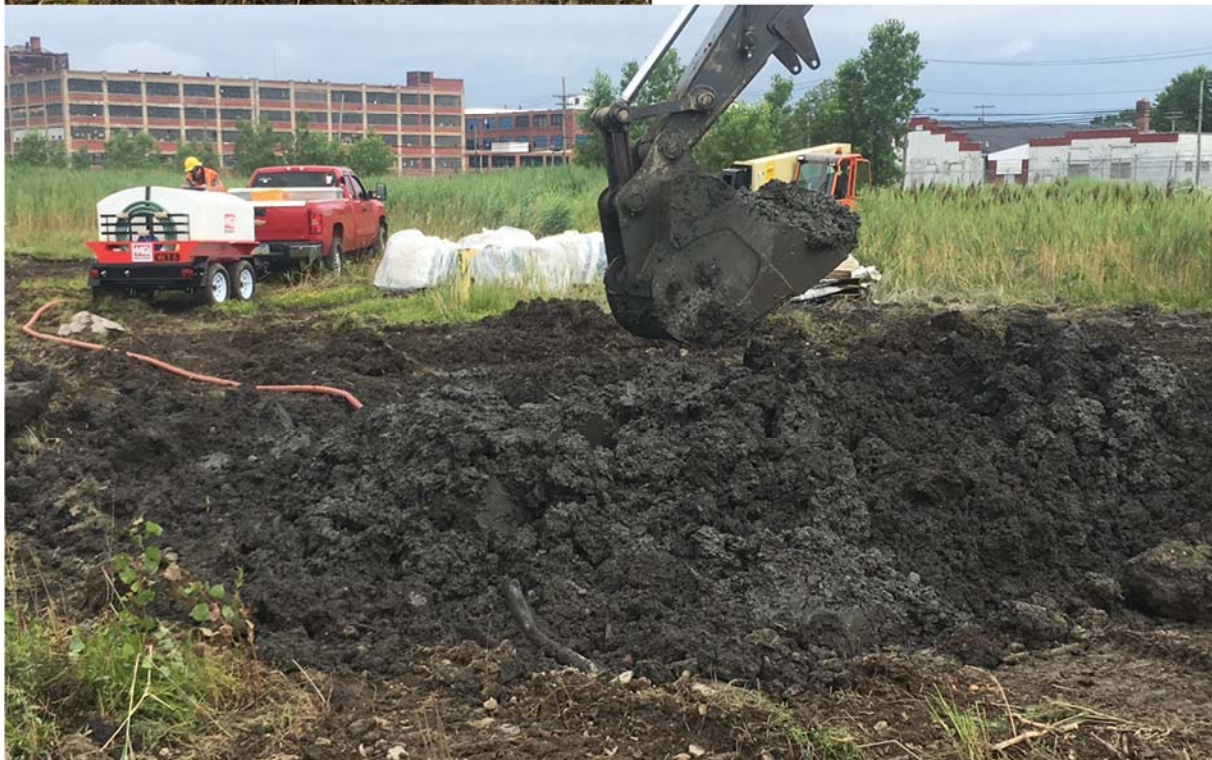
Photograph 6 – Addition of water at Test Cell GCM 4-4 after reagent had already been mixed
