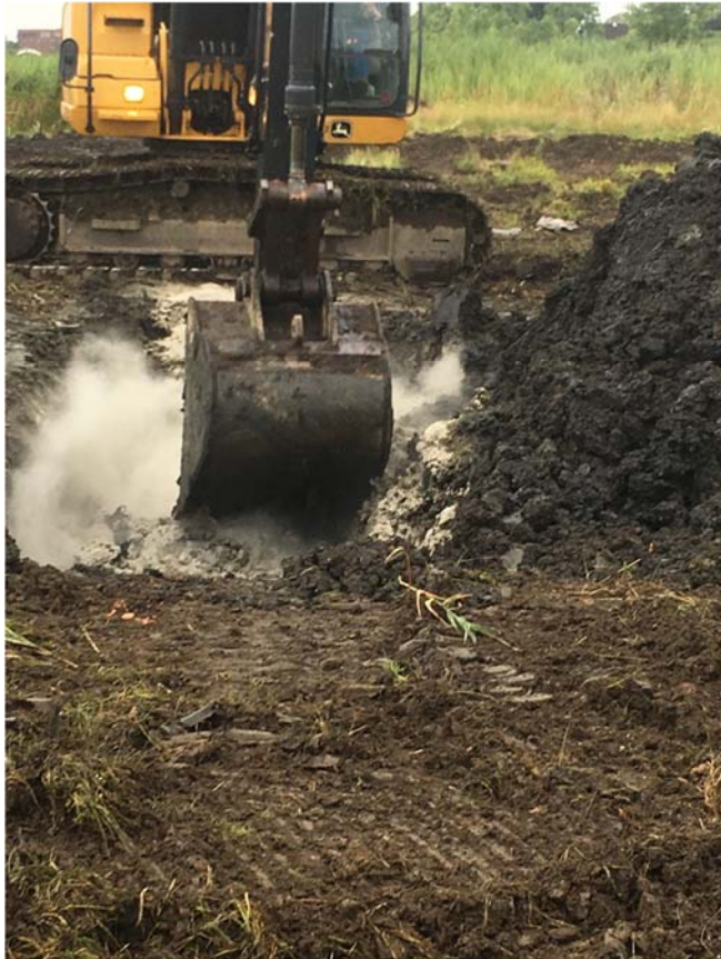
Photograph 5 – Dry mixing of reagent at Test Cell GCM 4-4.
