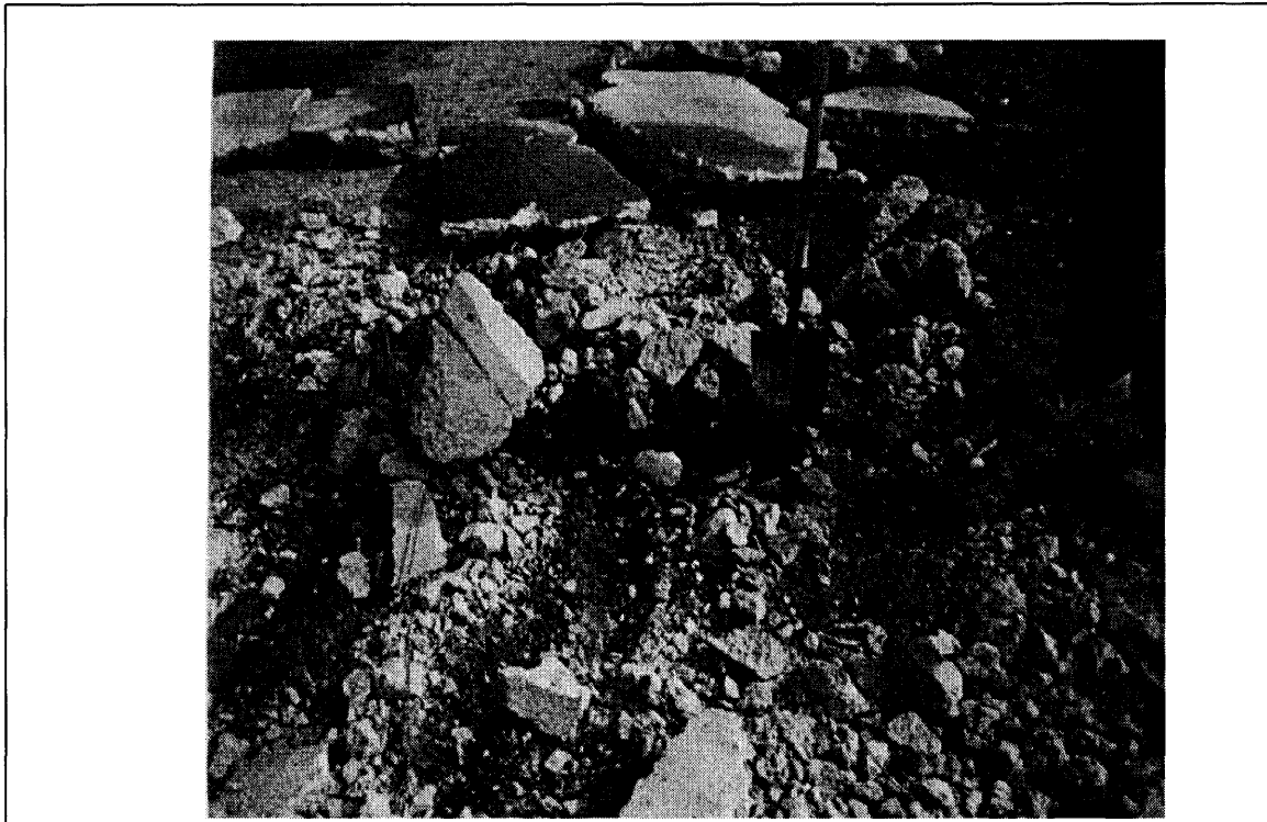
View of TP-02. Picture shows soil conditions just below concrete.
