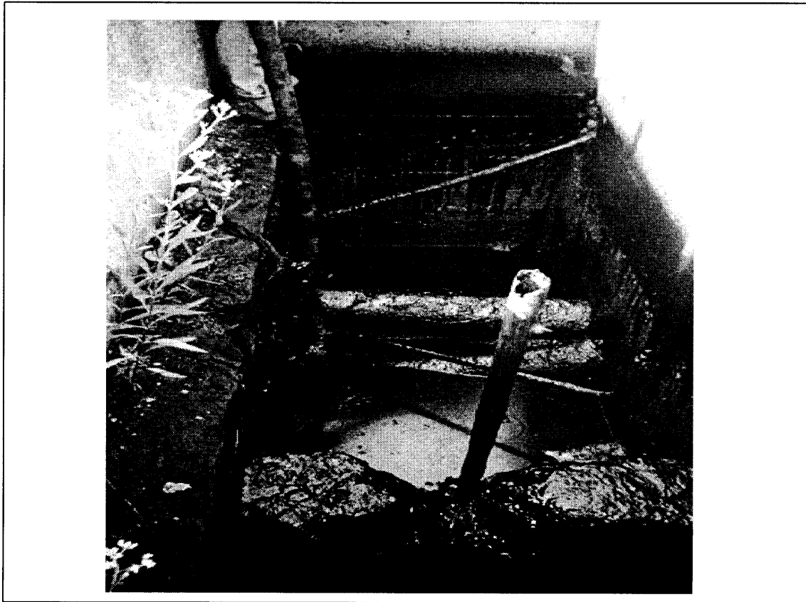
View from south of pipes at TP-09.
