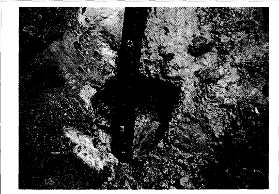
View of soil below concrete at TP-02. Soil is stained and product noted.
