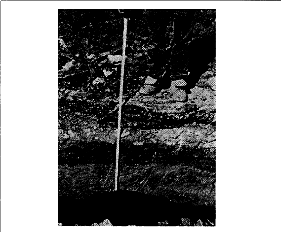
View of TP-06. Bottom of excavation approximately 15 feet bls.
