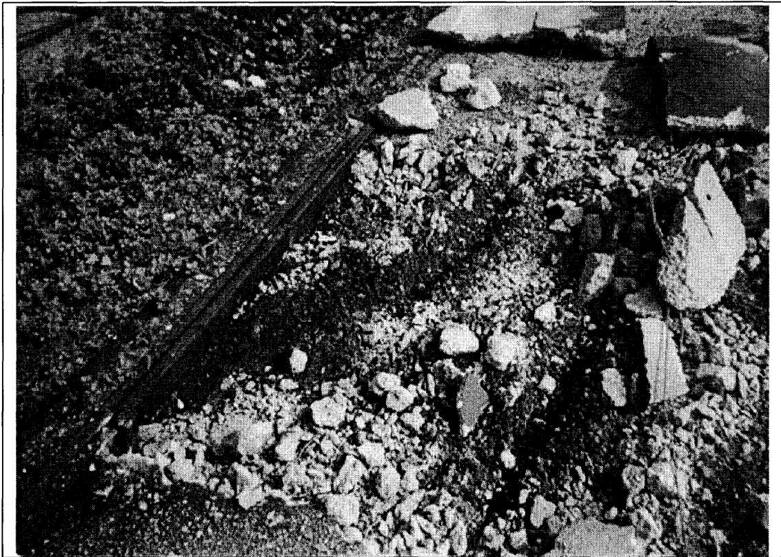
View of TP-01. Picture shows soil conditions below concrete. No visible impacts noted.
