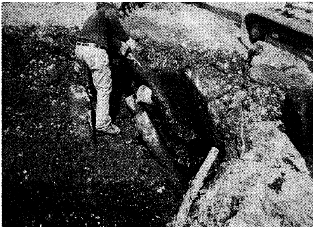
View of TP-10 of pipes entering from the east jutting upwards. The two(2) pipes in foreground are 6" diameter, and one(1) 10" diameter pipe in background. All pipes appear to end at this point. A 3-inch pipe crossing the west side of the trench, aligned north-south cannot be observed.
