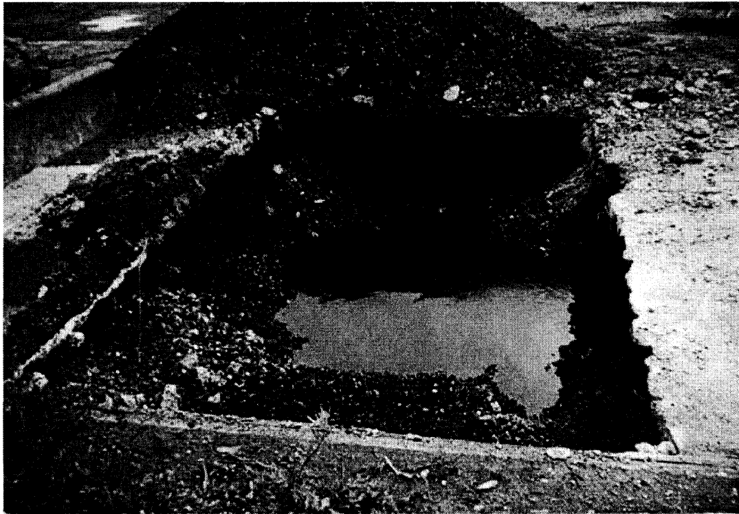
View from the west of TP-01. Shows depth to water, no appearance of petroleum impact.
