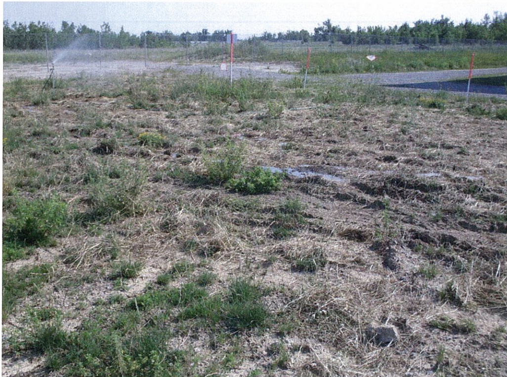
Rolled and re-seeded vehicle ruts.
