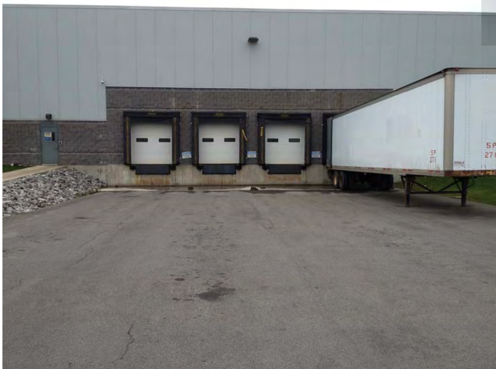
November 2012 – View of loading dock on the northeastern corner of the facility.
