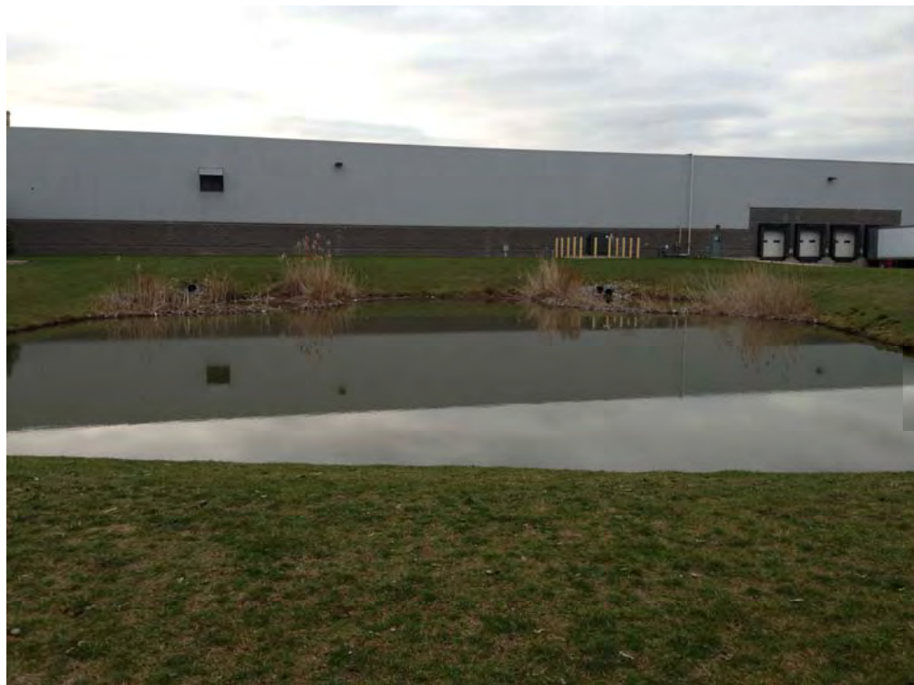
November 2012 – View of retention pond and loading dock from eastern outlet.
