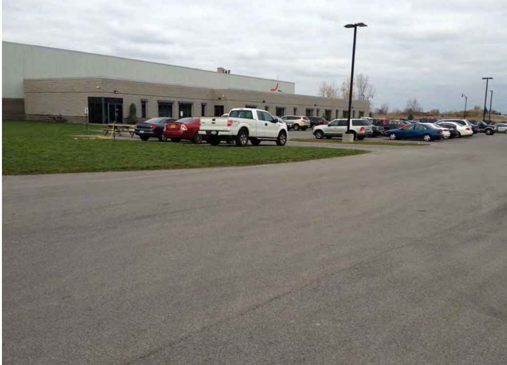
November 2012 – View of asphalt drive and parking area on southern side of the facility.
