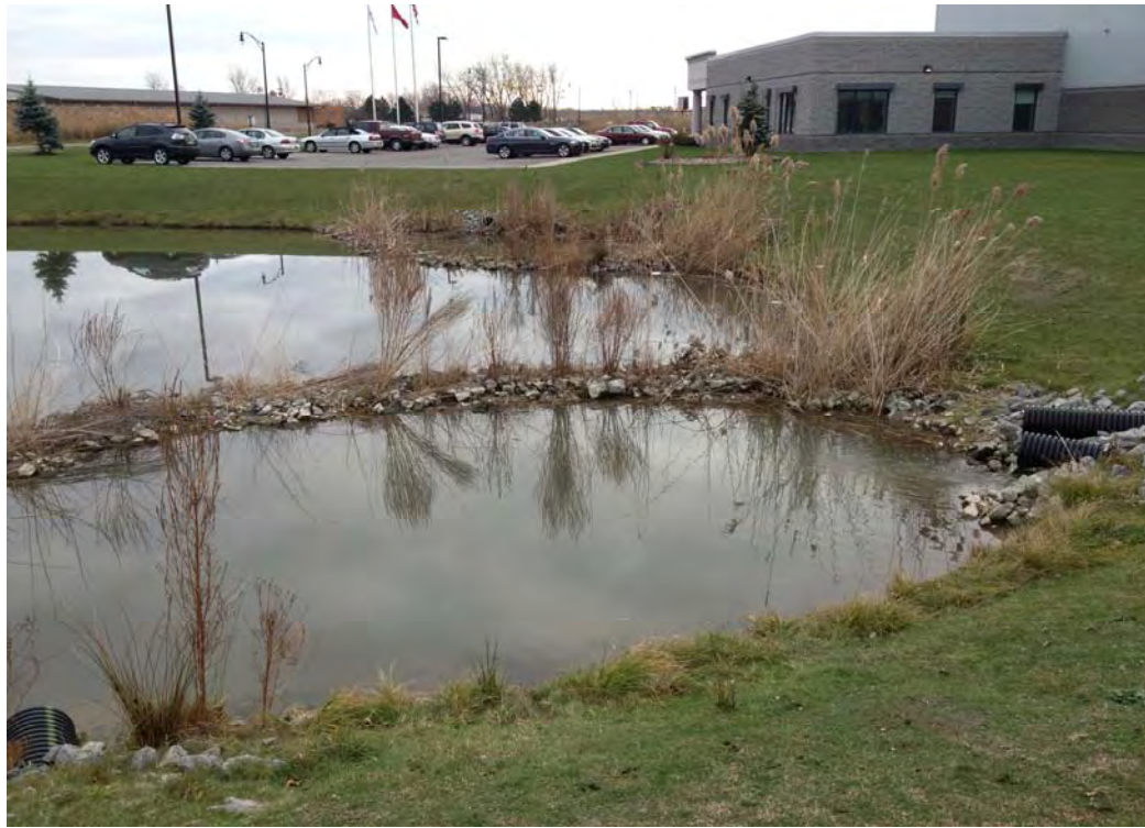
November 2012 – View of retention pond on northeastern corner of the property (northwestern portion of pond).
