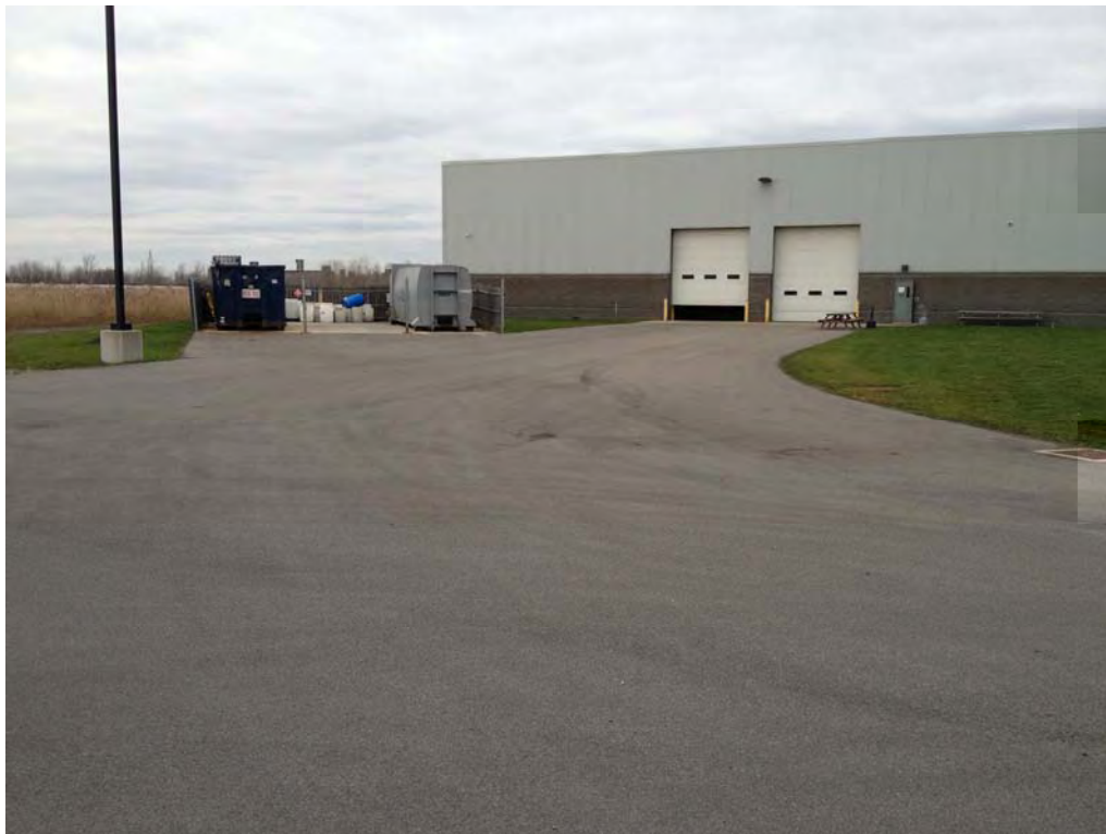
November 2012 – View of asphalt parking area and loading dock on south side of facility.
