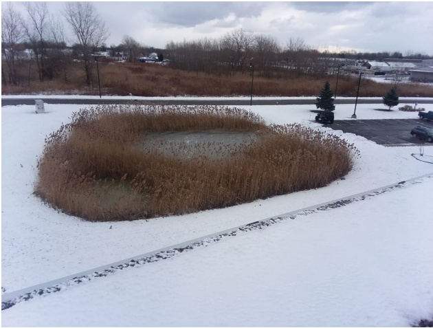
Photo 13: Stormwater pond in December 2019.
