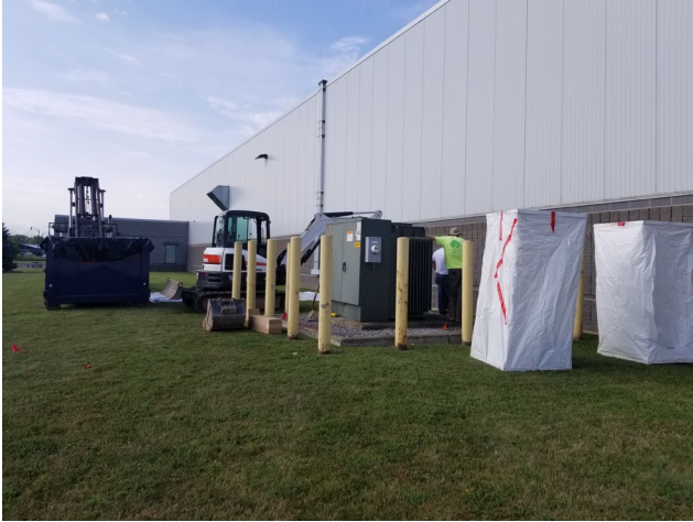
Photo 1: Area of July-August 2019 utility trench excavation.
