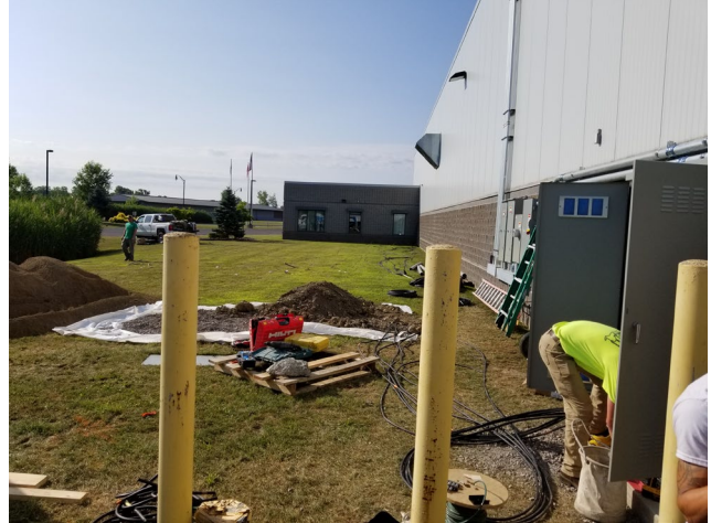
Photo 2: Area of July-August 2019 utility trench excavation
