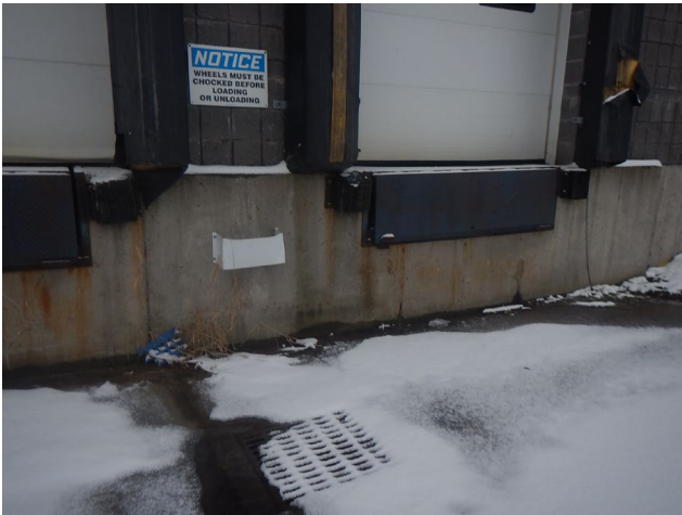
Photo 9: Catch basin in northeast loading dock area
