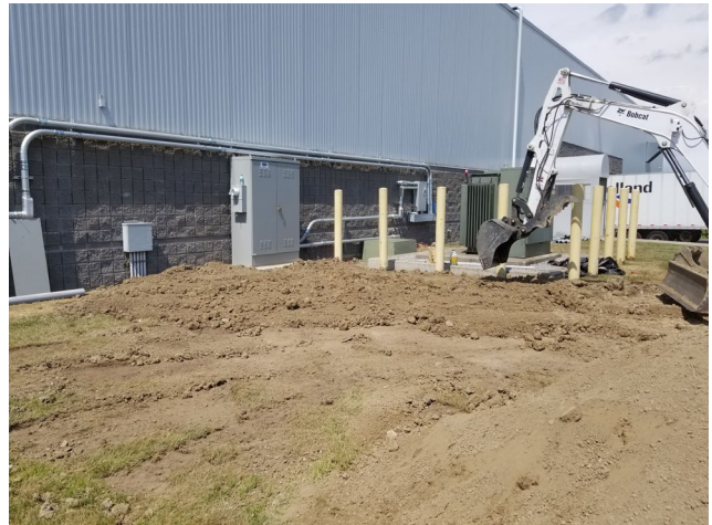
Photo 4: Utility trench excavation backfilling
