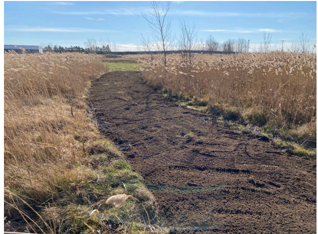
Photo 10: Rutting repair with imported topsoil, December 2020.
