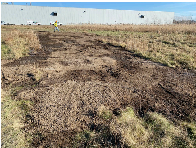
Photo 11: Rutting repair with imported topsoil, December 2020.
