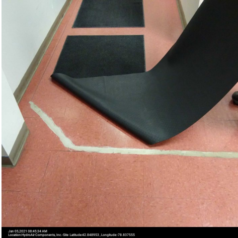
Photo 1: Representative office floor crack repair with hydraulic cement.
