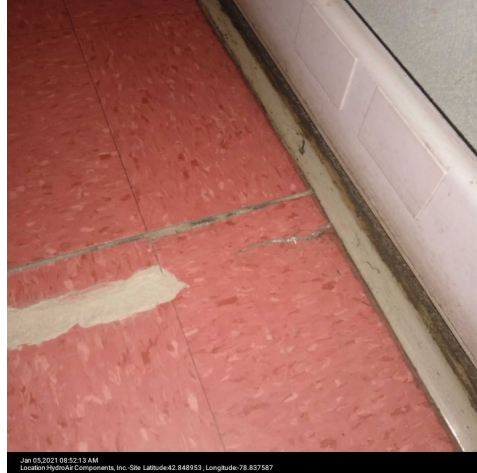
Photo 2: Small floor cracks extending below carpeted floor coverings in Site office.
