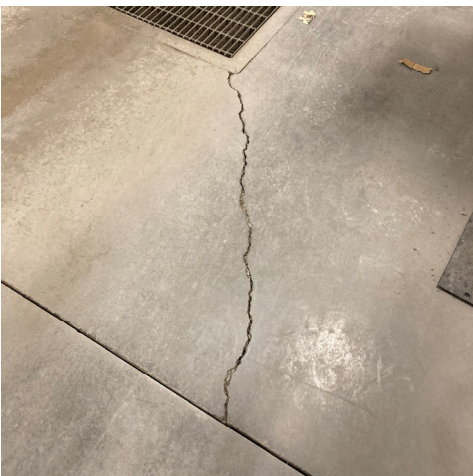
Photo 11: Minor floor cracking in manufacturing space.
