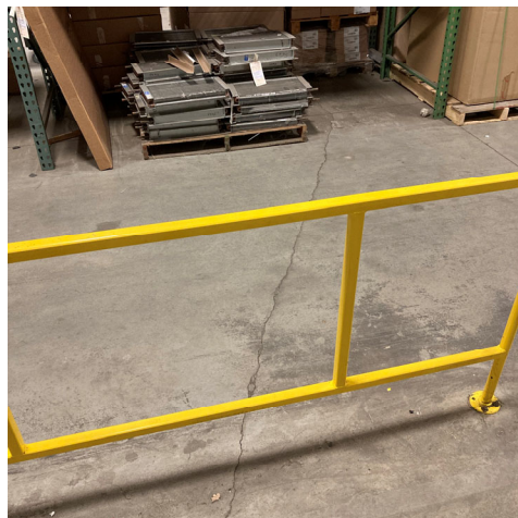
Photo 12: Minor floor cracking in manufacturing space.
