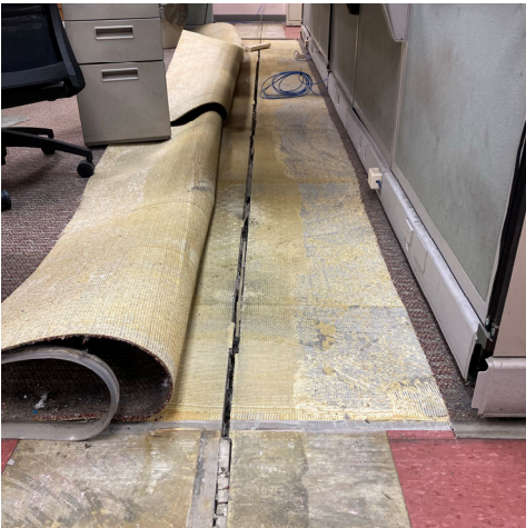
Photo 3: Expansion joint separation underneath office linoleum tile and carpeting.
