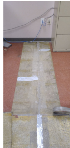
Photo 6: Expansion joint sealing in office area.
