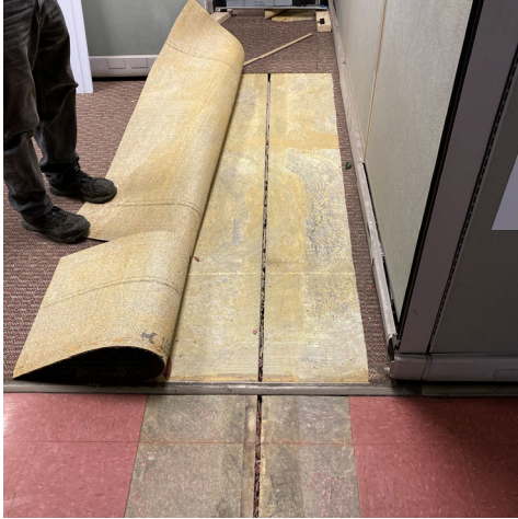
Photo 1: Expansion joint separation underneath office linoleum tile and carpeting.
