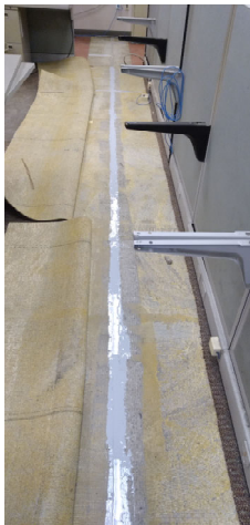
Photo 5: Expansion joint sealing in office area.
