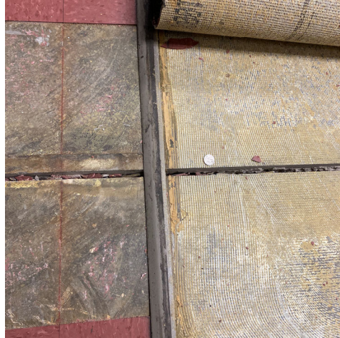
Photo 2: Expansion joint separation underneath office linoleum tile and carpeting.
