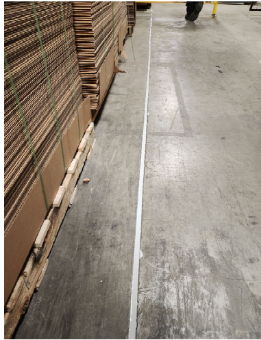
Photo 5: Polyurethane caulking in floor slab expansion joint with greater than 0.5 inches of expansion (March 2023)
