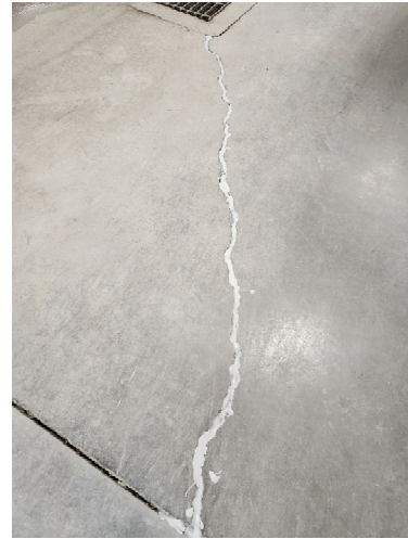
Photo 6: Polyurethane caulking in floor slab crack near paint booth (March 2023)
