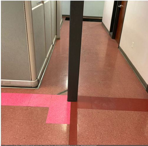
Photo 1: Linoleum tiles placed over repaired floor cracks in office hallway (March 2023)
