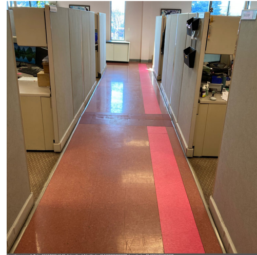
Photo 2: Linoleum tiles placed over repaired floor cracks in office hallway (March 2023)
