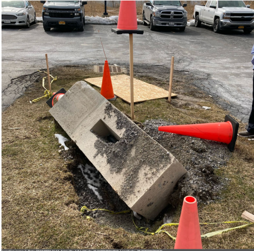
Photo 9: Parking lot light post and foundation damaged by vehicle (March 2023)
