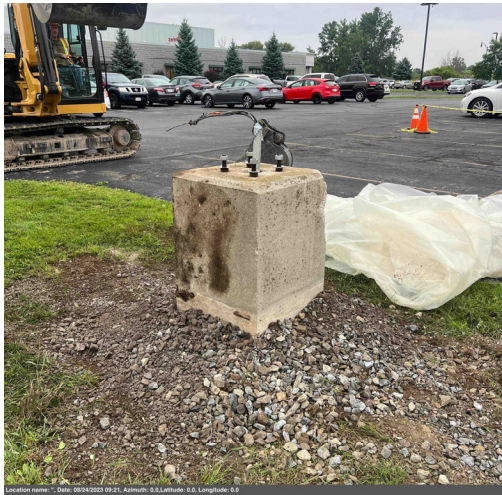
Photo 11: Light post foundation backfilled with excavated material and previously imported stone (August 2023)
