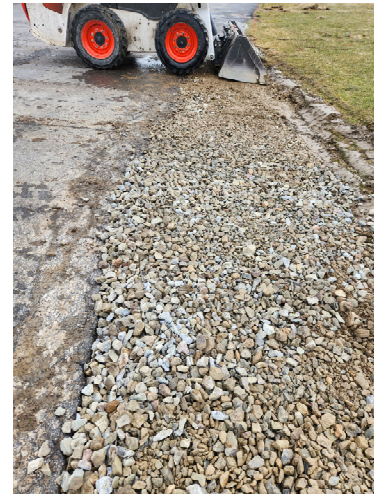
Photo 16: Parking lot/driveway rut repair/filling with previously imported stone.
