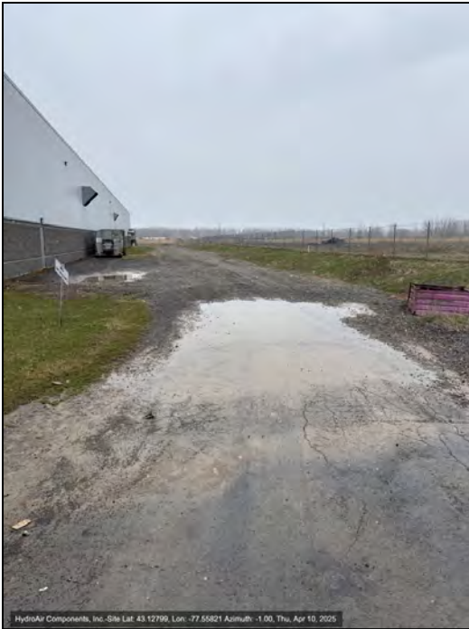
Photo 25: Apparent stormwater ponding at eastern end of northern gravel driveway.
