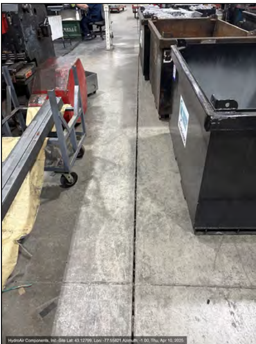
Photo 15: ~ 3/4-inch gap in manufacturing facility floor expansion joint.
