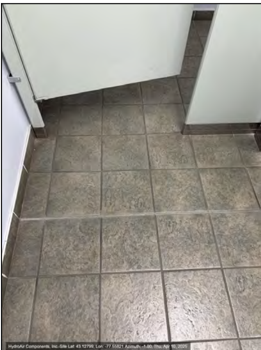
Photo 7: Previously sealed floor crack in men's office bathroom.
