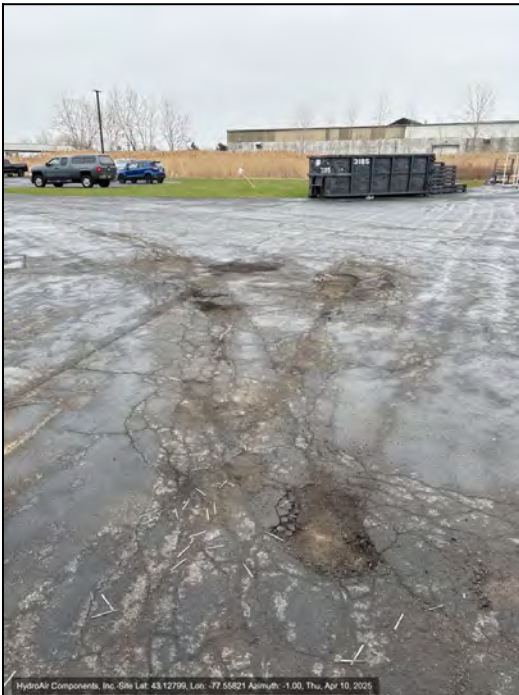
Photo 43: Deteriorating asphalt in parking lot.
