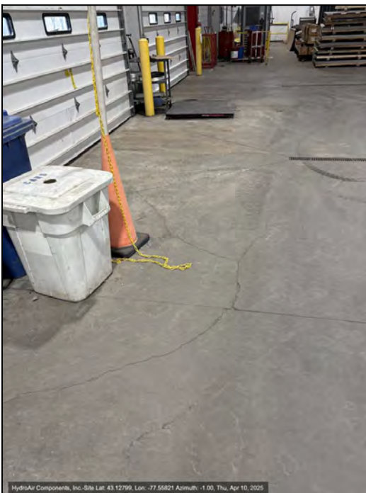
Photo 11: Small cracks in concrete floor in southwest loading area.
