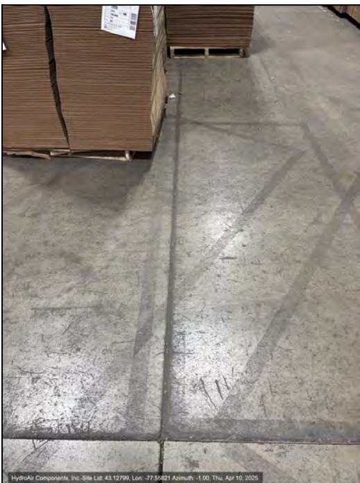
Photo 19: Previously sealed manufacturing facility floor expansion joint.
