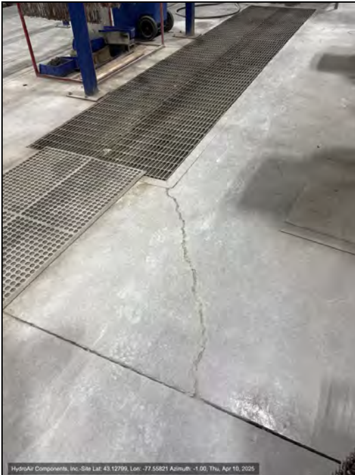
Photo 17: Previously sealed floor crack near paint booth.
