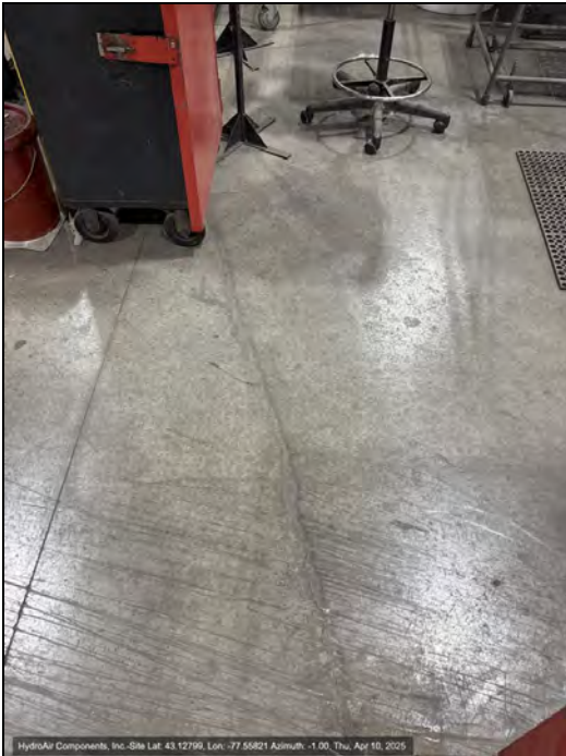
Photo 13: Previously sealed floor crack near "SW" Magnehelic gauge.
