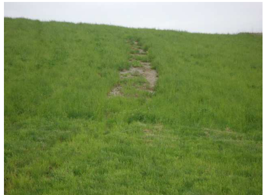
Light vegetation due to vehicle traffic between WT-7 and WT-8.
