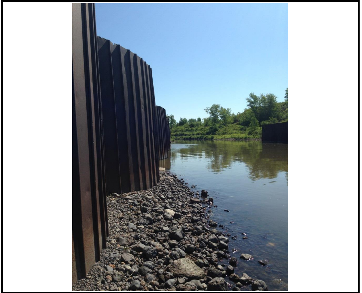
Photo No. 3: Steel coffer dam at mouth of Smokes Creek
