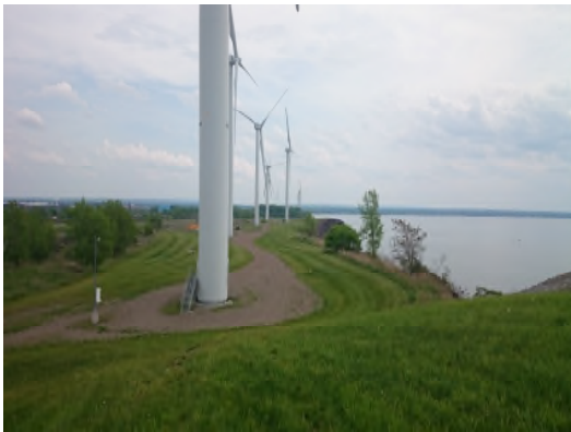
View of turbine array looking southeast.
