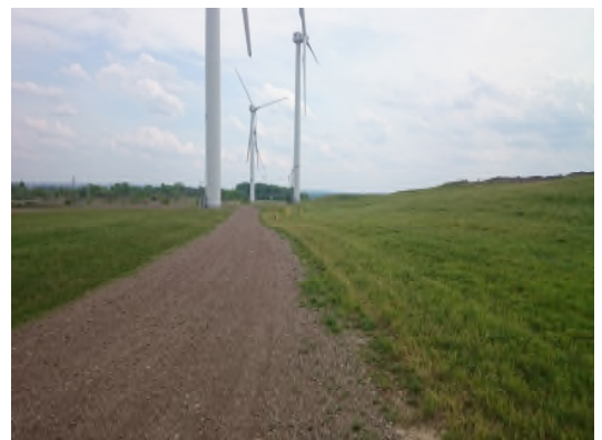
View of turbine array looking southeast.
