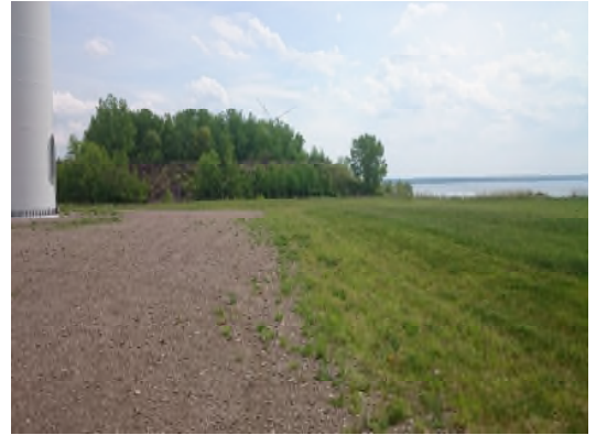
View of WT-1 looking southeast.
