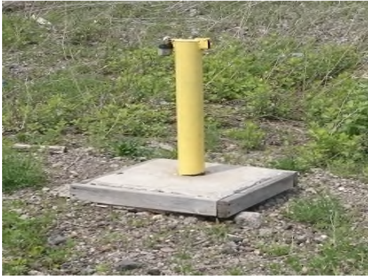
View of monitoring well WT1-05.
