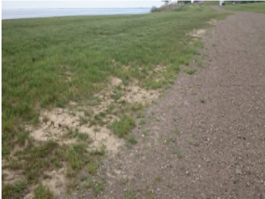
Slight tire rutting and bare vegetation patches west of WT-6.
