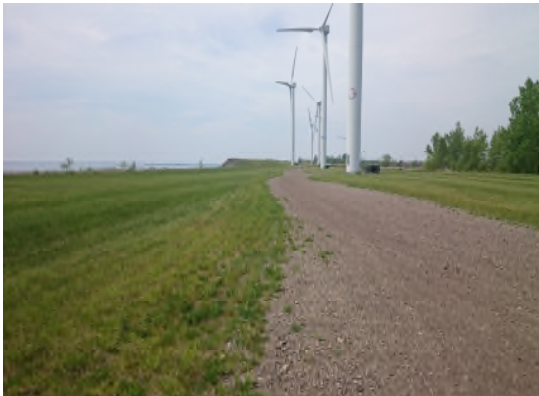
View of turbine array looking northwest.
