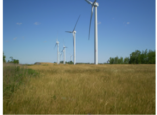
View of turbines and cover system looking northerly.
