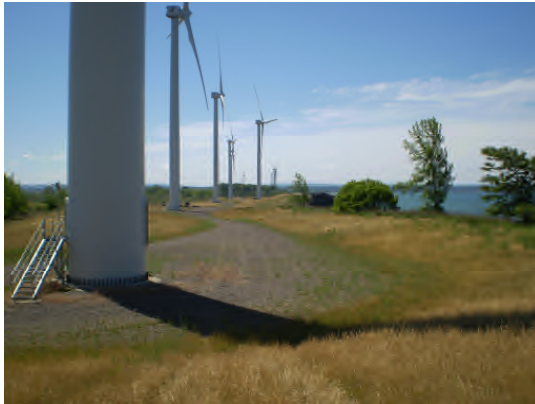
View of turbine array looking southerly.
