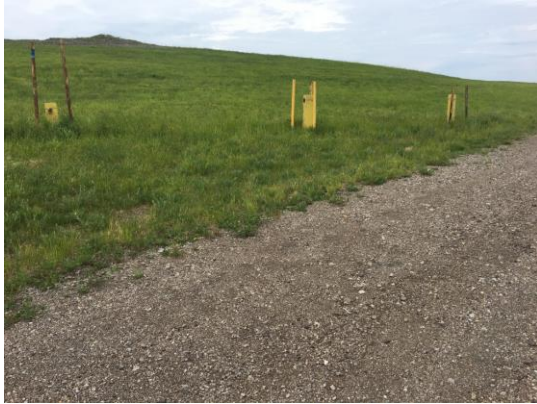
View of monitoring wells and cover system between WT#5 and WT#6.
