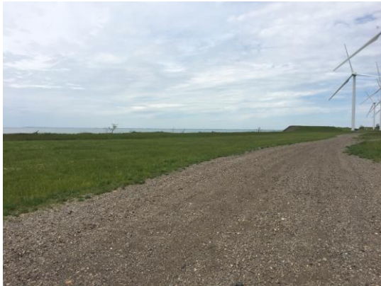
View of cover system west of access road, looking northerly from WT#1.
