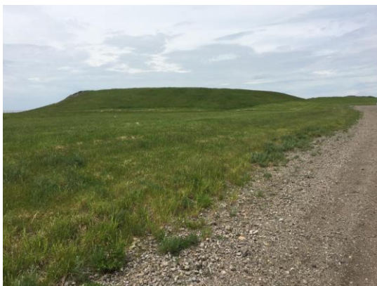
View of cover system west of access road, looking northerly from the road between WT#3 and WT#4.
