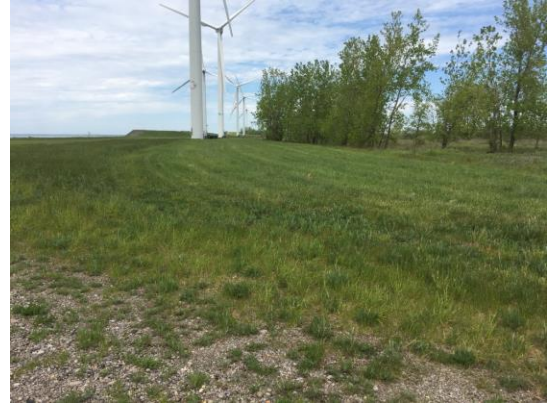
View of turbines and cover system east of access road, looking northerly from turbine WT#1.
