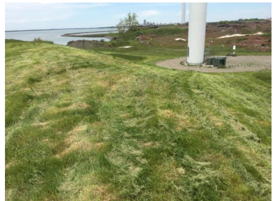
View of cover system looking north at WT#8.
