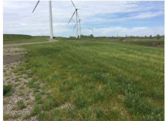
View of turbines and cover system east of access road, looking northerly from WT#3.
