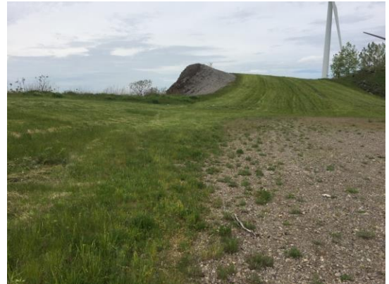
View of cover system north of WT#7, looking northerly towards WT#8.
