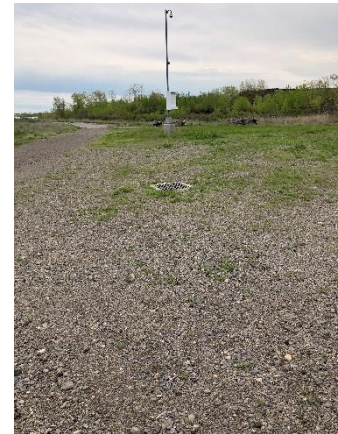
View of storm water catch basin looking south.
