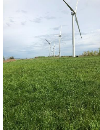
View of turbines and cover system looking northerly.
