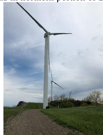
View of soil cover looking northerly towards WT 7 and WT 8.
