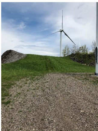
Northern portion of cover system Note: tire tracks.
