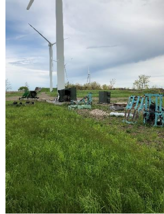
Extra transformer and electrical equipment storage area.
