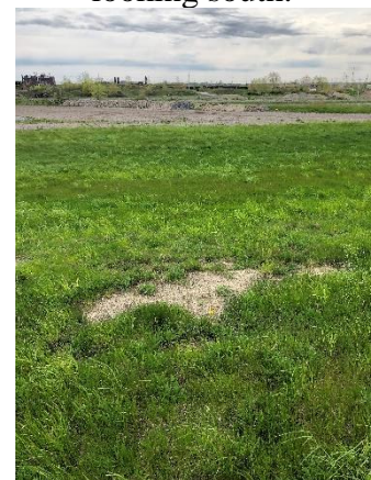
View of minor stressed vegetation on cover system.
